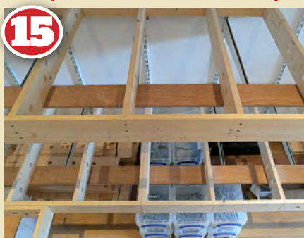
15 Two levels of baseboard are shown being supported by the metal brackets and plywood strip sections. When the lowest level is completed lighting will be fitted to the underside of the level above (probably LED strip lights) to give even illumination.
