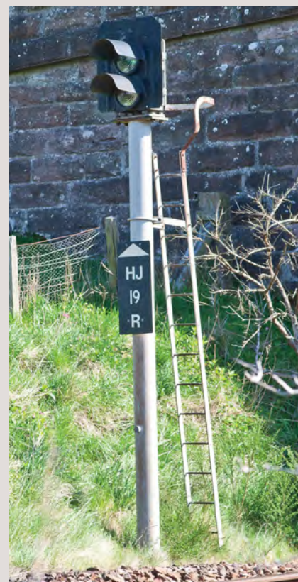
The front of the same signal displaying a green aspect (top) at the time. A distant signal would be fitted with a yellow lens in the lower position rather than red.
