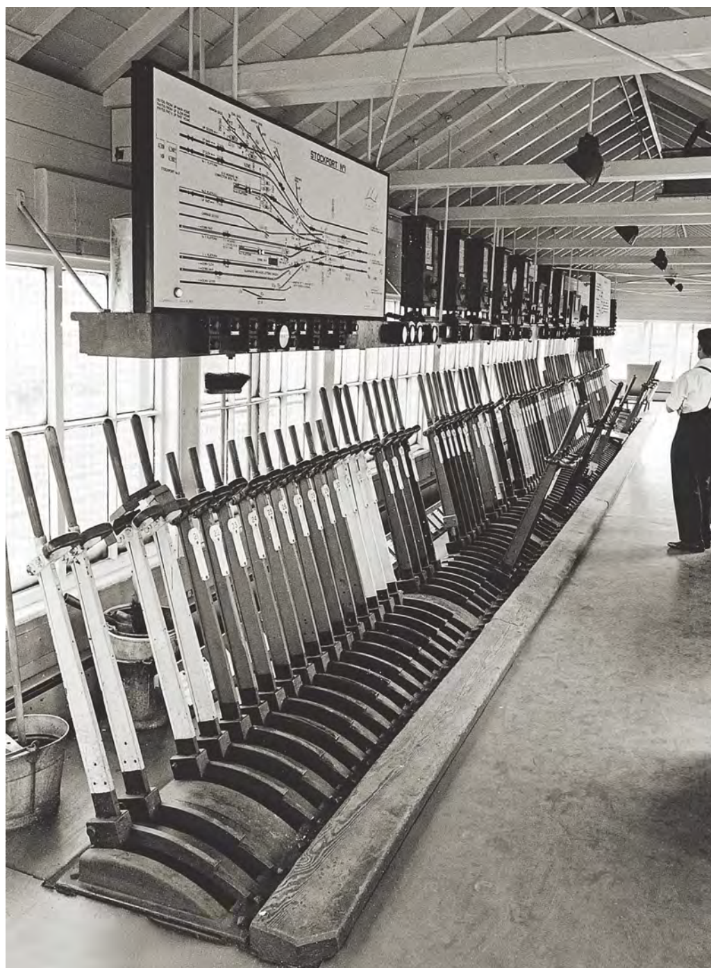
Lever frame signalboxes controlled short distances of the railway which meant a huge number of staff were required to operate them. This is the lever frame in Stockport No. 1 signalbox in 1968.
