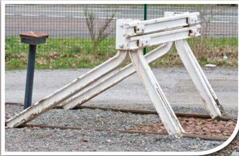
The second bufferstop at Dunkeld and Birnam is rusted and only has white paint applied to the bufferbeam face. Note how the sleepers are buried in ballast and how the frame rails taper towards the top.
