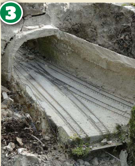
The final cutting was completed with a disc cutter and with the tunnel section now removed it exposes the junction trackwork.
