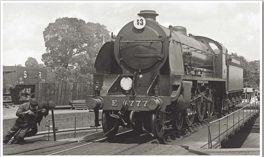
Turntables were powered by a number of different means – including locomotive crews! The crew of Maunsell 'King Arthur' 777 Sir Lamiel work hard to turn the 140ton 4-6-0 on an unidentified turntable in 1930. Gordon Stuart/Rail Archive Stephenson.
