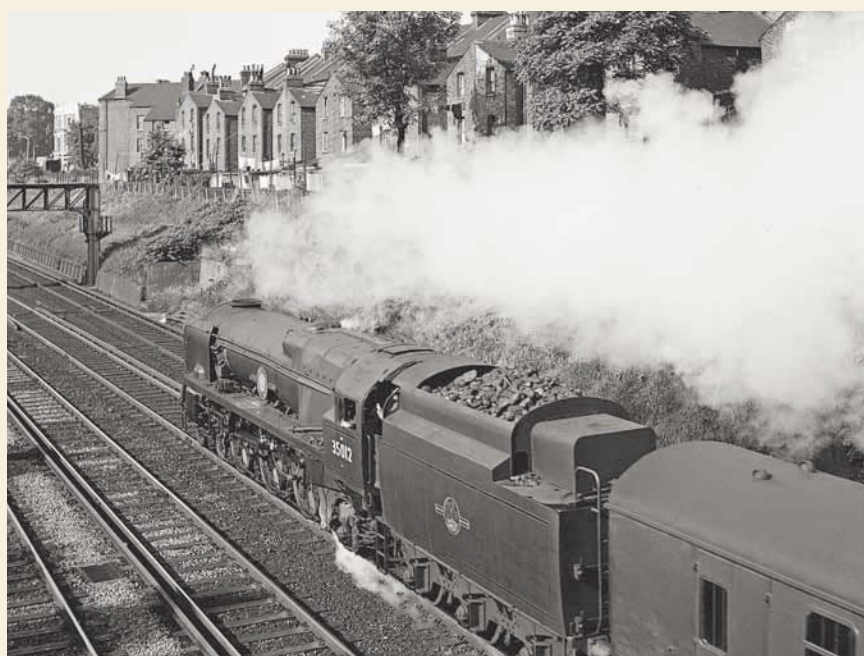
The rebuilt 'Merchant Navys' followed the styles of the BR Standard designs and were easier to maintain. Illustrating the lines of rebuilt locomotives 35012 United States Line forges south from Clapham Junction with the 8.30am Waterloo-Weymouth on July 13 1964. Brian Stephenson .
