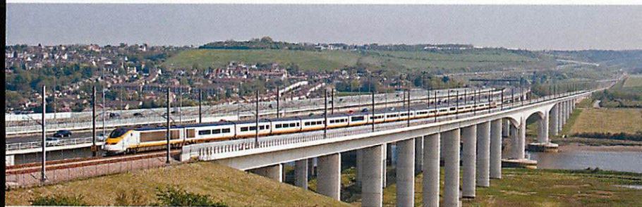
The most modern railway bridge in the UK is the Medway Viaduct on the high speed line from London St Pancras to the Channel Tunnel. A Class 373 Eurostar hurries away from the camera across the Medway bridge forming train 9036, the 15.32 St Pancras to Paris Nord on Sunday April 19 2009. Brian Stephenson .
