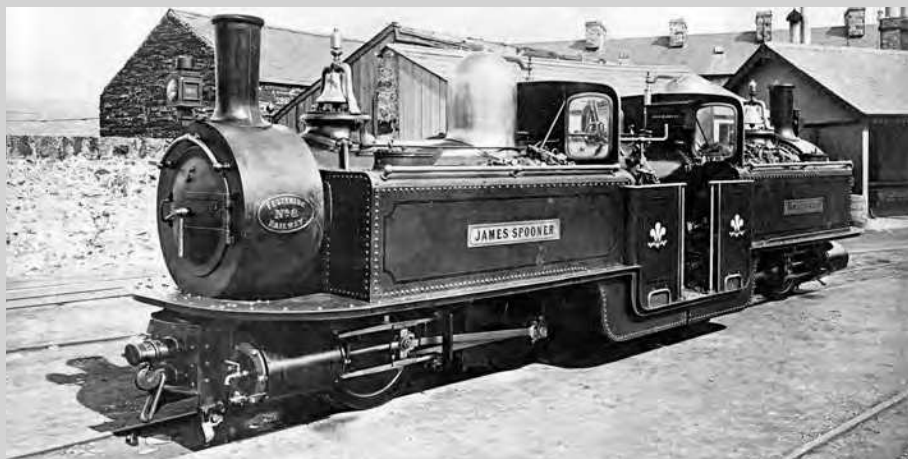
1872 built Double Fairlie 8 James Spooner was built by Avonside Engine Company in Bristol for the Ffestiniog Railway. The open cab 0-4-4-0T stands at Porthmadog station soon after completion.
