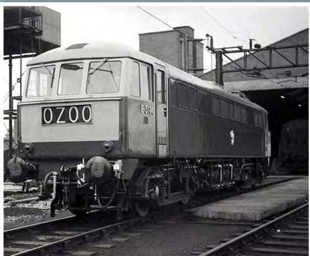
E3114 of class AL6 (class 86 under TOPS) was newly delivered from Doncaster when I photographed it at Longsight electric depot in October 1965. With this class the switch was made to the darker Rail Blue livery that would subsequently be standardised on all traction. The first five AL6s initially lacked warning panels and had red buffer beams, the remaining 95 had small yellow panels and blue buffer beams. Tim Shackleton.
