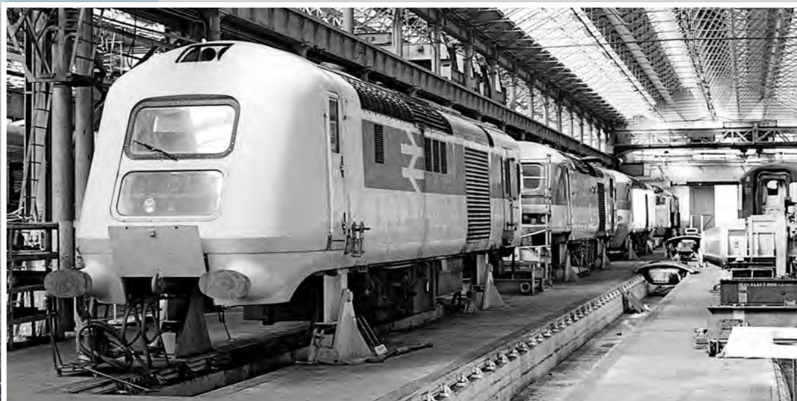
Prototype HST power car 41002, renumbered ADB975813 as part of the departmental fleet, is overhauled at Derby Works on September 6 1980 for use by the Research Centre. John Chalcraft/Railphotoprints.uk
