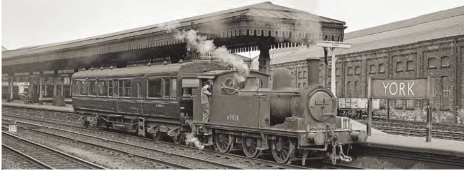
Shunting and station pilot duties were the most common use for the 'J72s'. BR built J72 0-6-0T 69016 stands at York with inspection saloon M45037M in 1960. Gordon Hepburn/Rail Archive Stephenson.
