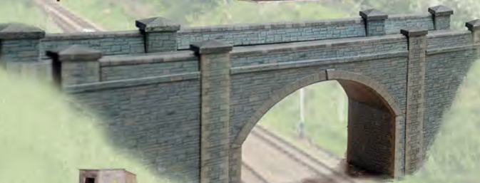
A16 Stone Bridge/Tunnel Entrance
