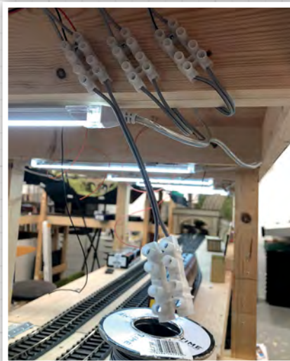
Left: Underneath the boards three new power buses have been installed. From left they are for the inner circuit, accessories and outer circuit. This is during the process of installing the inner circuit bus.
