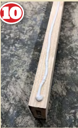
10 To ensure a strong and consistent joint between the baseboard frame and the plywood surface, No More Nails type adhesive was added to the top edge of each frame member. The baseboard surface was then lowered on top of this.
