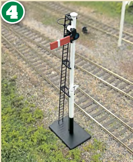
The wires can then be threaded through the baseboard followed by the mounting base on the signal. Once in position it will sit flush and level with the baseboard surface.
