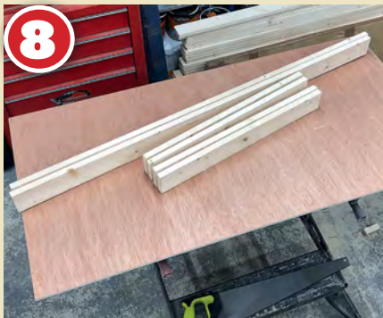
8 Using the same process the cross-member timbers were cut to size, 576mm, to fit between the outer frame members leading to a 'kit' of components to assemble.
