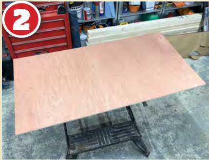
2 The top surface for all of Hornby Magazine's exhibition layouts is 9mm plywood – and it has been since our second magazine project. The first was built on 6mm plywood which, while lighter, wasn't as strong.
