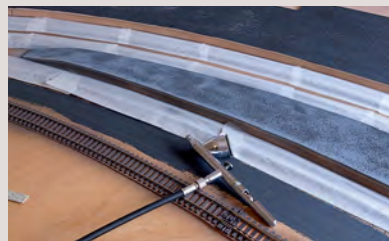
Above: Paper templates allow bases to be cut from 12mm MDF. Below: Wills stone plastic sheet was cut into strips for the platform faces while an airbrush was used to colour the final surface.
