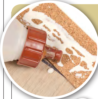
The first step is to lay track underlay (cork in this case) which has been cut to width and is being glued in place using a waterproof PVA glue.
