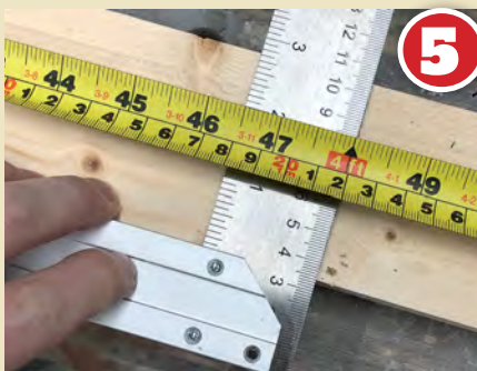
5 Having confirmed the baseboard top size, we can prepare the timber for the frame. To mark the lengths, use a tri-square and a tape measure for accurate measurements. We set out measurements for the long sides at 1,220mm.
