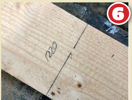
6 Mark the cut position with a pencil using the tri-square then, for future reference, note the length of the cut section on the timber. This helps to ensure the right sections are used for the right area of the board frame.
