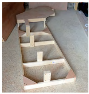
Left: Open frame baseboards were built for the viaduct scene.
