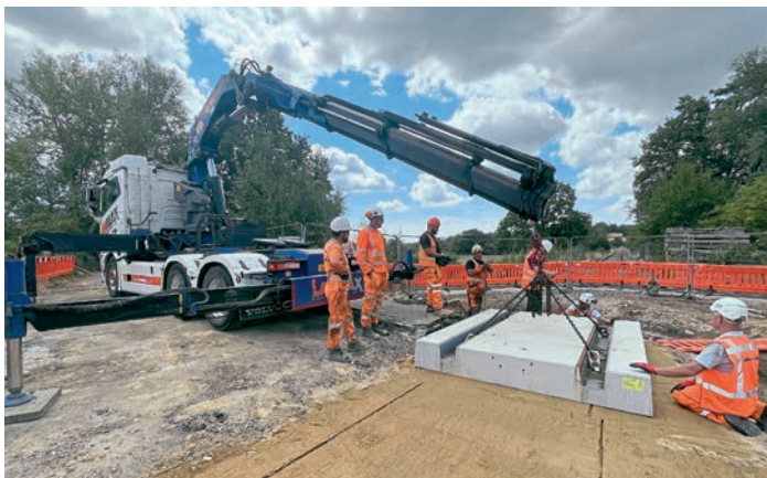
The first of the concrete slabs that will carry the railway over Northbridge Street was lowered into position on July 30, its alignment carefully monitored to match the existing RVR track. RVR
