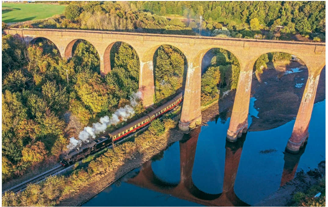
LMS 'Black Five' No. 45428 Eric Treacy emerges from beneath Larpool Viaduct on September 30, 2025. NYMR supporters will bungee jump from this structure on September 20 to raise money for the Bridge 42 appeal at Grosmont. OWEN HAYWARD
