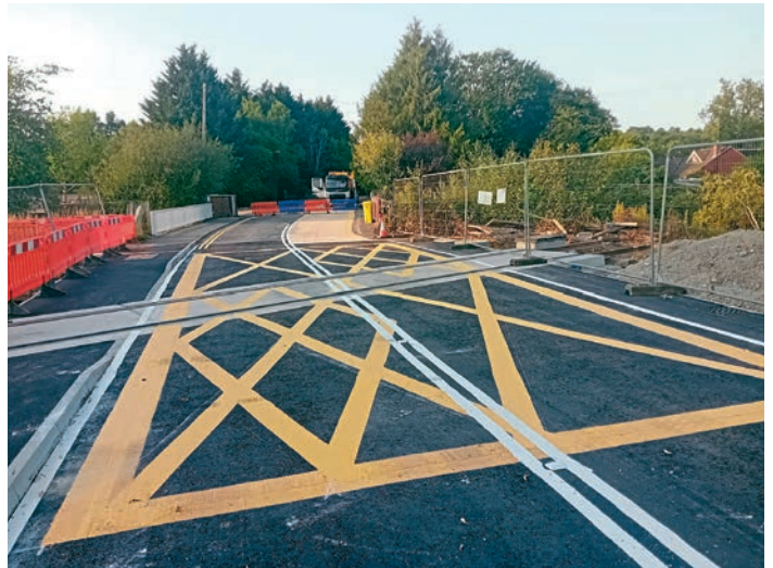
By August 14, the Northbridge Street level crossing was completed to the point of allowing the road to reopen. RVR
