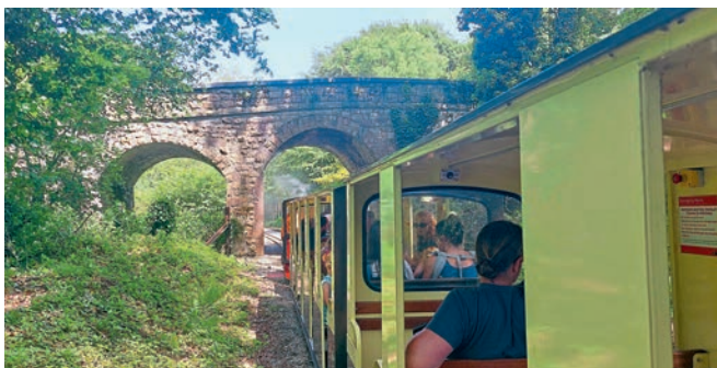
View from the Lappa Valley's 15in on the way back to Benny Halt showing Metha Bridge and the wartime brickwork from when the bridge was widened during the Second World War.
