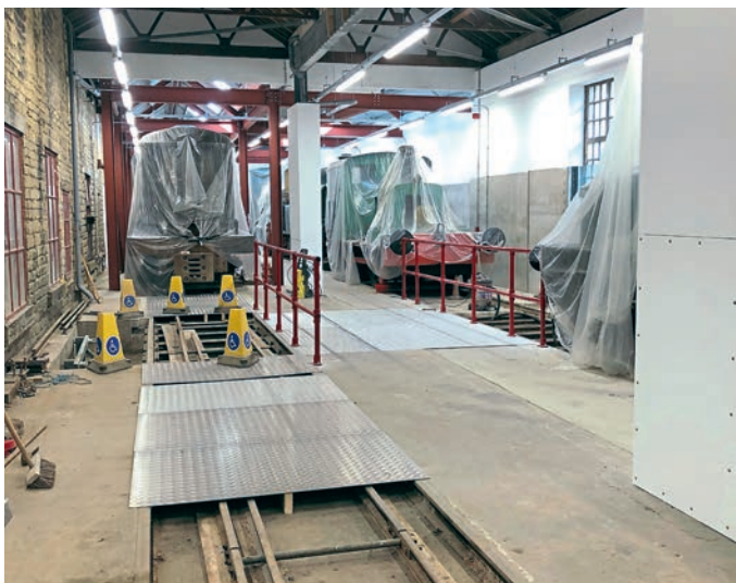
The Railway Gallery taking shape prior to reopening.
