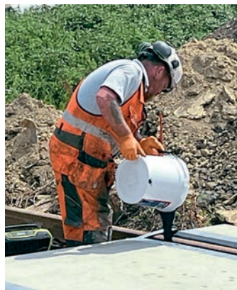
Corkelast, a specially-designed bonding material, was poured into the grooves that will both hold the rails in place and reduce noise. RVR
