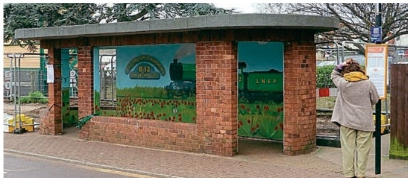
The bus shelter prior to demolition, with the transport hub work site alongside the North Norfolk Railway tracks. HUGH VENABLES/CREATIVE COMMONS
