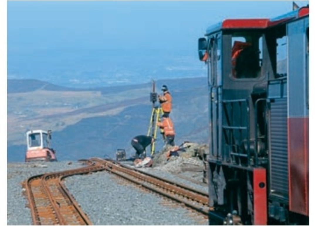
Installing the new points indicator at Clogwyn, looking towards Llanberis. PHIL MARSH
