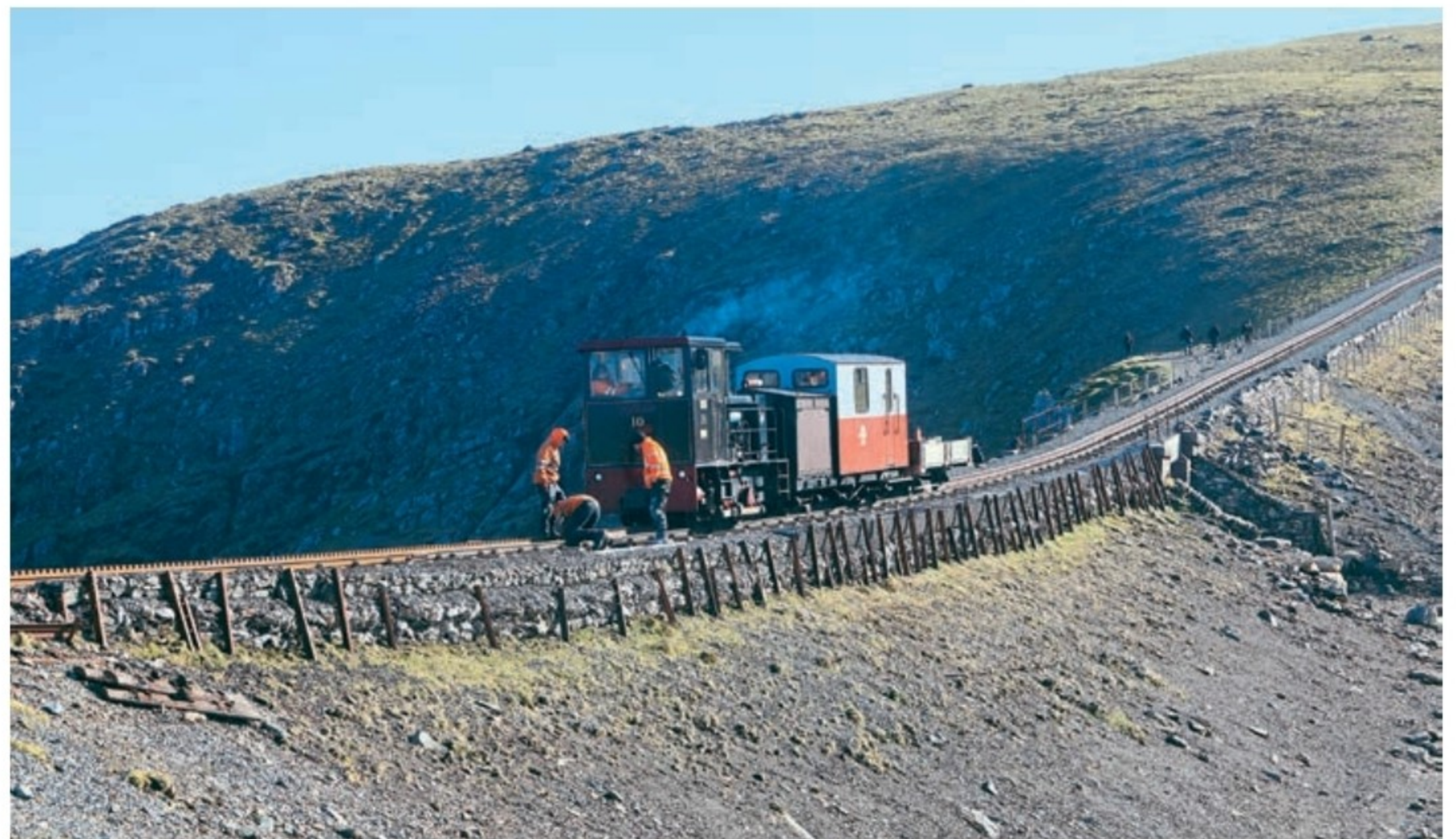
Gauge checking by the first train to run on the new track on the ridge above Clogwyn. PHIL MARSH
