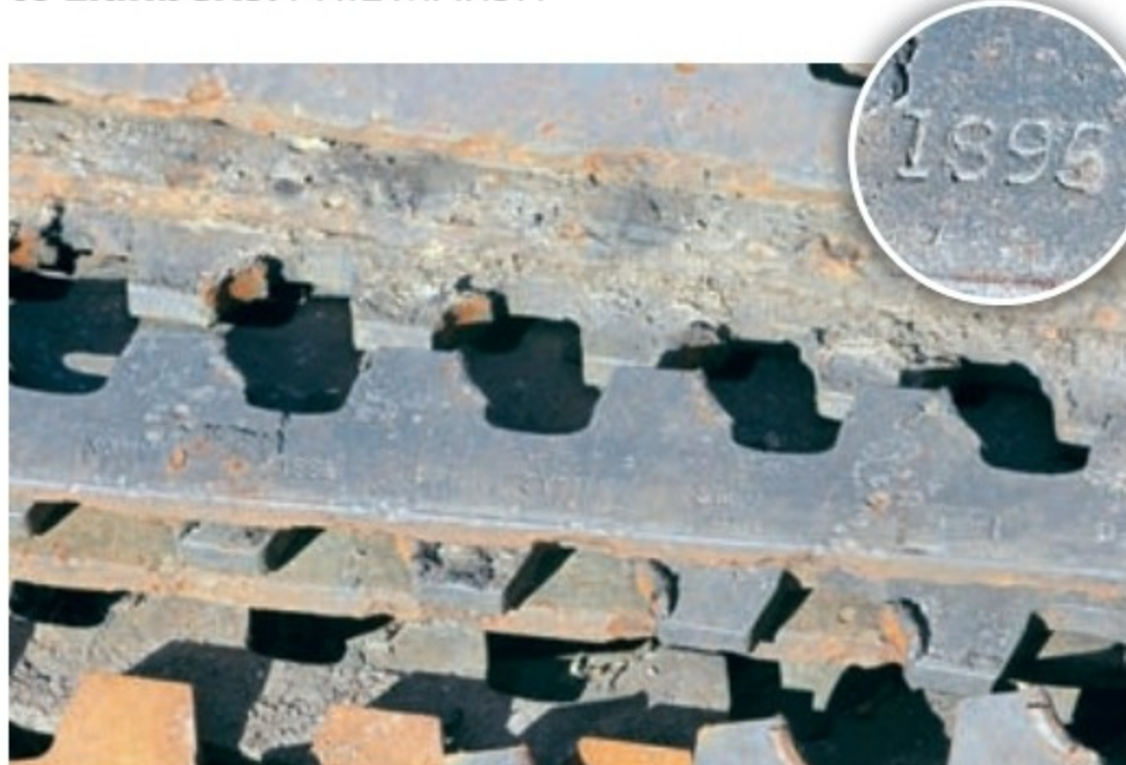
Original section of 1895 rack replaced at Clogwyn. PHIL MARSH
