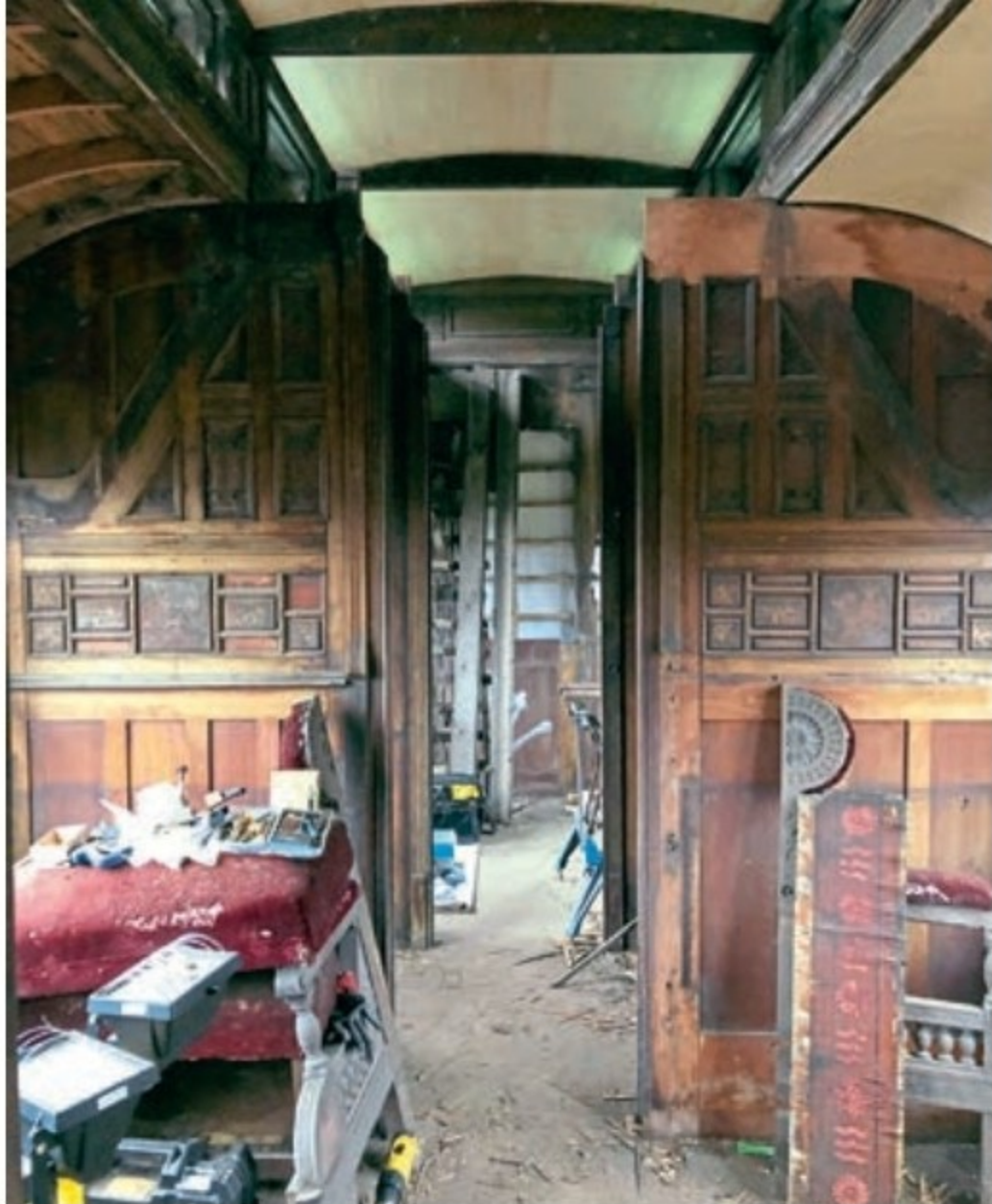
Inside the carriage, the original panelling has been put back in place. SALLY CLIFFORD
