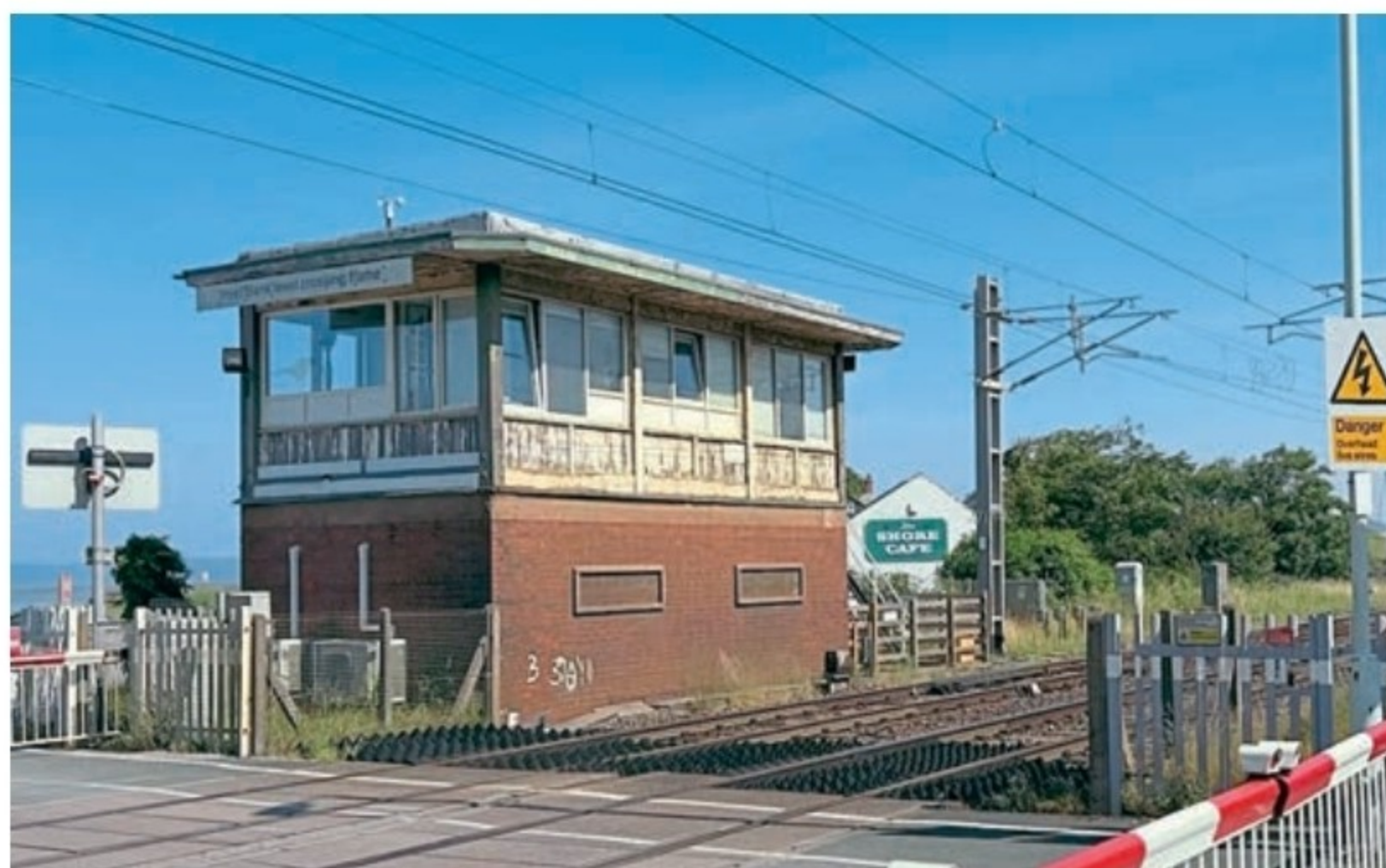
The signalbox at Hest Bank on the West Coast Main Line. NR
