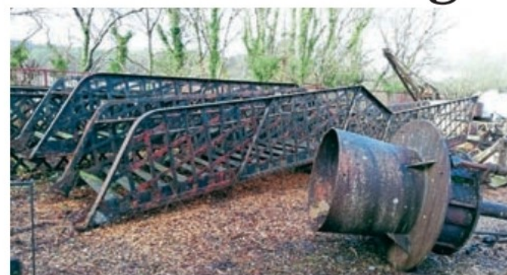
The Taff Vale Railway footbridge in store at Nantgarw. Amgueddfa Cymru is seeking expressions of interest to find it a new home. AMGUEDDFA CYMRU
