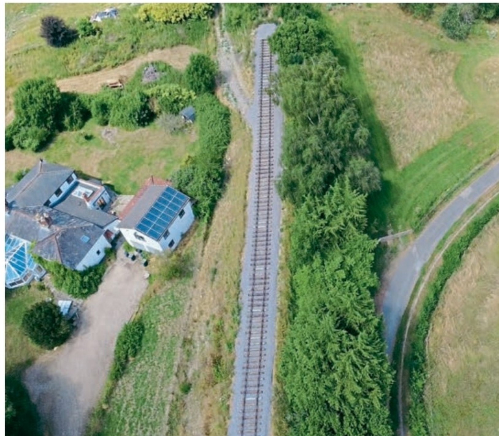
An aerial view of the new track leading from Shillingstone station. SDR
