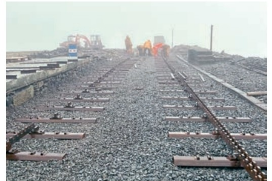
Clogwyn Loop being lifted last October prior to being relaid. SMR
