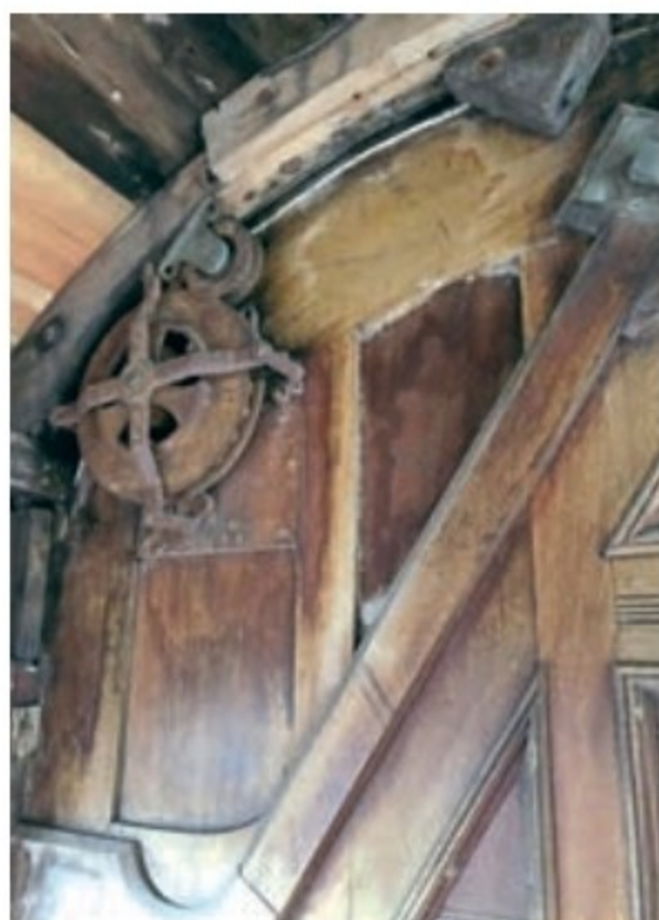
The original spring-loaded mechanism to lower the bed into place. SALLY CLIFFORD
