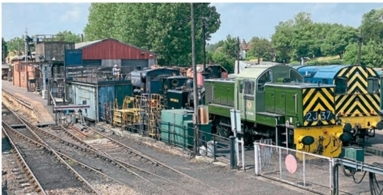
Rolvenden, the engineering hub of the KESR, has not seen substantial investment for several decades. A new fundraising club has been set up to raise £50,000 over five years, with Rapido Trains UK pledging £10,000 per year in match-funding. JULIE WILKINSON/KESR
