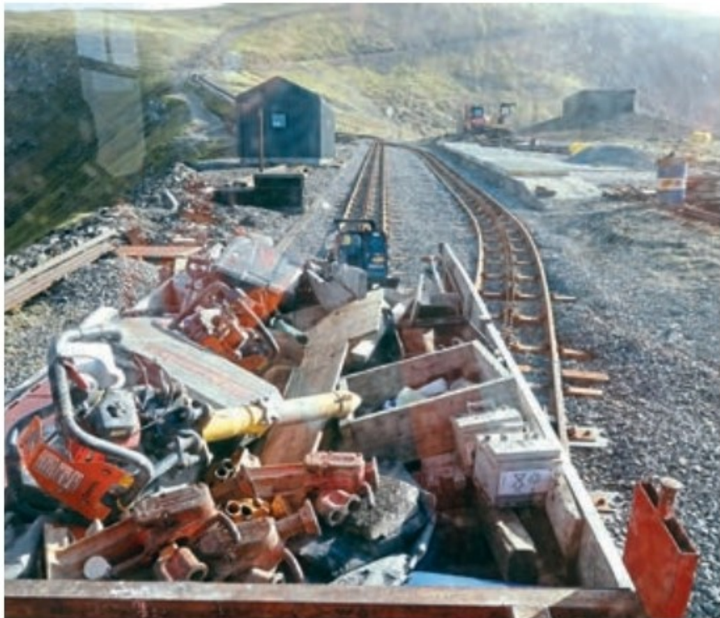
With all equipment loaded, the works train departs from Clogwyn Loop at the end of the March 3 shift. PHIL MARSH
