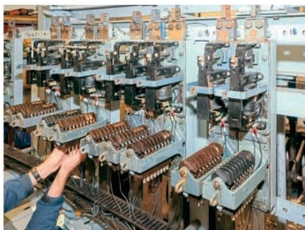
New cranks being installed as the new lever frame starts to go in.
