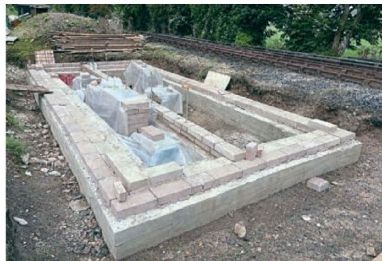
The concrete for the foundations for the new Junction Box, now set. TOBY WATKINS
