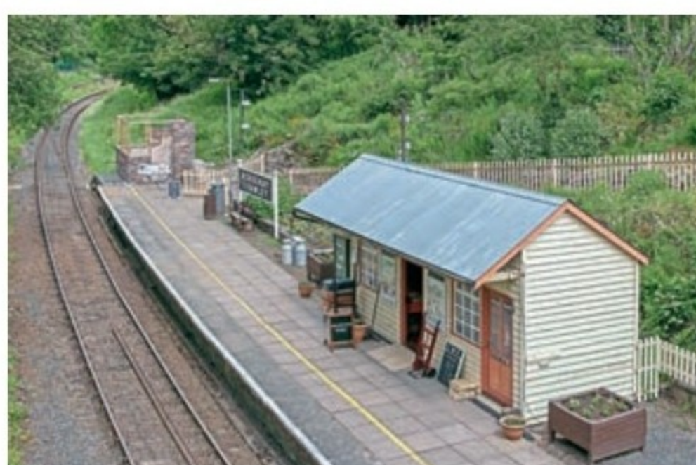
Horsehay & Dawley station where work progresses on the new signalbox.
