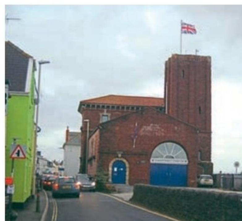
The Brunel Pumping House alongside the Exeter to Plymouth main line in Starcross.
