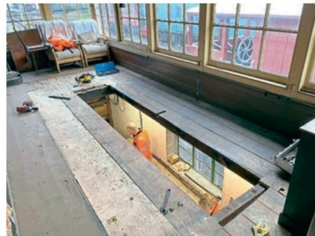
With the old frame gone, some floorboards were cut away, ready to accommodate replacements.
