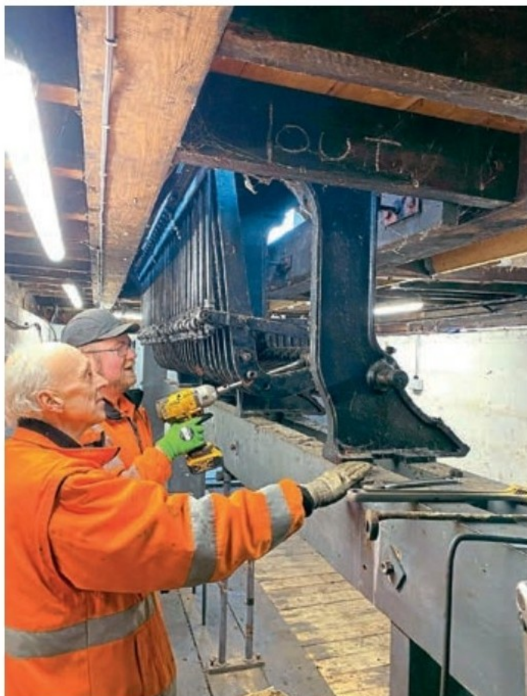
Linkages being disconnected from levers below the frame on January 10.
