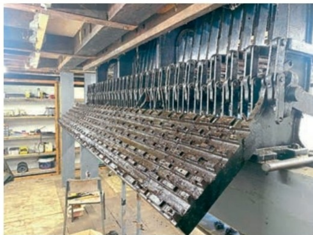
A baron interlocking panel after linkages were all removed.
