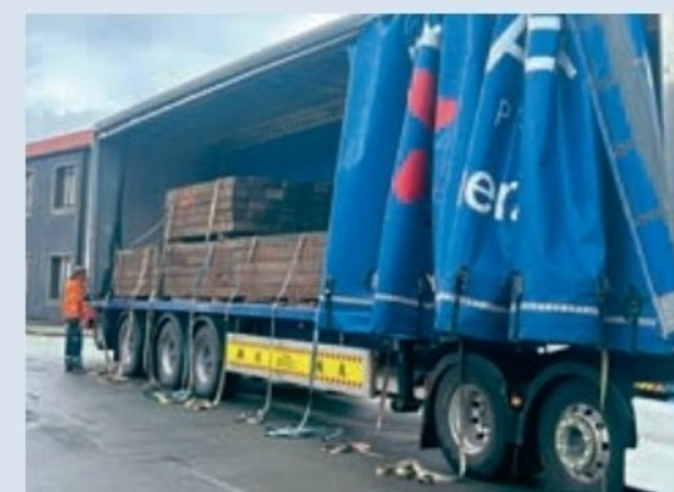
The first consignment of hardwood sleepers for the 'Red Dragon' extension is delivered. BLRT
