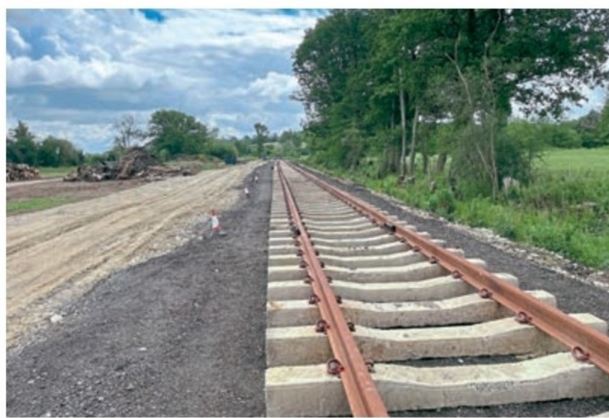
The first stretch of track on the KESR extension was completed by June 5, with more to follow imminently. MIKE HART/RVR
