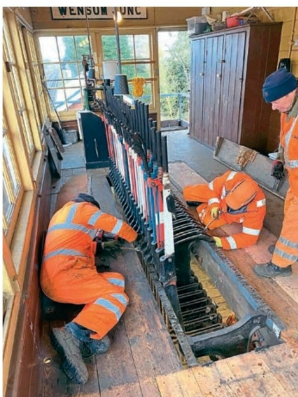
As lever frames tend to span two floors, this often required passing components from above down to those below. By January 10, dismantling the old frame was well underway.
