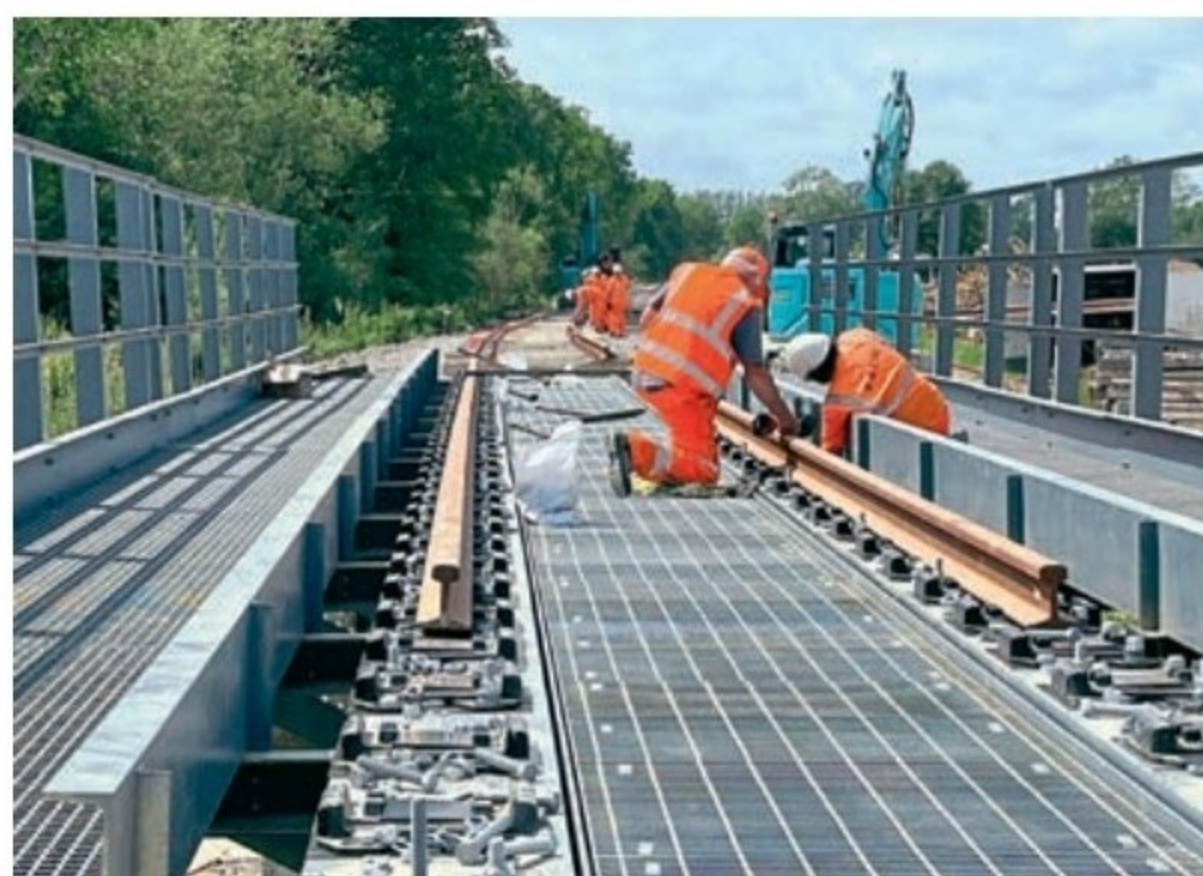
Rails being fitted to the recently installed Bridge 24 decking. MIKE HART/RVR
