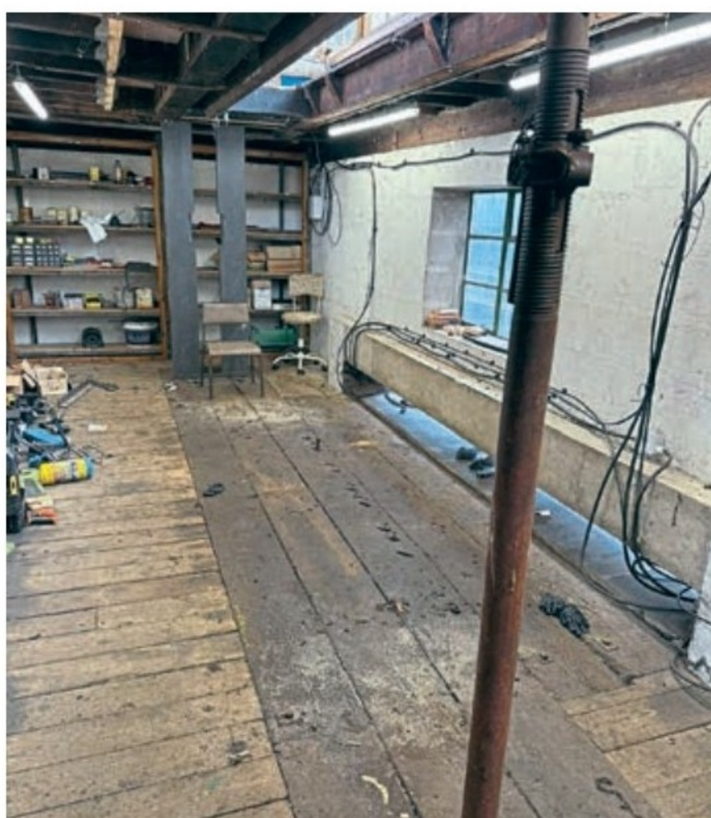
With beams removed as part of the dismantling process; steel props were required to temporarily support the upper floor.
