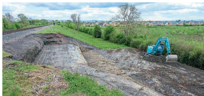
Repairs to the landslip underway on April 20. IAN CROWDER
