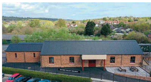
The newly completed Robertsbridge Junction station building opened on April 17.
