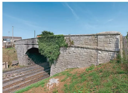
Northbrook Road overbridge on the Swanage Railway. EH
