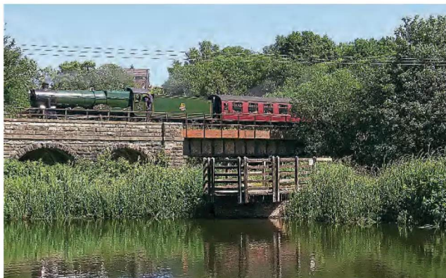
Picturesque Higher Woodhill Viaduct on the East Lancashire Railway needs £1.28 million spent on repairs. ELR
