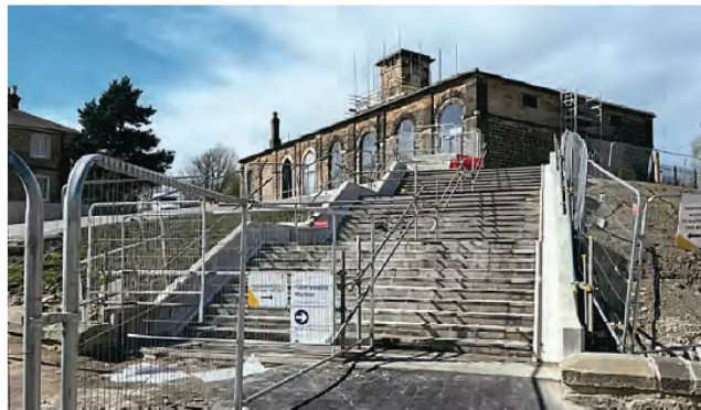
The entrance to Darlington Hopetown railway heritage centre's main building is almost complete. DBC
