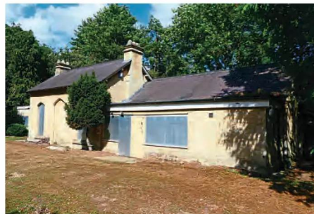
Wansford Road station before dismantling. ROBIN JONES
