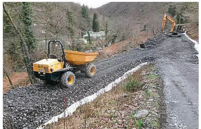
The embankment to support the Corris Railway's extension is gradually being built thanks to the delivery of spoil created through the construction of a new road bridge at Machynlleth. CR
