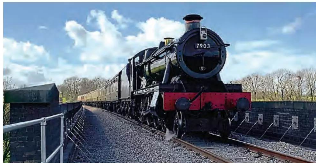
Regular trains returned to Stanway Viaduct on March 29 following the completion of the first phase of repairs to the structure built for the GWR in 1903/4. WR Foremarke Hall is pictured heading the second train over the viaduct following its reopening. G/WR
