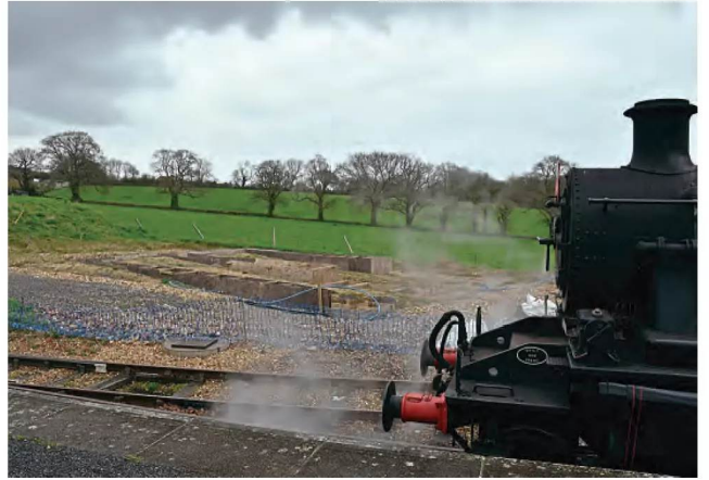
At Wootton, a small goods shed is in the process of being built that will convey the way freight was handled by the railway. On March 27, the groundwork was well and truly underway, though recent heavy rainfall had temporarily halted progress.
