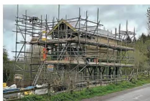
The Grade II-listed Hertford East signalbox taking shape at Constable Burton on the Wensleydale Railway. NICK KEEGAN/WR
