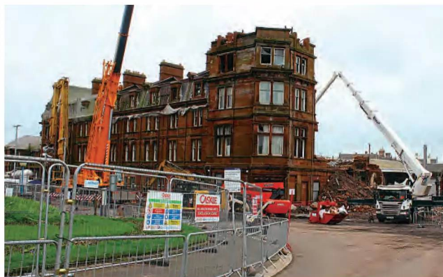
Work starts to demolish the north range of the station hotel, with the fire-damaged tower to the right. HUGH DOUGHERTY
