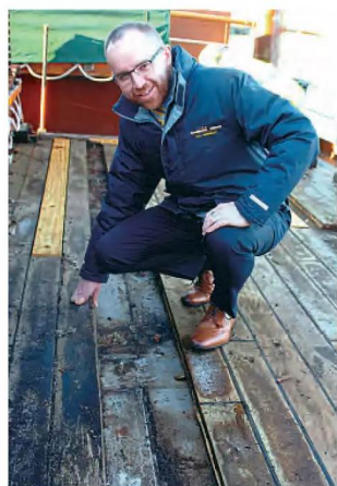
Waverley general manager Paul Semple has plenty to smile about as he inspects decking repairs on board the paddle steamer. HUGH DOUGHERTY
