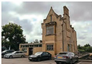
Cirencester Town station building is to receive vital repairs. CDC
