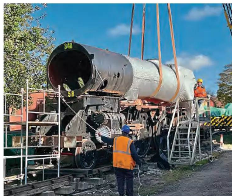
On November 7, the boiler for No. 34058 Sir Fredrick Pile was lifted off its frames at Sellindge. SIMON TROY/SLL
