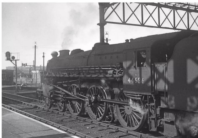
'Black Five' No. 44686 is about to depart from Liverpool Exchange. You can see, clearly, the Caprotti valve gear and the changes to the locomotive's appearance brought about by this alteration. The strange dome-shaped object just to the right of the smokebox is the top of a water column – a common feature at the end of many a station platform in the steam era. NEVILLE WELLING
