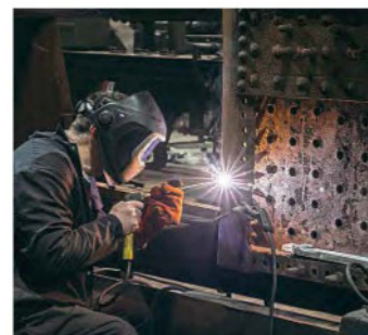
New platework being welded in the outer firebox of the boiler. The lower part of the throatplate is being replaced. Once that has been riveted in place, the firebox side sheets can be replaced. GWS
