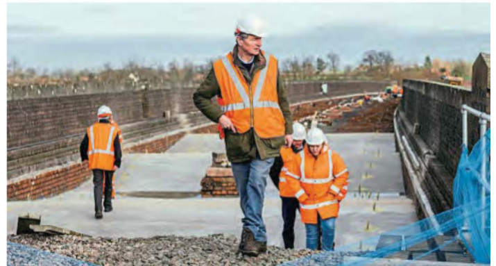
Sir Timothy Laurence inspecting Stanway Viaduct, with the newly installed grout visible along the faulty joint between the common red and the engineering blue bricks. JACK BOSKETT/G/WR
