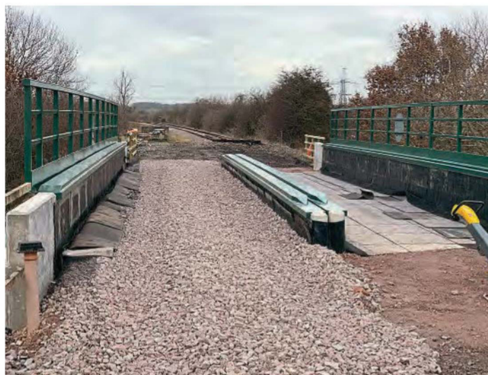
The A60 bridge, part of the GCR Reunification project. On the left, new ballast will carry trains between the two sections of the GCR, and on the right, relaid track will take trains to the national network. GCR
