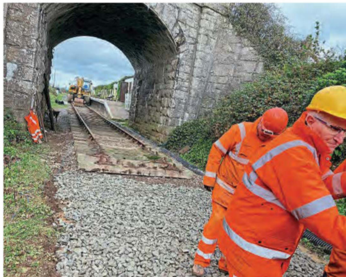
Work underway to extend the Helston Railway's running line south from its current terminus at Truthall Halt. HR
