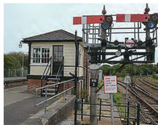
The soon-to-be-redundant Grade II-listed signalbox at Par station. N CHADWICK/CREATIVE COMMONS
