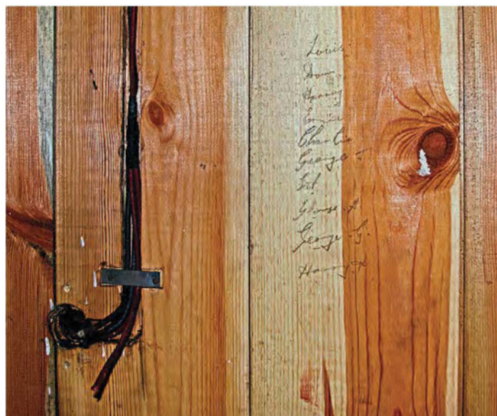
The pencilled names of the men who built No. 24617 and original wiring exposed during the start of restoration in September 2022.
