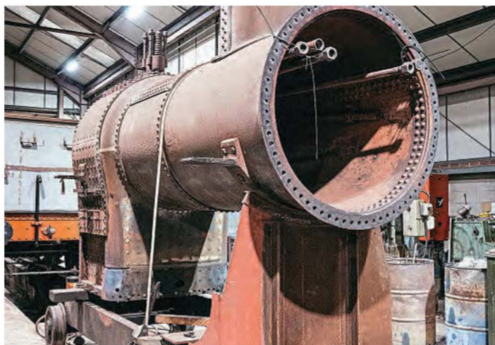
The boiler of No. 1363 on a trolley while the firebox repairs are being made. GWS
