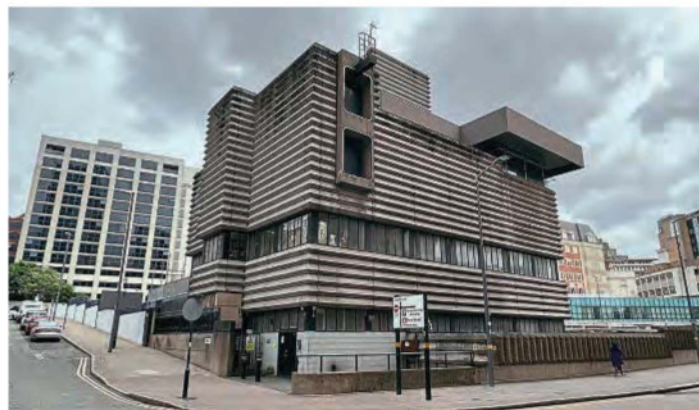
Birmingham New Street's Grade II-listed Power Signal Box. NR
