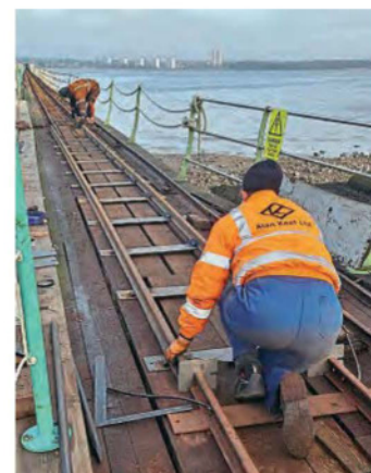
The aligning of track and points on the pier railway on December 6. ALAN TITHERIDGE/HRHA
