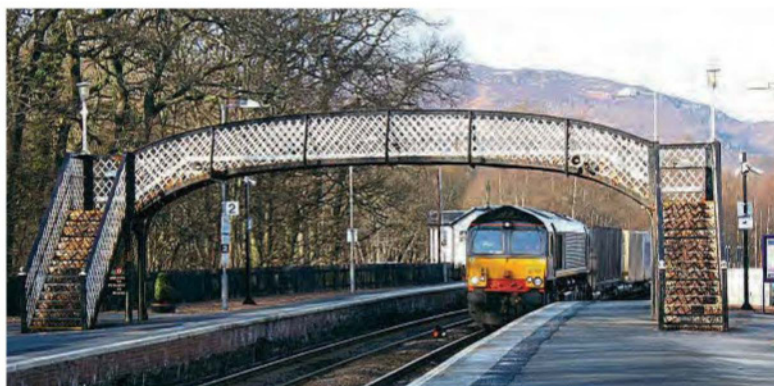
Left: Direct Rail Services Class 66 No.66420 passes beneath Pitlochry station's Victorian footbridge with a container train from Inverness on February 19, 2010. HUGH DOUGHERTY
