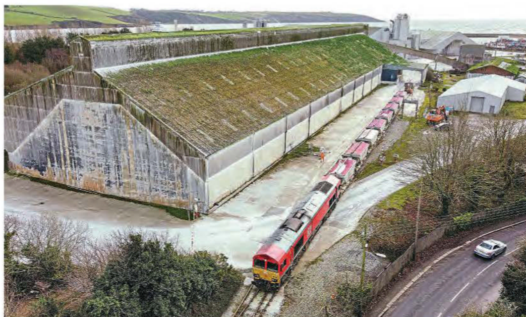
The rake of nine redundant CDA wagons delivered to Par Docks on December 6. JOHN HIRD/BWR
