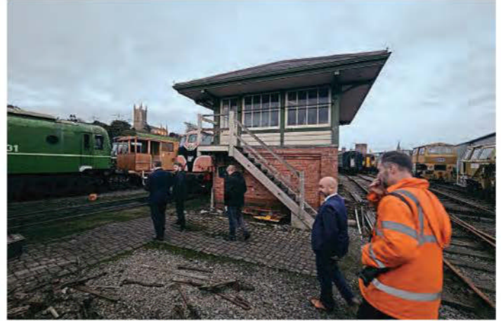
The visiting politicians inspect the damage to the yard for themselves after the flood water receded. D&CDR
