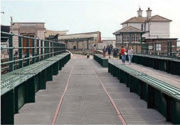
Folkestone Harbour station renovation with the restored viaduct swing bridge walkway surface.
