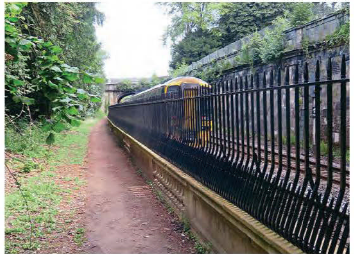
Sydney Gardens balustrade wall safety railings looking north towards Beckford Road bridge.
