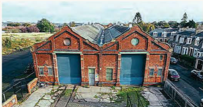
Maryfield Depot from above, showing its surviving tram tracks. Its Victorian bricks are in need of refurbishment. DMOT
