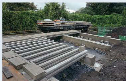
Left: A new platform being constructed at Sittingbourne Viaduct station will enable step-free access to the Sittingbourne & Kemsley Light Railway's services for the first time. SKLR
