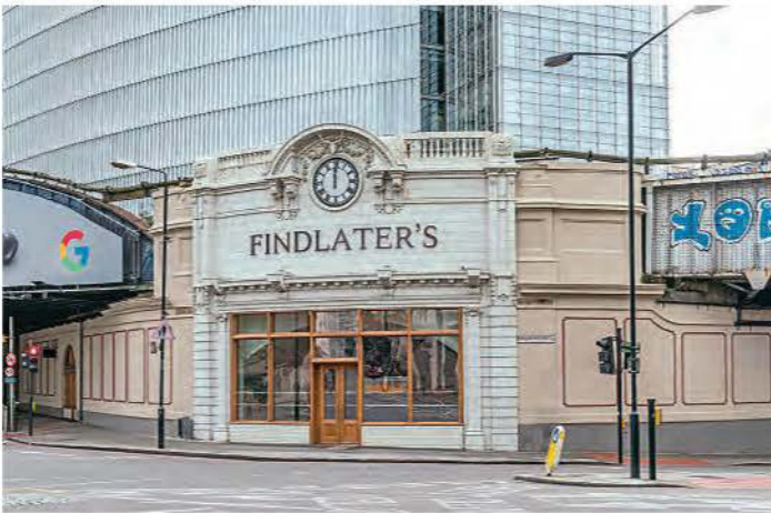
Work began in January 2022 to restore the historic group of four arches at London Bridge Island. The most prominent, the 'corner' facing London Bridge, took the name of the company once occupying the arch, the Scottish wine merchant Findlater's.
