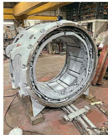
The outer casing of the Crompton Parkinson main generator has been refurbished at the contractor's workshops while the armature has been taken out for machining and rebanding. TEAM 45
