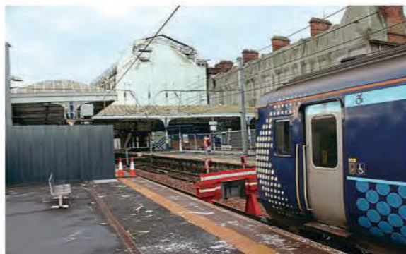
A Class 156 sits at the limit of working at Ayr Station on December 6 with a barrier across the tracks towards Girvan and Stranraer and a temporary buffer stop. The fire-ravaged hotel, parts still covered in scaffolding and protective sheeting, tower above the station.
