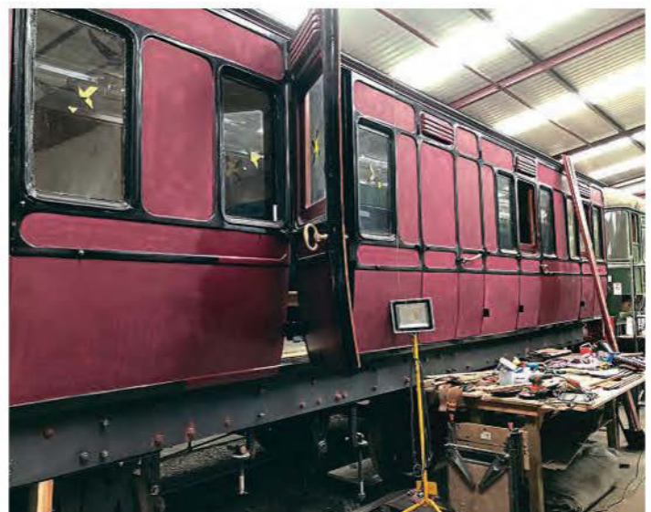
Work is underway to restore the Midland Railway carriage used in the 1970 film The Railway Children .
