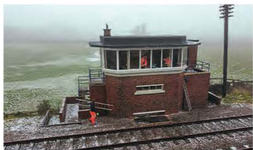
Hotchley Hill signalbox with repaired concrete on December 3. TOM INGALL
