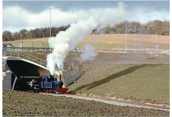
Barclay 0-6-0T No. 1641 of 1919 Doll emerges from beneath the new Chamberlains Bridge on the Leighton Buzzard Railway.
