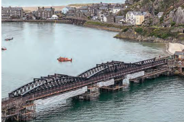
Restored Barmouth Viaduct is open again for trains and walkers. NETWORK RAIL
