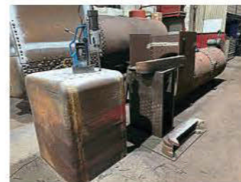
Drilling crown bolt holes in GER 0-4-0T No. 229's new firebox. THE FLOUR MILL
