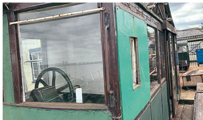
Hythe Pier carriage No. 2 (1327) out of service, awaiting inspection and restoration. ALLAN FAIRHEAD/HRHA
