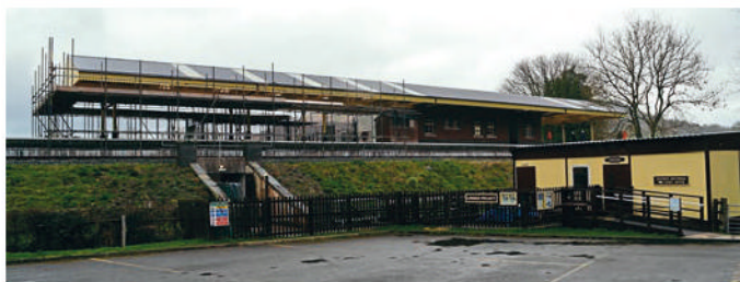
Above: Scaffolding has started to be dismantled at the LR's new Corwen terminus following cladding out of the new canopy roof. Opening is set to take place on June 1. OWEN HAYWARD
