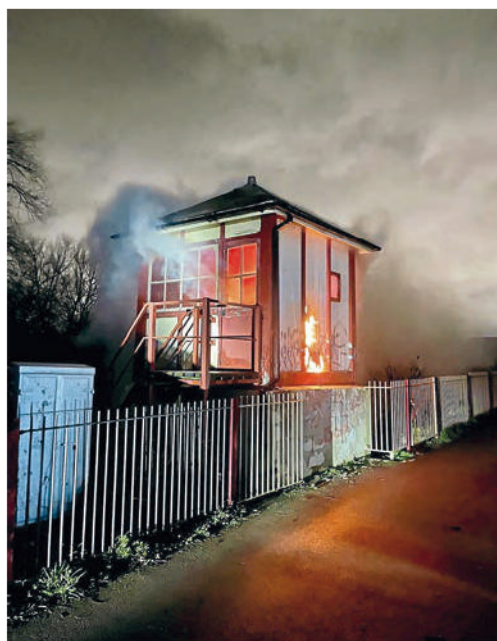
The fire in Orton Mere signalbox, which is believed to be an arson attack, at about 12.30am on March 13.
