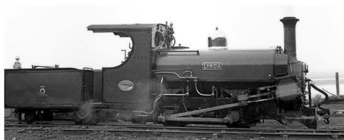
Above: pictured in August 1964 following further modifications to fit the gauge of Garnedd Tunnel and clearly showing the absence of a leading pony wheel, something which would not be added until 1970. FF&WHR
