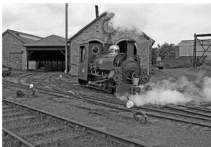
Above: pictured in August 1964 following further modifications to fit the gauge of Garnedd Tunnel and clearly showing the absence of a leading pony wheel, something which would not be added until 1970. FF&WHR
