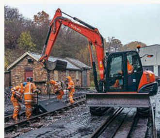
Trackwork in progress as part of the winter maintenance schedule. NYMR
