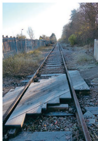
The Fletton Loop at Peterborough, pictured at one of two foot crossings in Belsize Avenue, is currently closed because of the need to replace track components over a section.
