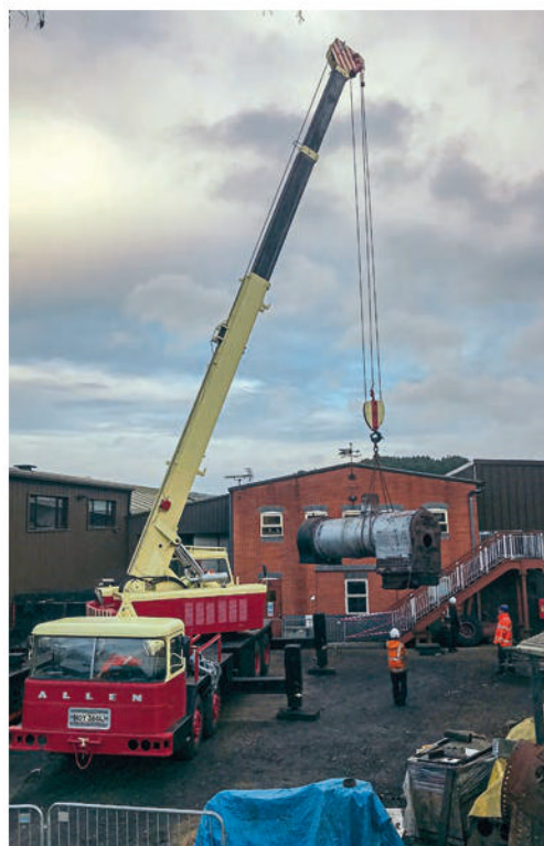
The successful lift of the boiler of Ring Haw at Weybourne. STEVE ALLEN/M&GNJRS
