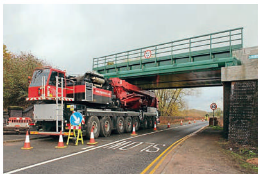
The completed bridge, with the crash protection beam in front of the main decks, has slightly improved headroom over the road compared to the original. KARL GILLOTT/FRIENDS OF THE GREAT CENTRAL MAIN LINE
