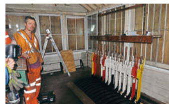
Above: The lever frame back in place inside the signalbox. MNR
