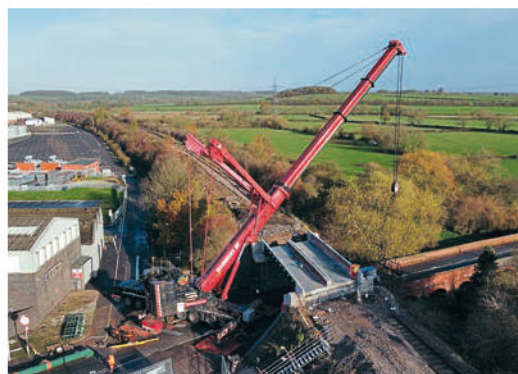
View from above: The two new bridge decks in place above the A60 on the morning of Sunday, November 20. FRIENDS OF THE GREAT CENTRAL MAIN LINE
