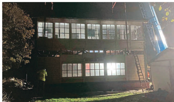
Just 20 hours after being split in two at Reedham, the signalbox comes back together at Holt. STEVEN ASHLING/NNR
