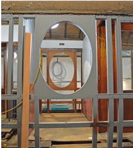
The iconic Thompson ovular window is positioned where the toilet compartments once resided, and which are now due for reinstatement.
