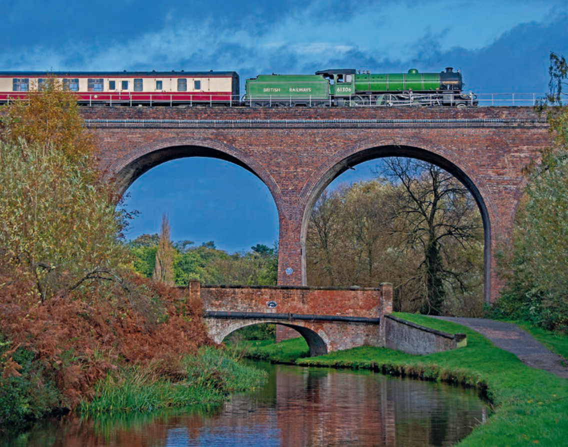
B1 No. 61306 Mayflower slows for a signal while crossing Falling Sands Viaduct as it heads home to Crewe on November 11. JOHN TITLOW
