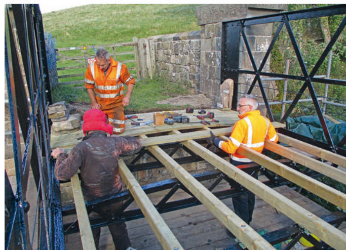
Work being undertaken on the Kirkby Stephen East footbridge. SRC
