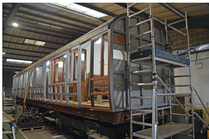
Corridor Lavatory No. 88339 is a unique survivor of its design and is currently undergoing overhaul in the offsite workshops. The external cladding has been removed and new timbers installed to the framework where required.
