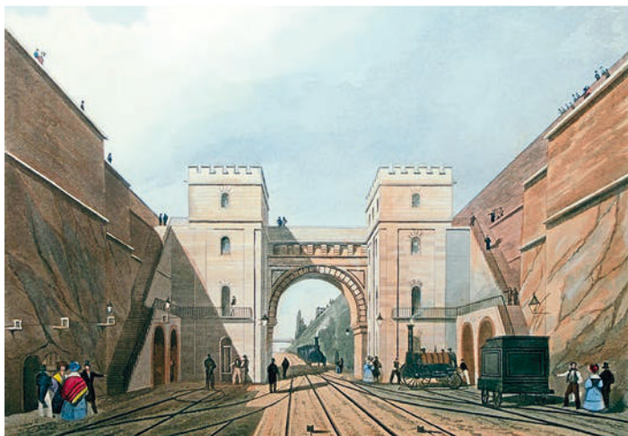
The Moorish Arch which accommodated rope-winding engines to haul trains up the inclines. HISTORIC ENGLAND
