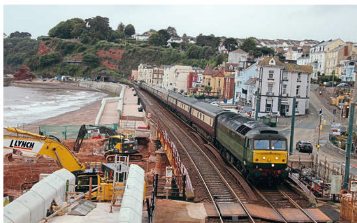
West Coast Railways two-tone green Class 47/8 No. 47815 Great Western and Class 47/7 No. 47746 Chris Fudge 9.7.70-22.6.10 head the return 1Z86 5.50pm Paignton to Birmingham International Northern Belle charter past the Dawlish sea wall works on the evening on September 3. THOMAS MILLS
