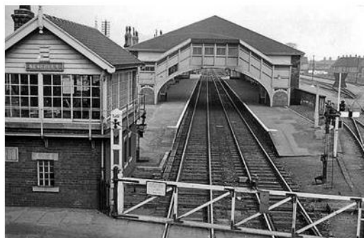
Beverley station and its historic footbridge in 1961.
