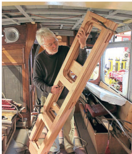
Woodwork supremo Jim Gilchrist checks out the newly-completed platform door frames, built using the originals as patterns. HUGH DOUGHERTY
