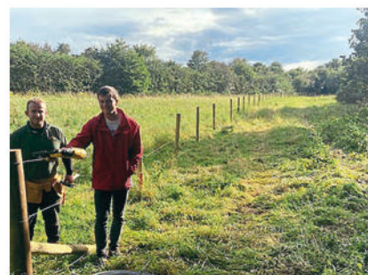
The fence being erected on the border of the land that Melton Constable Trust acquired at High Kelling in October 2021. MCT
