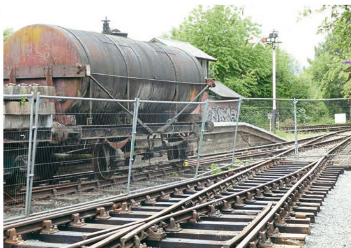
As seen on September 18, the newly completed point which links the Railworld sidings to the Nene Valley Railway, allowing the HST driving cars to be brought in by rail. ROBIN JONES
