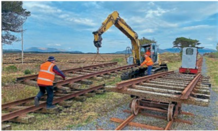
Back to the future! Narrow gauge tracks being used to transport broad gauge track panels, just as contractors might have done building the line in 1895. JIM DEEGAN
