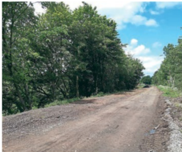
The new Leek station platform will be sited on the left overhanging the embankment. NICOLA FOX
