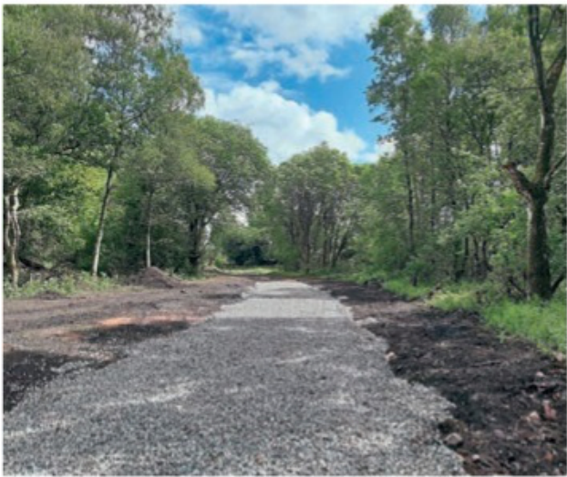
Ballast laid on the east end of the north-to-east section of triangle looking towards Ipstones. The fence dividing the construction area from where the next track will join the existing rails to Leek can be seen in the distance. NICOLA FOX
