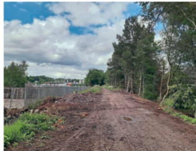
End of the line: The footpath continues to Morrisons but the railway will terminate here. To the left of the railings, sleepers await installation close to the site of what will be the station building. NICOLA FOX
