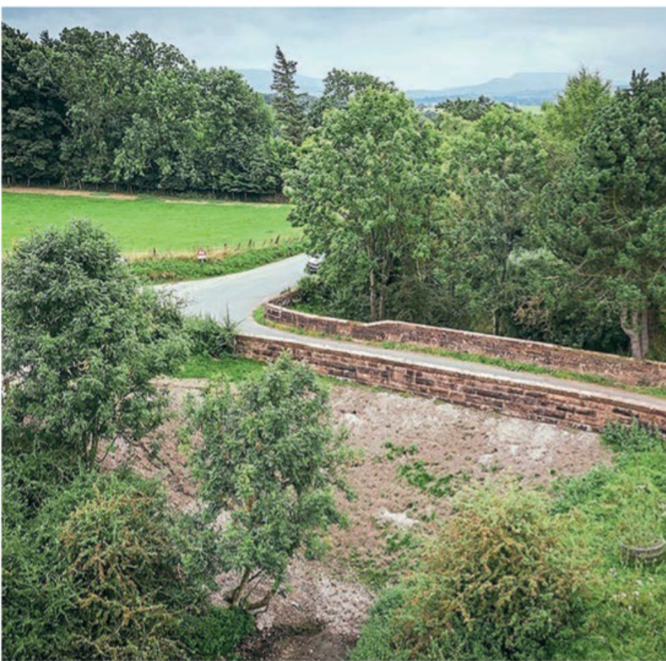
The infilled bridge at Great Musgrave, from which National Highways must now remove the concrete. HRE GROUP
