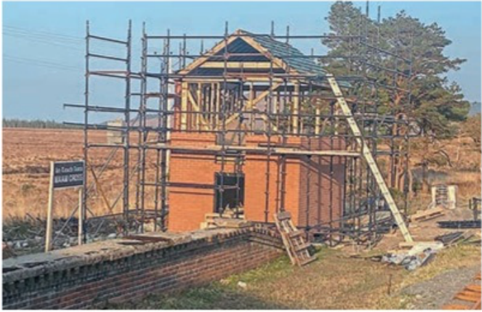
Maam Cross signal cabin rises again above the platform, the cabin's second rebuild in a century. JIM DEEGAN
