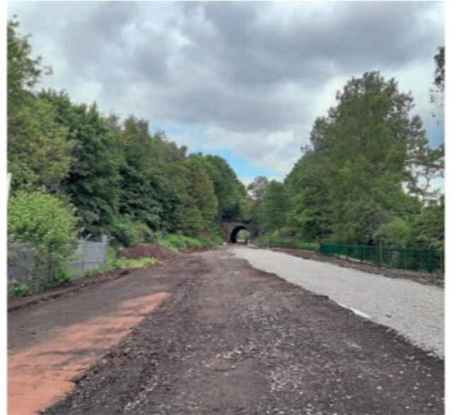
Looking towards Birchall Tunnel, here is where the north-to-south and the north-to-east section of the triangle will meet. NICOLA FOX
