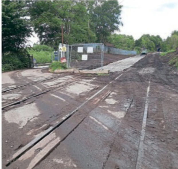
The road crossing with BR-era rails still embedded in the asphalt. Birchall Tunnel can be seen in the distance. NICOLA FOX
