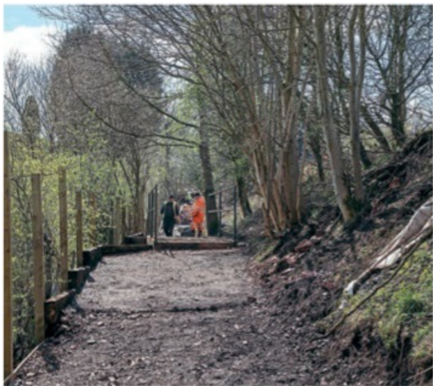
Installing the concessionary footpath and high fence to protect walkers from golf balls. DAVE GIBSON
