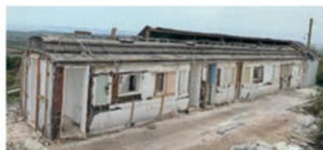
No. 9037 exposed for the first time after the building extensions were removed. PAUL RICE/WSRHT
