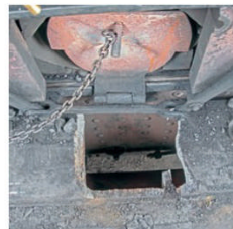
The failed casting on the footplate of No. 813. The transverse spring for the rear drivers was fixed at this point.
