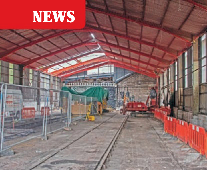
Above: Inside Bridgnorth shed showing the pits fenced off, piling drill and safety netting throughout for the roof replacement on May 12 (taken with permission of Walsh Construction).
