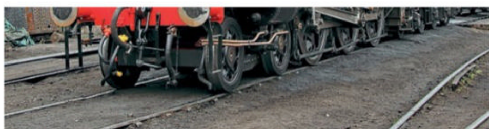
The rail heads in Bridgnorth yard are flat and sinking so need to be replaced.
