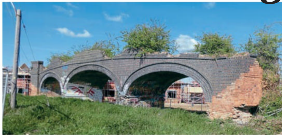
Bridge 234 was once a gateway for rail passengers arriving at Bourne, and now it is surrounded by a new housing estate under construction. As we closed for press, it was still standing.
