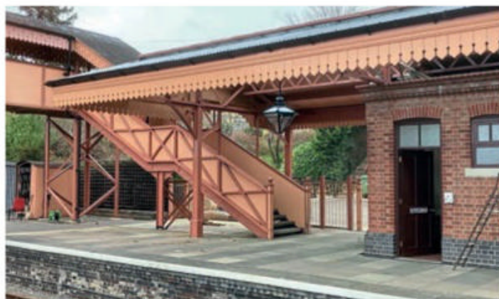
The Broadway canopy extension viewed from Platform 2. DAVID HOLDSWORTH
