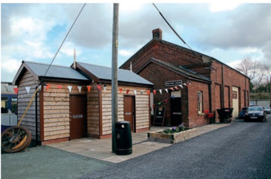
The new toilet block and restored goods shed at Weston Wharf.
