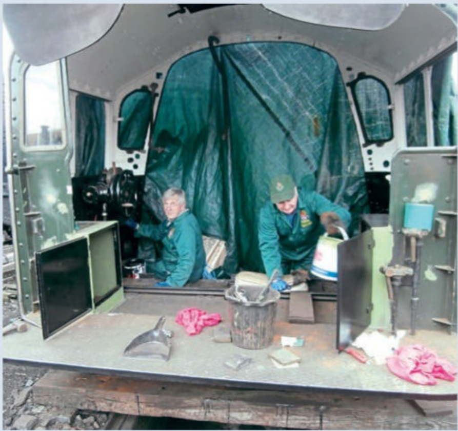
Progress made on the inside of the cab of No. 71000 Duke of Gloucester . The two cabinets have been designed and made by Dave Oliver, the BR Class 8 Steam Locomotive Trust's engineering principal, to house the electrical equipment. The two support crew members at work in the cab are Richard Maxwell (left) and Mark Watts. BRC8SLT
