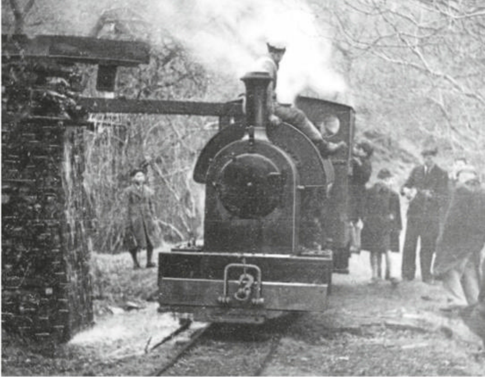
The last recorded time that the original Ty Dwr watering stop was used in 1952 by No.4 Edward Thomas . TR COLLECTION
