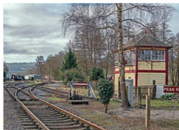
The entrance into Rowsley South.
