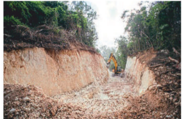
A JCB digger excavating a cutting for the new railway. ST NICHOLAS ABBEY
