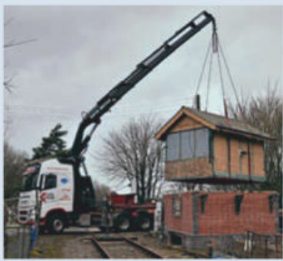
The Spooner Row signalbox craned into its new position at Wymondham Abbey on February 18. MNR
