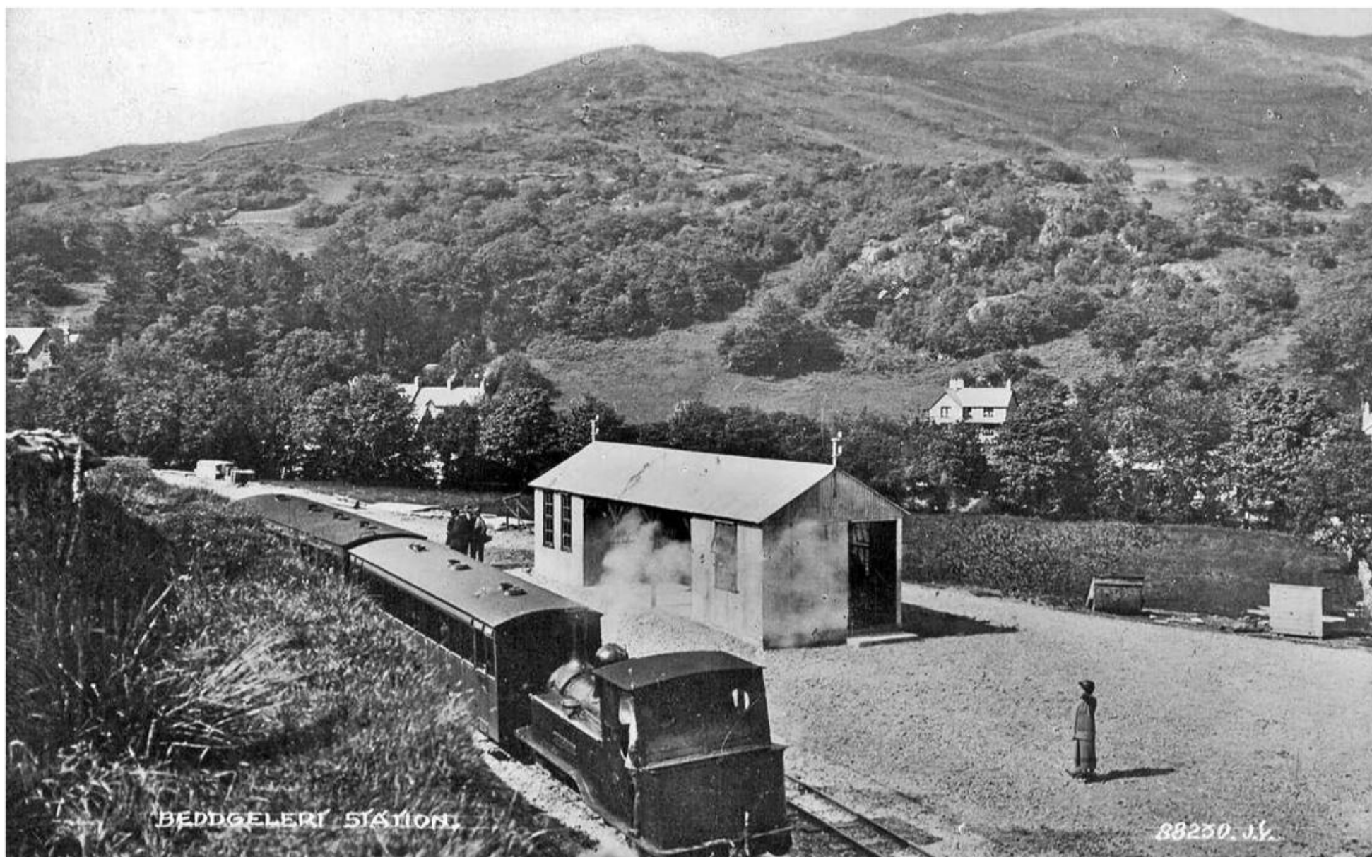
Early visitor: The newly-constructed Beddgelert station hosts a visit of 0-6-4T Moel Tryfan in 1923 on what is believed to be a crew training run prior to the opening of the line in June that year. VALENTINE POSTCARD/WHRHG ARCHIVE
