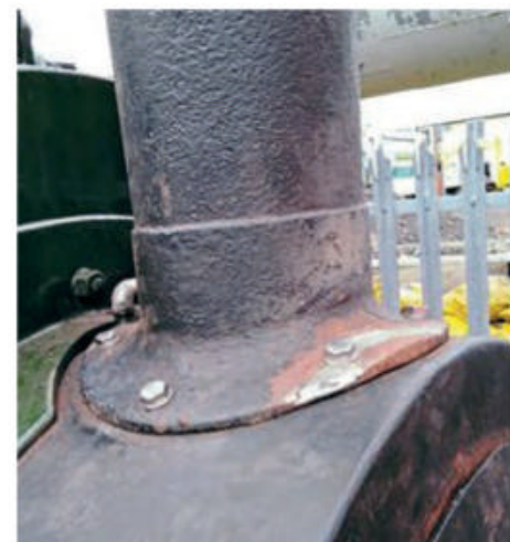
Jurassic 's chimney back in position with repaired section at the front. JULIE BATES/LCLR
