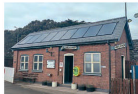
Tywyn Wharf station with newly-fitted flush solar panels. LUKE RYAN/TR
