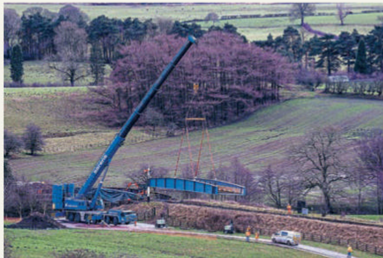
The first of the new bridges being lifted into place on February 14. CHARLOTTE GRAHAM
