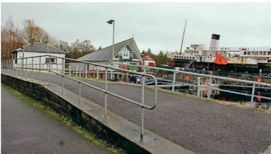
The platform of Balloch Pier station today with the steam winch house in front of the Maid of the Loch's bows, as the steamer sits on the steam slipway on February 2, 2022. HUGH DOUGHERTY
