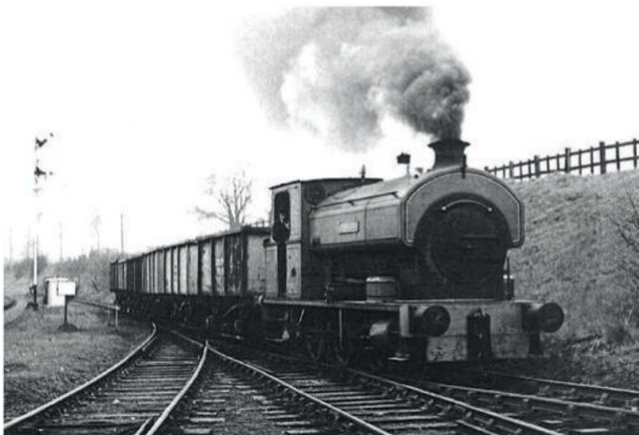
Above: Avonside 0-6-0ST No.1917 of 1923 Pitsford shunting a rake of seven iron ore tippler wagons at Pitsford Sidings in the early 1960s. It was originally preserved at the late Sir William McAlpine's private Fawley Hill Railway and moved to the Nene Valley Railway in 1972. It then moved to the Elsecar Railway where it was overhauled and named Earl Fitzwilliam . It was withdrawn from service there in 2001 and has since been awaiting overhaul. NLR
