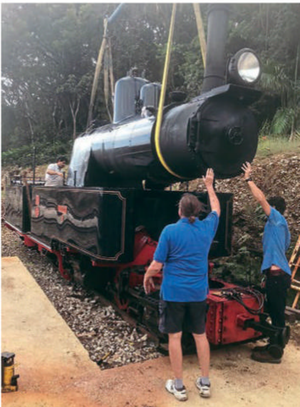
Reinstalling Tjepper 's boiler following repairs. MARTYN WARD
