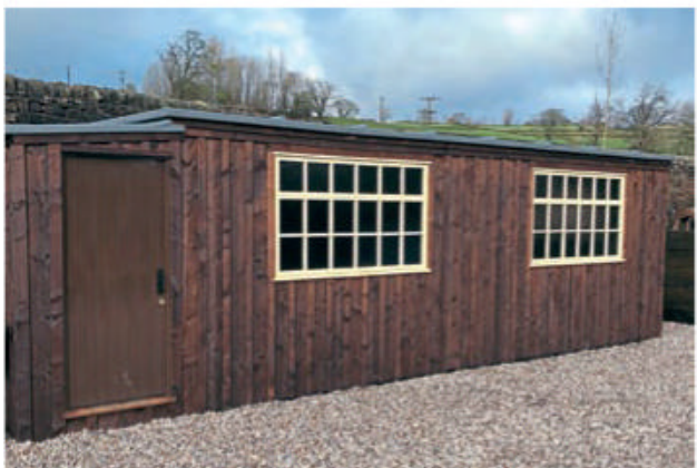
The replica Midland Railway hut which is being transformed into a refreshment kiosk at Oakworth station. SALLY CLIFFORD
