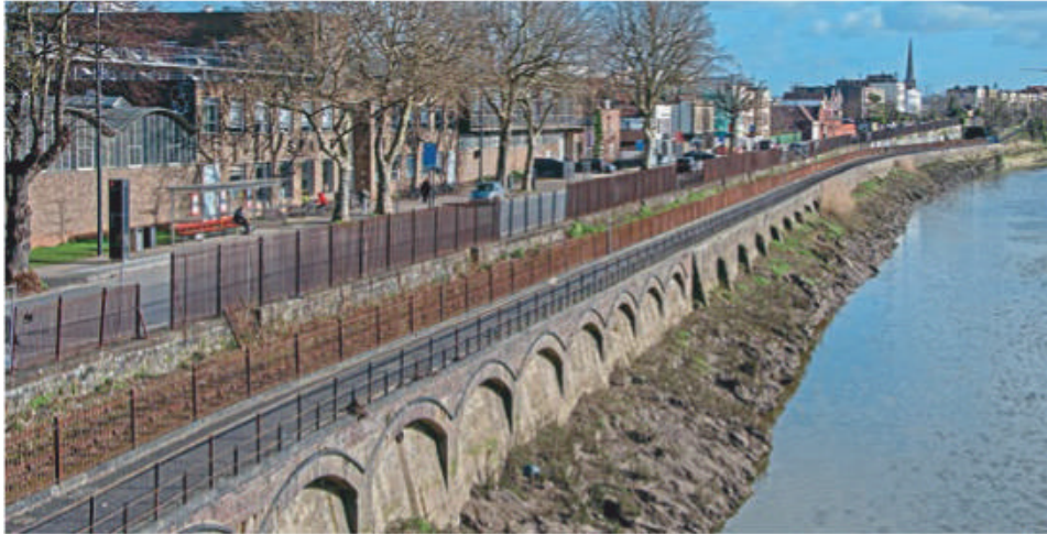
The present Bristol Harbour Railway running line. The bridge in the background is where the line exits the docks, alongside the River Avon and Chocolate Path, which is to be repaired more than three years after it was shut due to serious subsidence. It will be fixed as part of plans to futureproof the historic harbour-side infrastructure, with £2.5 million due to be spent around the Floating Harbour and New Cut over the next two years.
