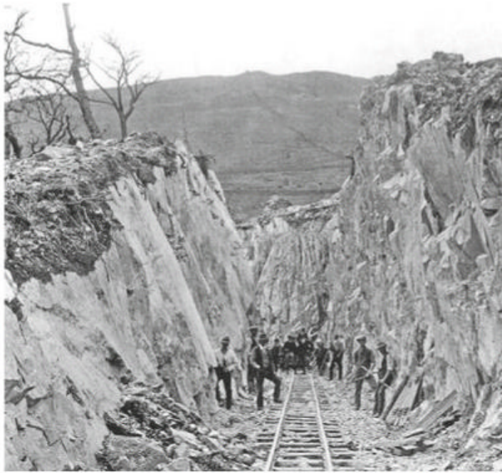
Right: Taking a break: The scale of the operation to build the WHR line is evident as a small army of workers takes a well-earned breather for the photographer at Cwm Cloch cutting above Beddgelert during track-laying prior to the opening in June 1923. MCALPINE FAMILY ARCHIVE
