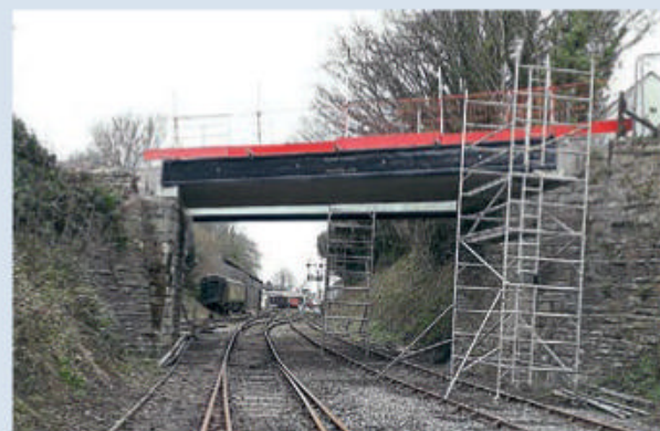
The new Beacon Road bridge seen from the Parkway branch looking towards Bodmin General and awaiting balustrades. BWR
