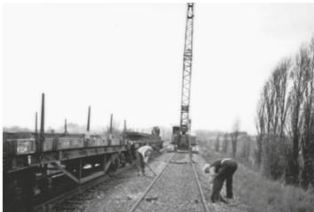
Track lifting underway at Whitehouse West in 1965. LUKE KAY
