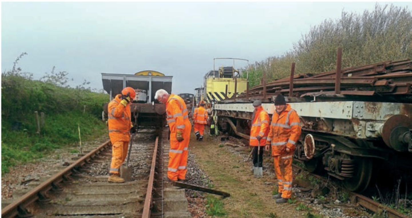
Members of the Lincolnshire Wolds Railway permanent way team checking the alignment of the sleepers for the push towards Pear Tree Crossing.
