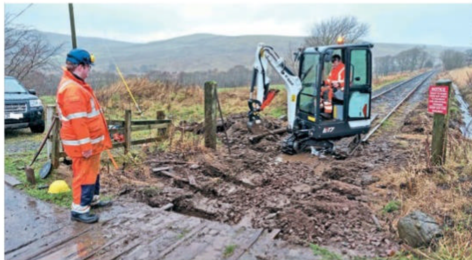
Digging in: Work in progress in bitter winter weather at the Doon Valley Railway's farm crossing replacement site. DVR
