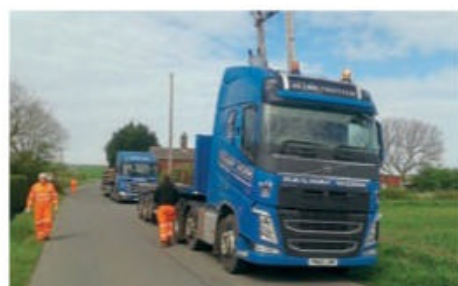
Lorries queueing up to unload some of the hundreds of concrete sleepers delivered to Pear Tree Lane.
