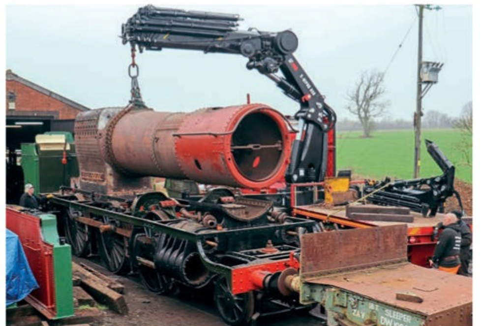
The boiler for GWR 2-6-2T No. 4110 was trial fitted into the frames at Cranmore on January 25. LEE THORP/ESR
