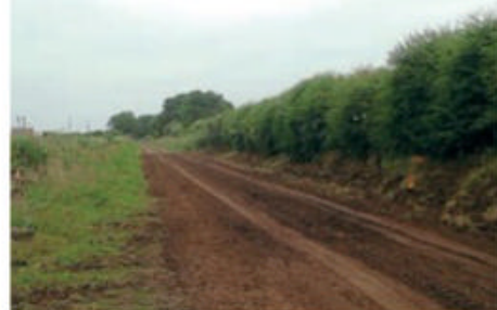
The next stretch of bare trackbed ready for a weed-suppressing membrane to be laid. Pear Tree Lane crossing is in the trees. Some of the hundreds of sleepers alongside the trackbed can be seen in the grass, ready to be swung across. The track is to be laid along where the lorry wheel marks are; the run-round loop will be to the left of this picture.
