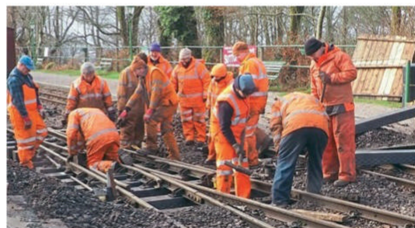
The Lynton & Barnstaple Railway has become the latest narrow-gauge line to replace life-expired traditional wooden sleepers with sleepers made from recycled plastic which should last much longer. At the end of January, volunteers from all over the country descended on Woody Bay station for a working weekend to lay the first plastic sleepers underneath two sets of points in the station and a short section down the line. The plastic sleepers on the right in the photograph, seen being laid under the points, are an inch thicker than the old wooden sleepers stacked up in the foreground. TONY NICHOLSON
