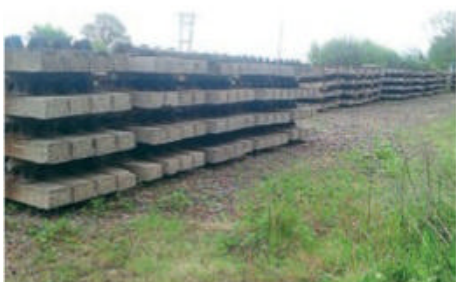
Sleepers stacked and ready to be transported down the cleared trackbed.
