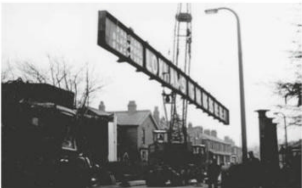
The demolition of the bridge spanning Leyland Road, near the Bridge Inn in Penwortham. ROGER ROBERTS COLLECTION
