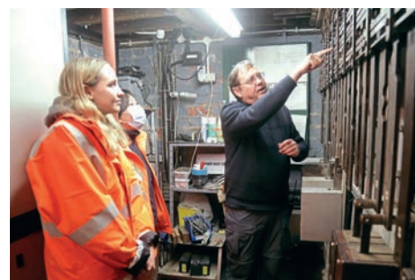
Mechanical interlocking is explained by a volunteer at Chinnor signalbox on November 5.
