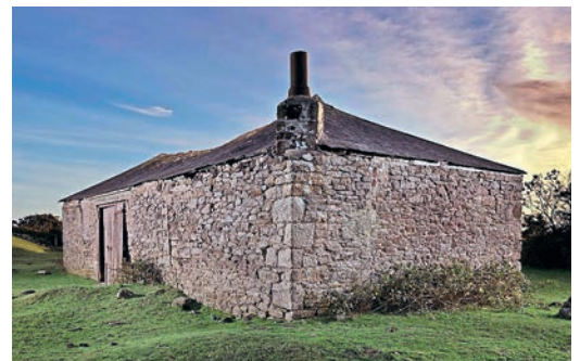
Tyrwhitt's Wharf is built of Dartmoor granite and retains evidence of functional features, such as the tall entrances at either end of the building to allow horses to enter and leave. HISTORIC ENGLAND
