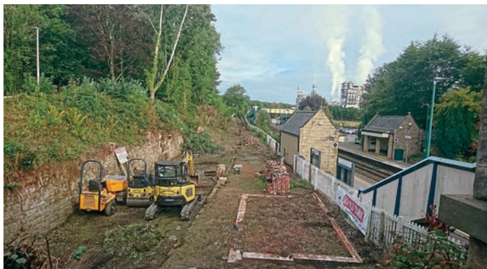
Looking along the newly revealed remains of Chirk's narrow gauge tramway station alongside the main line station. GVT
