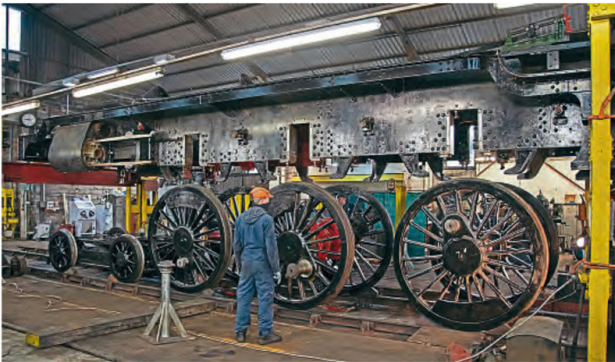
A trial positioning on road four on the lifting jacks is No. 4930 Hagley Hall 's frame and wheels inside Bridgnorth shed on April 21. The track will be infilled with concrete, bringing the floor level.
