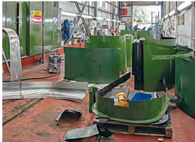
The boiler cladding of No. 4930 being painted in preparation for fitting inside Bridgnorth shed on September 15. This section of the shed will be the entrance for construction works and cordoned off.
