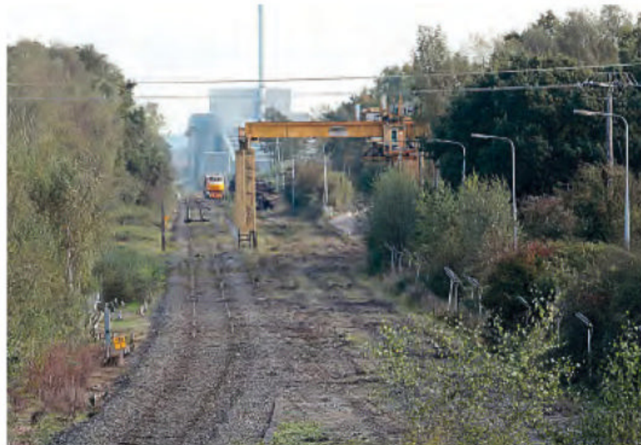
Looking south, October 17 saw track lifting operations south of Calvert station underway. PHIL MARSH
