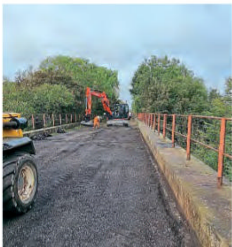
Contractors WL Straughan & Son Ltd start removing the deck material from the Aln Valley Railway's Cawledge Viaduct after AVR volunteers lifted the track. TOM LLOYD/AVR
