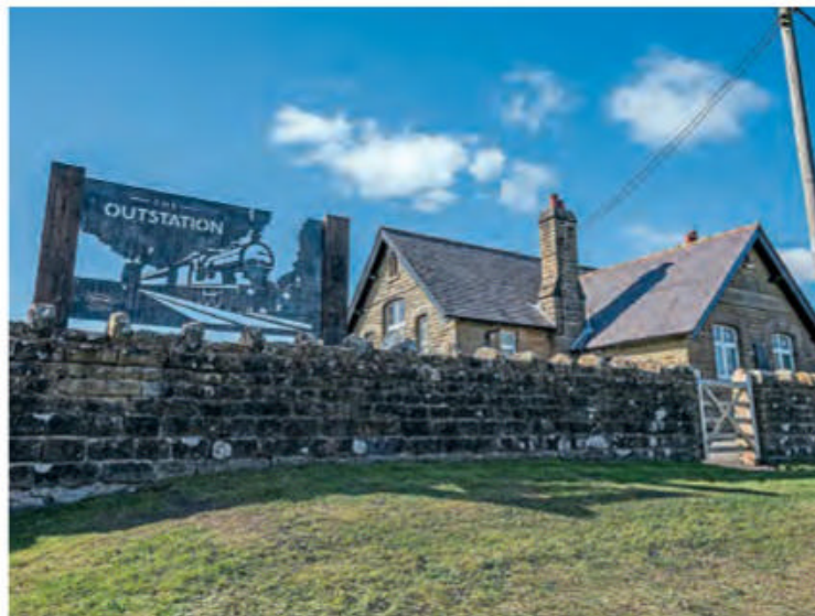
The North Yorkshire Moors Railway's new volunteer development hub, The Outstation, at Stape.
