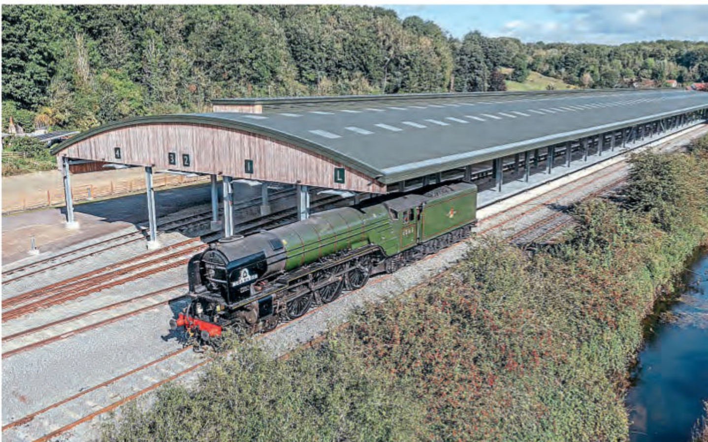
The new £4 million Pickering carriage stable with A1 No. 60163 Tornado in the foreground. CHARLOTTE GRAHAM/NYMR
