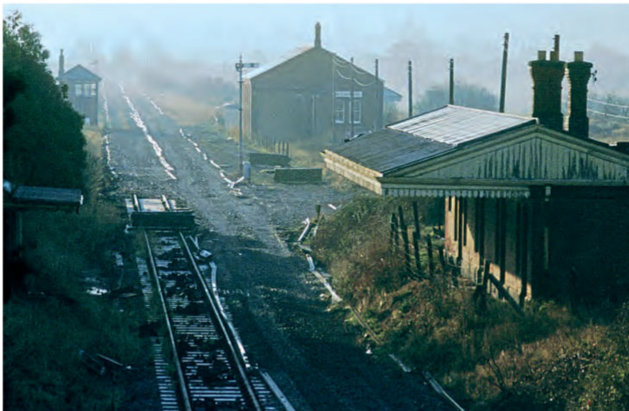
What the preservationists started with: Toddington in 1982, with some track already laid. The building, goods shed and signalbox survive but the platform had been bulldozed. RESTORATION & ARCHIVING TRUST
