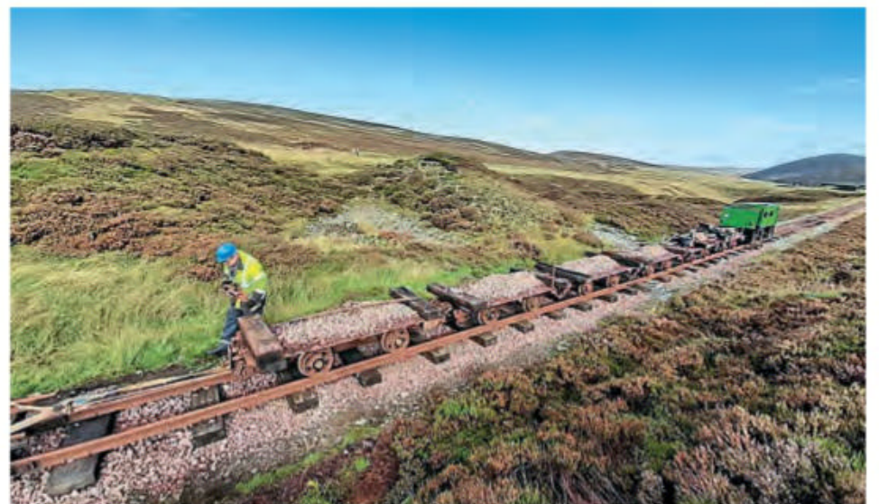
The Leadhills & Wanlockhead Railway works train with new ballast. L&WR
