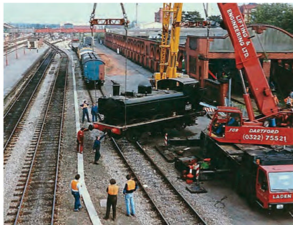
BR(W) 8750 0-6-0PT No. 9682 being craned into the GWR Preservation Group's first base at the Walls sidings, Southall, following its departure from Barry scrapyard in 1982. GWRPG
