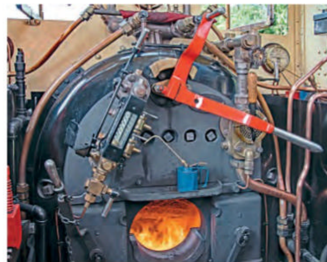
On the footplate of recently restored The Earl , showing the high standard of work and the new firebox brick arch.
