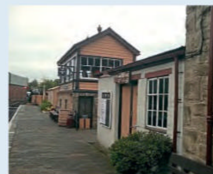
The parcels office at the end of Bridgnorth station. TONY BENDING
