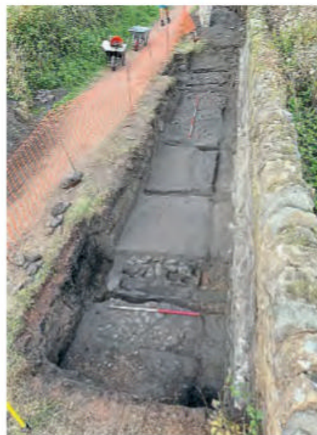
The 2021 excavated section showing the space between the rails, sleepers and the cobbles laid between the three levels of rails.
