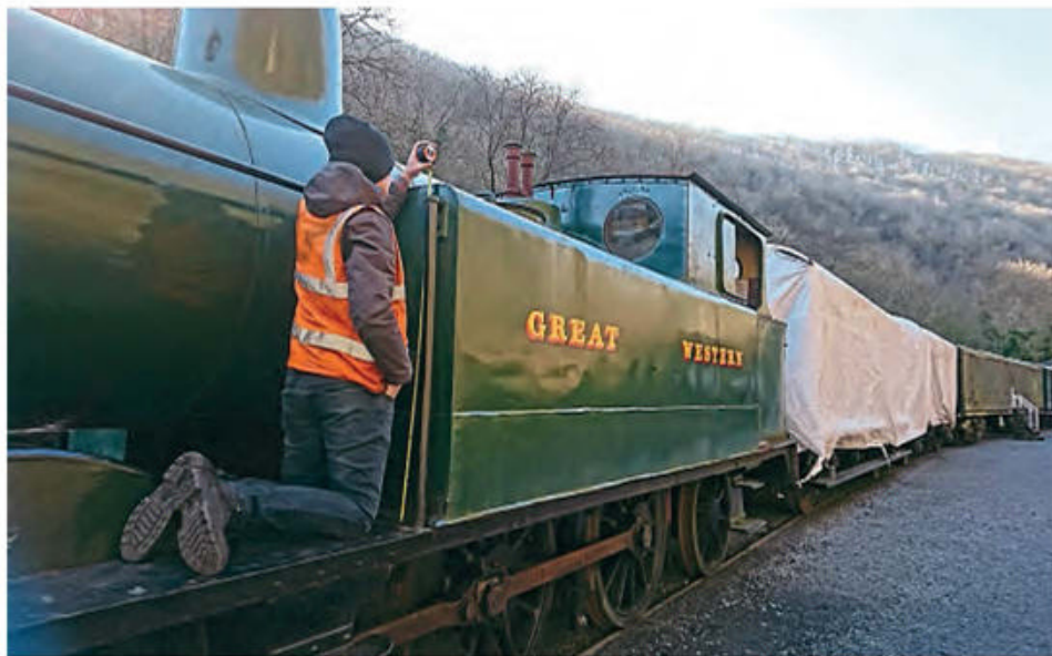
Measuring up Taff Vale Railway 0-6-2T No. 28's old water tank before CAD modelling the new one. GR/ NRM
