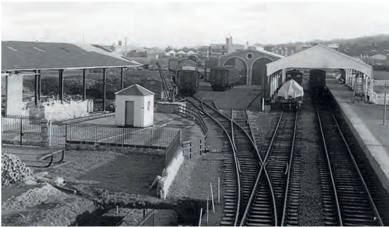
Taking shape: By 1984, all the bones of today's Bo'ness station were there or under construction. SRPS
