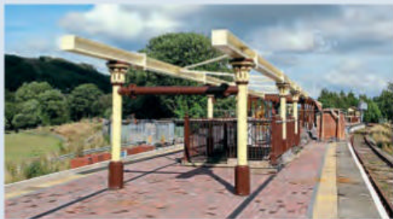
The new longitudinal beams and bracing now in place on the columns around the subway stairway at Corwen. PETER NEVE
