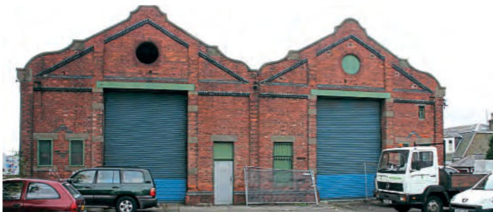
Maryfield tram depot, which will house Dundee Museum of Transport from 2024. Its carbon neutral plans will be on show at the Cop-26 climate change conference in Glasgow in November. HUGH DOUGHERTY
