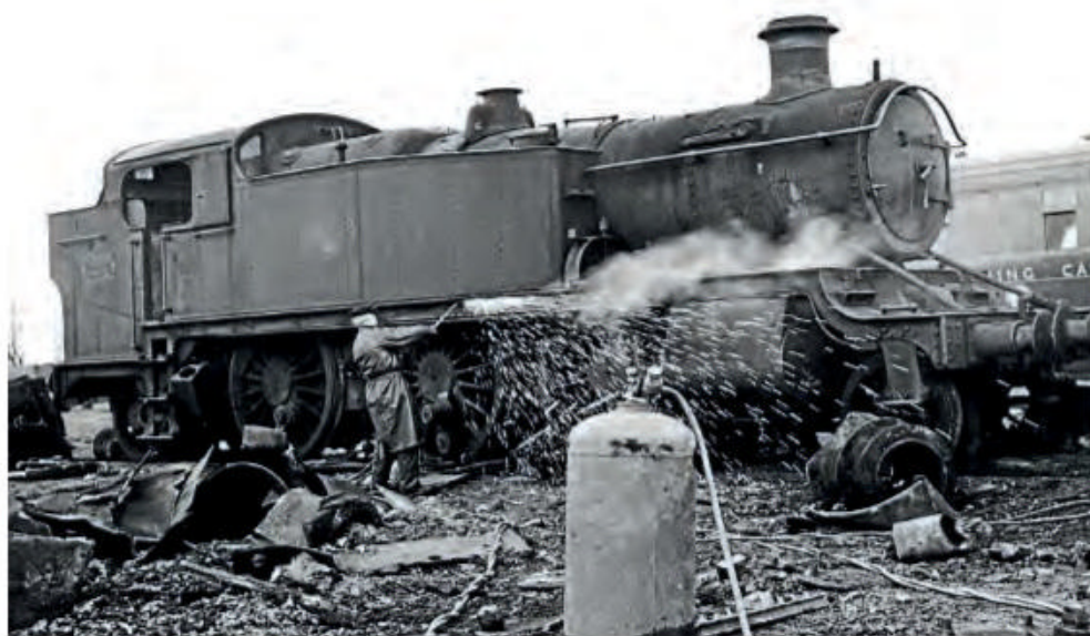
A sad end for 5101 class large Prairie tank No. 4155, as the scrap men start cutting it up at Long Marston on February 2, 1966.
