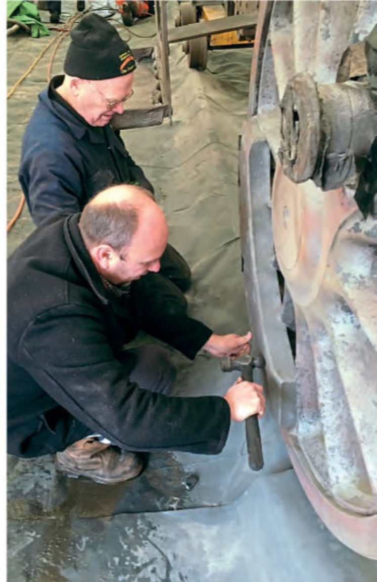
Left: Mike Solloway working on the new cab spectacle plate with Dan Wigg looking on. The round spectacle windows are visible, returning No. 2874 to its original condition. DAVID HOLMES
