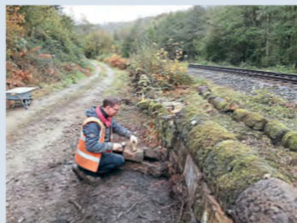
A volunteer carrying out masonry work on a lineside wall. NYMR
