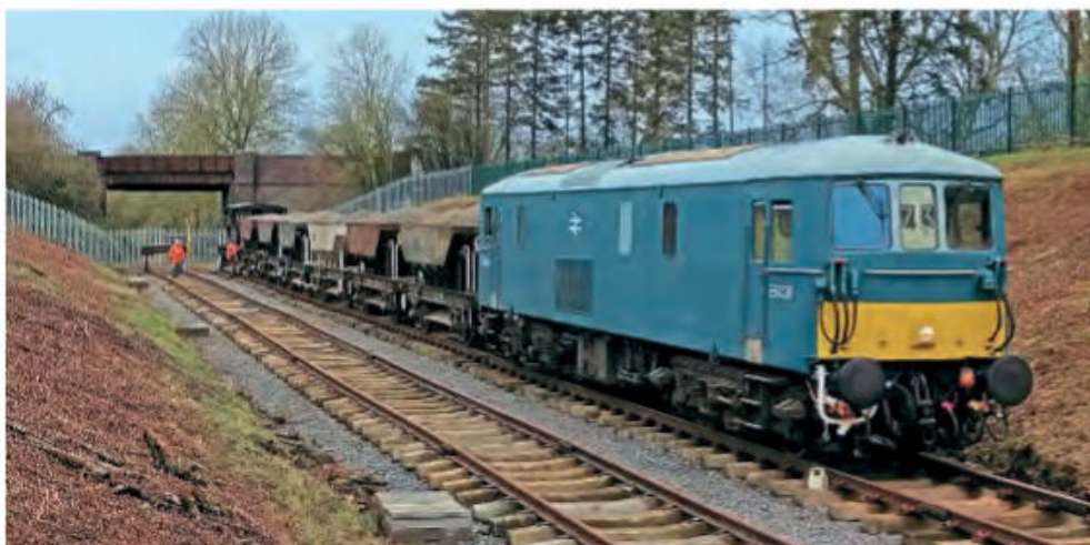
Class 73 electro-diesel E6036 (73129) with an engineering train at the Gloucestershire Warwickshire Railway's northern railhead in January 2018, about to ballast one of the two headshunts at Broadway. The palisade fencing marks the G/WR's boundary, the trackbed beneath Springfield Lane Bridge and northwards to Honeybourne being owned by Railway Paths Ltd. JO ROESEN
