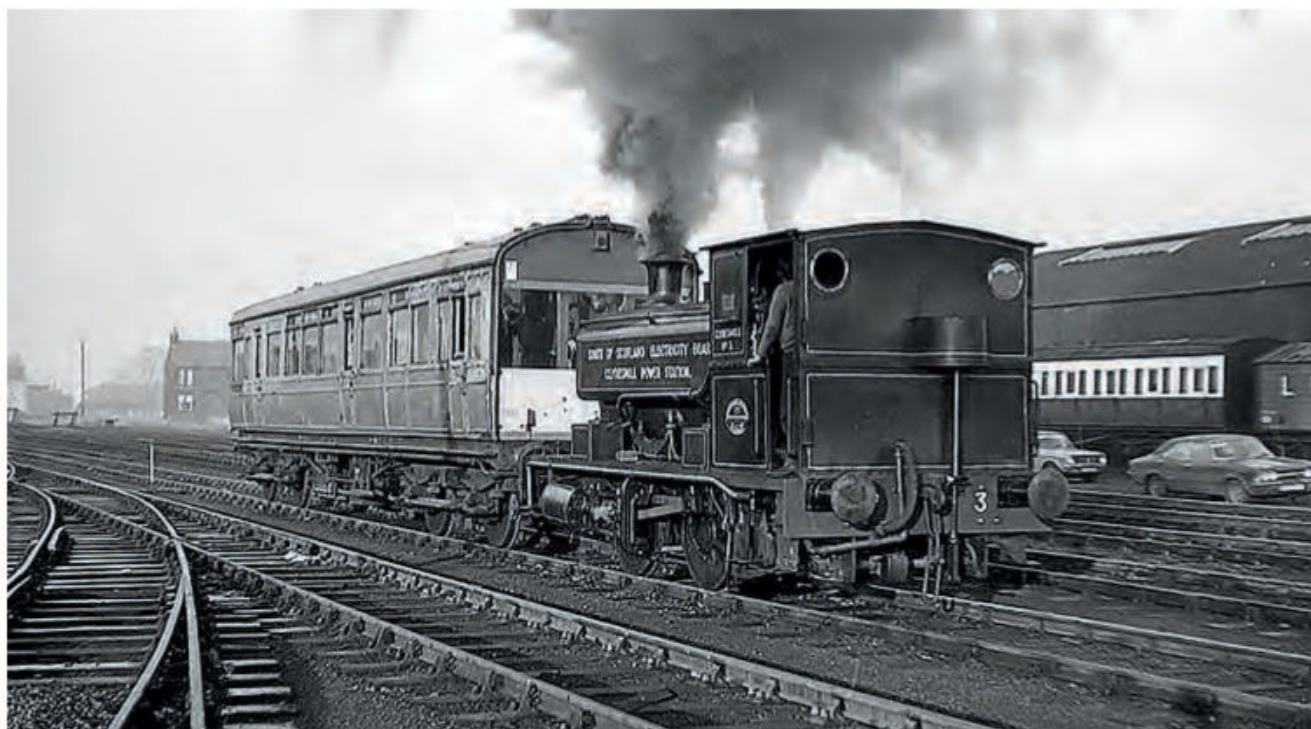
Early days of the SRPS with 1928-built Barclay 0-4-0ST Clydesmill No. 3 in steam at Falkirk in 1971. Gifted to the society, the locomotive beat the BR steam ban by being driven from Clydesmill Power Station to Falkirk under its own power, with a sympathetic BR turning a blind eye! JACK KERNAHAN
