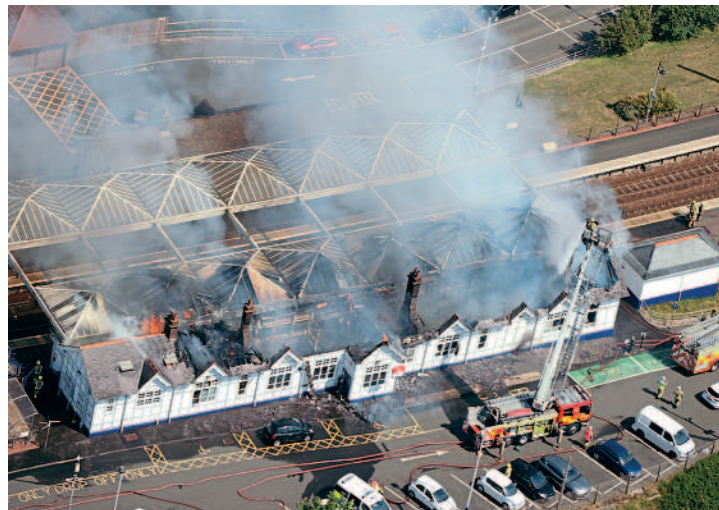
An aerial view of the fire which tore through Troon station's iconic Victorian building on July 17. SCOTRAIL
