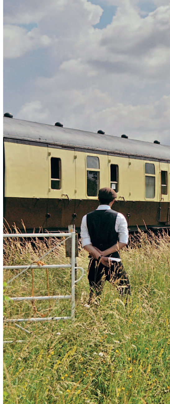
Left: The derelict Bristol & Exeter Railway signalbox at Stoke Canon in Devon, which the Cholsey & Wallingford Railway hopes to rebuild at Wallingford. TOBY JENNINGS
