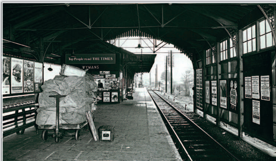
The canopy at Maidenhead, in a picture believed to date from 1961. RAILWAY HERITAGE TRUST
