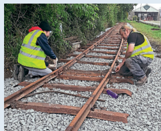
Laying 3ft gauge track at Belturbet station. BHR
