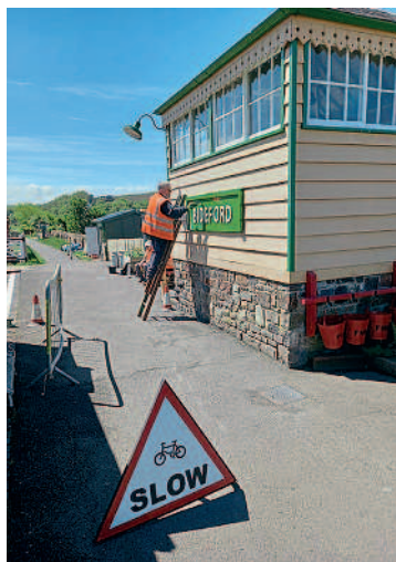
Left: Sprucing up the signalbox at Bideford station. BRHC
