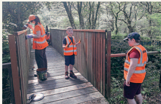
Young volunteers painting the footbridge at Dolgoch station. IAN EVANS/TR
