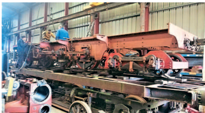
Drumboe's rolling chassis has been moved into the Henry Dunleath workshop at Whitehead. HEI
