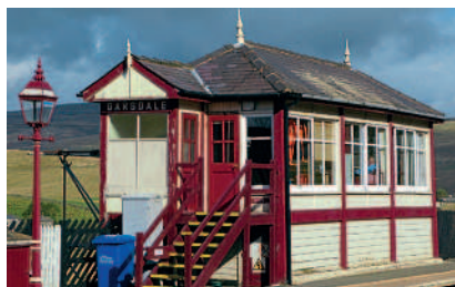
Garsdale's Grade II* listed signalbox. MARK HARVEY/FRIENDS OF SETTLE TO CARLISLE LINE
