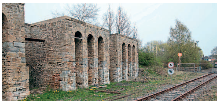
The coaling drops comprise a very early and rare example of a purpose-built facility for refuelling steam locomotives. HE
