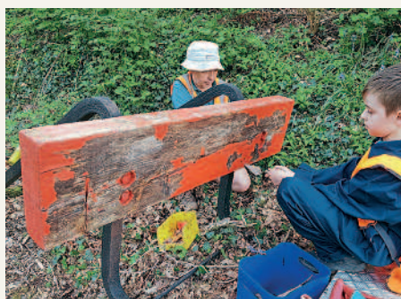
Team buffer stop work in progress during the Tracksiders' week. SALLY HIRST/TR
