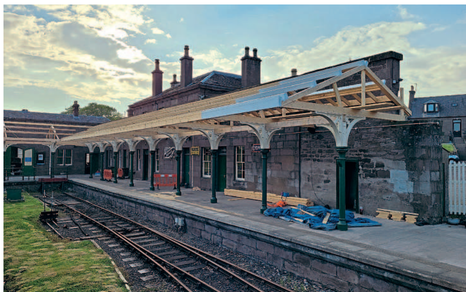
Reconstruction of the first section of the canopy is well advanced at Brechin station. CALEDONIAN RAILWAY
