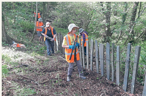
Maintaining the Talyllyn Railway's historic lineside fencing. IAN EVANS/TR
