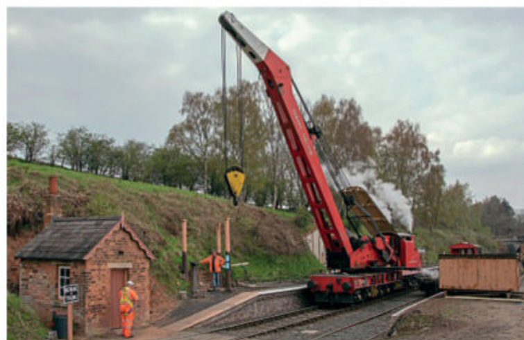
The 1960-built 10-ton Cowans & Sheldon steam crane that normally resides at Bridgnorth lifts the water tank at Eardington on April 20. JOHN TITLOW
