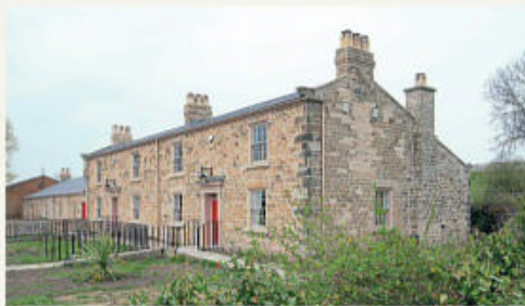
Newly-restored Hackworth House at Locomotion in Shildon, built c1830-1831 for Stockton & Darlington Railway locomotive superintendent Timothy Hackworth. LOCOMOTION
