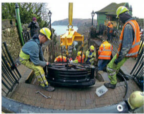
Installing the new Top Wheel installation on the Lynton & Lynmouth Cliff Railway. LLCR
