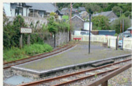
Corris station, where a new round-facility is to be provided. ROBIN JONES
