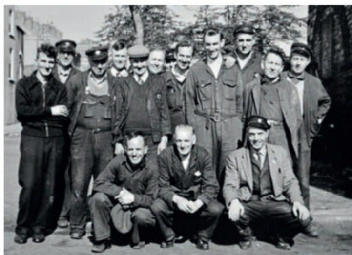
The museum has recently received this picture of GNR(I) staff at Foyle Road station. FVRM
