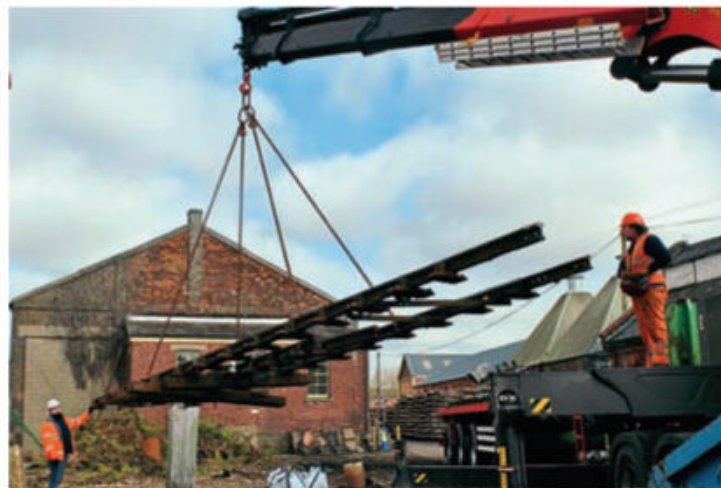
Trackwork for the replacement siding, donated by Sonic Rail Services, is seen being unloaded at Dereham. MNR
