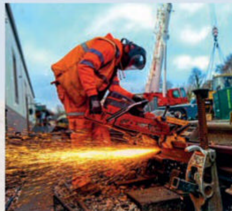
Cutting the closure rail on a switch panel refurbishment at Churston station on the Dartmouth Steam Railway. STEWART MACKENZIE/DSRRBC
