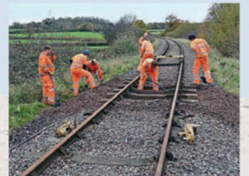
There were plenty of temporary tie bars holding failed sleepers on the old concrete section of the West Somerset Railway, which have been replaced with new timber sleepers. WSR INFRASTRUCTURE ENGINEERING
