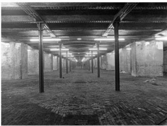
The New Warehouse basement in 1987, when it was used as a museum store. SCIENCE MUSEUM GROUP
