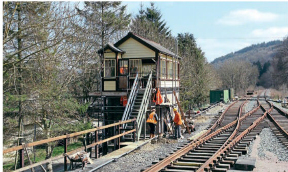
Work on the completion of the new Corwen terminus continues, as it is a Llangollen Railway Trust project outside of the administrator's remit, and manpower attendance has been within the Welsh Government's lockdown guidelines. This April 4 view shows the access path and fencing with the new stairway and renovated access porch for the former Weston Rhyn signalbox, and its new windows. The points and siding all need ballasting and tamping when operations can resume and a ballast train can work through. PETER NEVE/LRT
