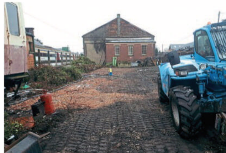
The siding which once ran up to Dereham's goods shed is to be re-laid. MNR
