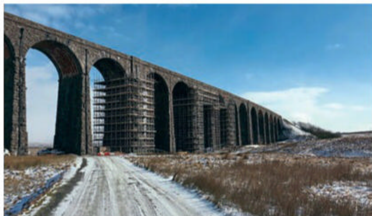
Majestic Ribblehead Viaduct in February's snow, surrounded by huge scaffolding towers built for the repairs to take place. NETWORK RAIL
