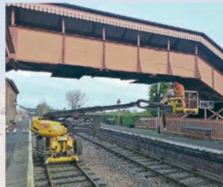
Graham Cole consultants carrying out winter bridge inspections between Bishops Lydeard and Williton on the West Somerset Railway. WSR INFRASTRUCTURE ENGINEERING
