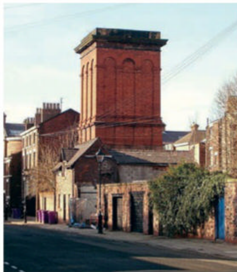
A ventilation shaft for Wapping Tunnel in Liverpool's Blackburne Place. DAVE ROOT
