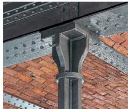
Ceiling detail preserved and restored in the new gallery. MOSI
