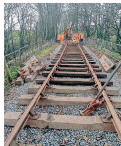
Pushing ahead despite the pandemic: Track-laying across Prospidnick bridge and along the alignment towards the old cutting. HRPS
