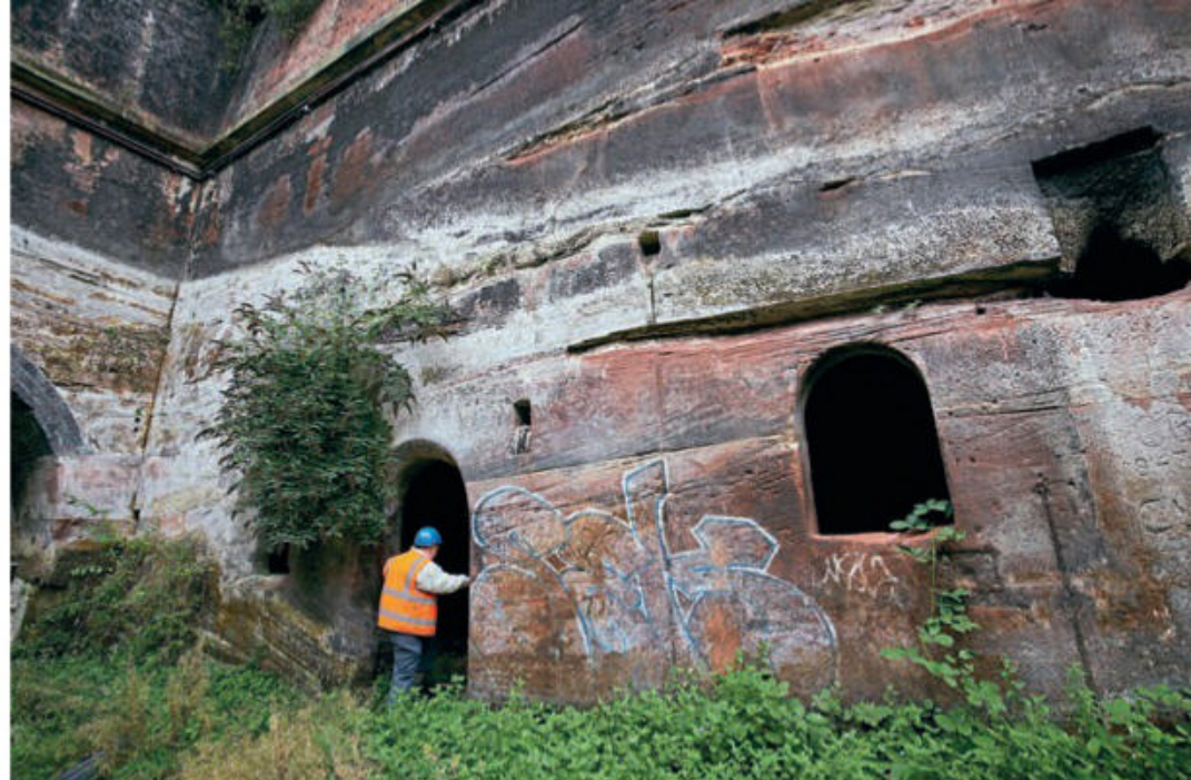
Inspecting the remains of the cutting brickwork. LMRT
