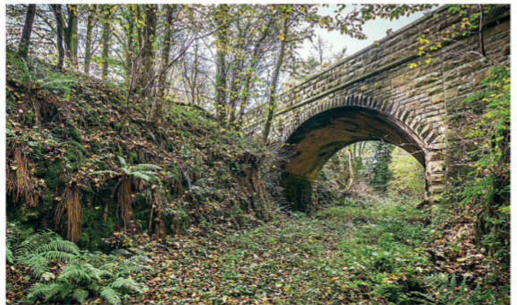
One of the bridges on a proposed greenway at Alnwick in Northumberland, which are to be infilled despite local objections. HRE GROUP
