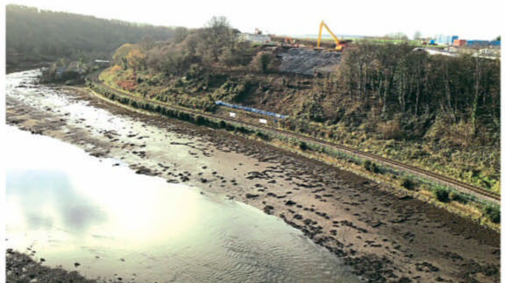
Major work has been carried out on the Esk Valley line into Whitby in a bid to prevent a landslide. NETWORK RAIL
