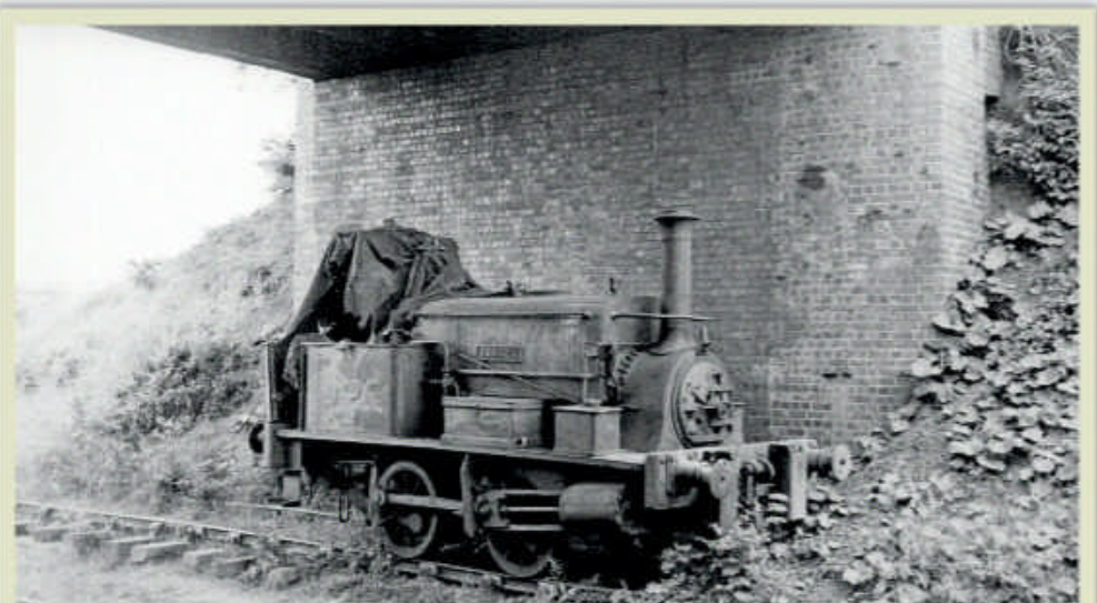
Rusting merrily away, Manning Wardle 0-4-OST No. 1088 Sankey is parked permanently under Camp Lane bridge, as seen in 1935. CSRM
