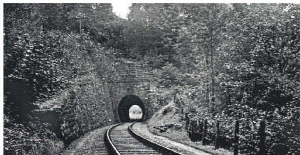
As it was: The eastern entrance to Bobbin Mill 'Big Tunnel' on the Cockermouth, Keswick & Penrith Railway in 1935, looking towards Keswick. The tunnel, which was filled in when the line closed in 1972, has been reopened as part of a restored railway trail. CUMBRIAN RAILWAYS ASSOCIATION
