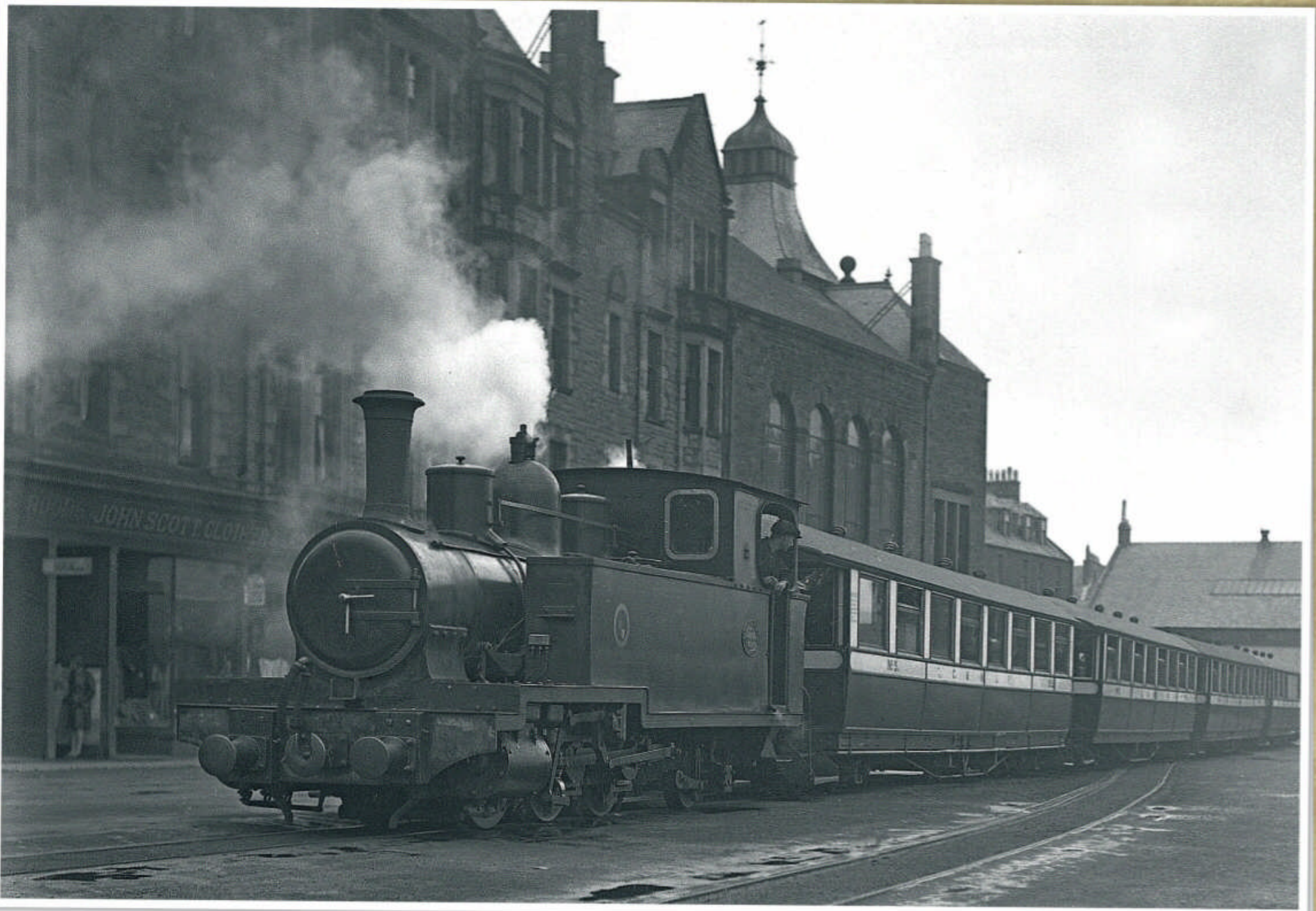
An Andrew Barclay 0-6-2T heads a Campbeltown and Machrihanish passenger train in Kintyre in 1930. Only three other passenger-carrying lines in the British Isles operated on 2ft 3in gauge, all of them in Wales – the Corris Railway, the short-lived Plynlimon and Hafan Tramway and the Talyllyn Railway. Opening in August 1906, the line was an immediate success, attracting 10,000 passengers in its first three weeks of operation and replacing the horse-drawn tourist charabanc traffic in Campbeltown. Like many others however, the railway fell victim to competition from motor buses and closed in May 1934.
