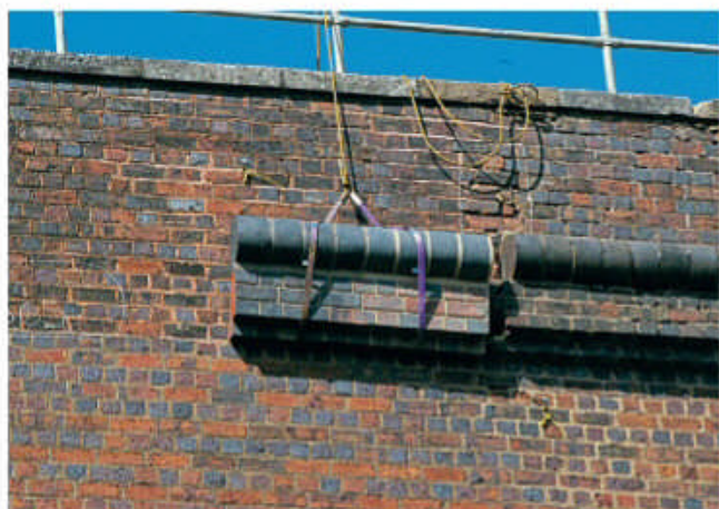
The new glass reinforced plastic corbelling is lowered into position. JONATHAN SYMONDS
