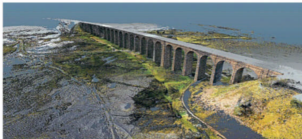
The computer-generated image of the 440-yard Ribbleshead Viaduct, seen like never before, is a major tool in its current maintenance schedule. NETWORK RAIL
