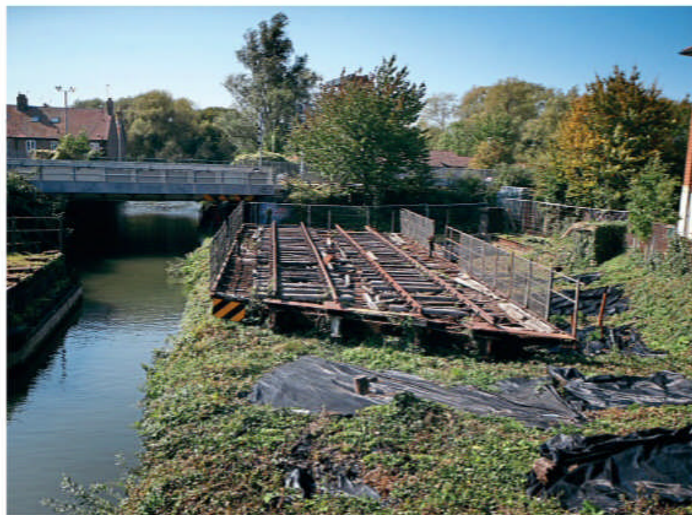
Enabling works in March 2019 saw Oxford Preservation Trust members turn the LNWR Rewley Road swing bridge onto the bank as a precursor to restoration. OPT
