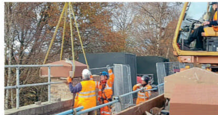
Above: Made from sandstone recovered from the Liverpool & Manchester Railway, one of the new capping stones is manoeuvred into place. SVR
