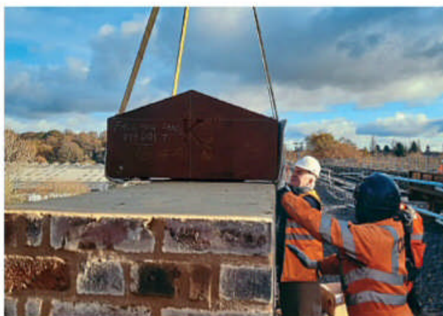
Cap that! Philip Chatfield supervising the installation of one of the capping stones at the viaduct. CAN
