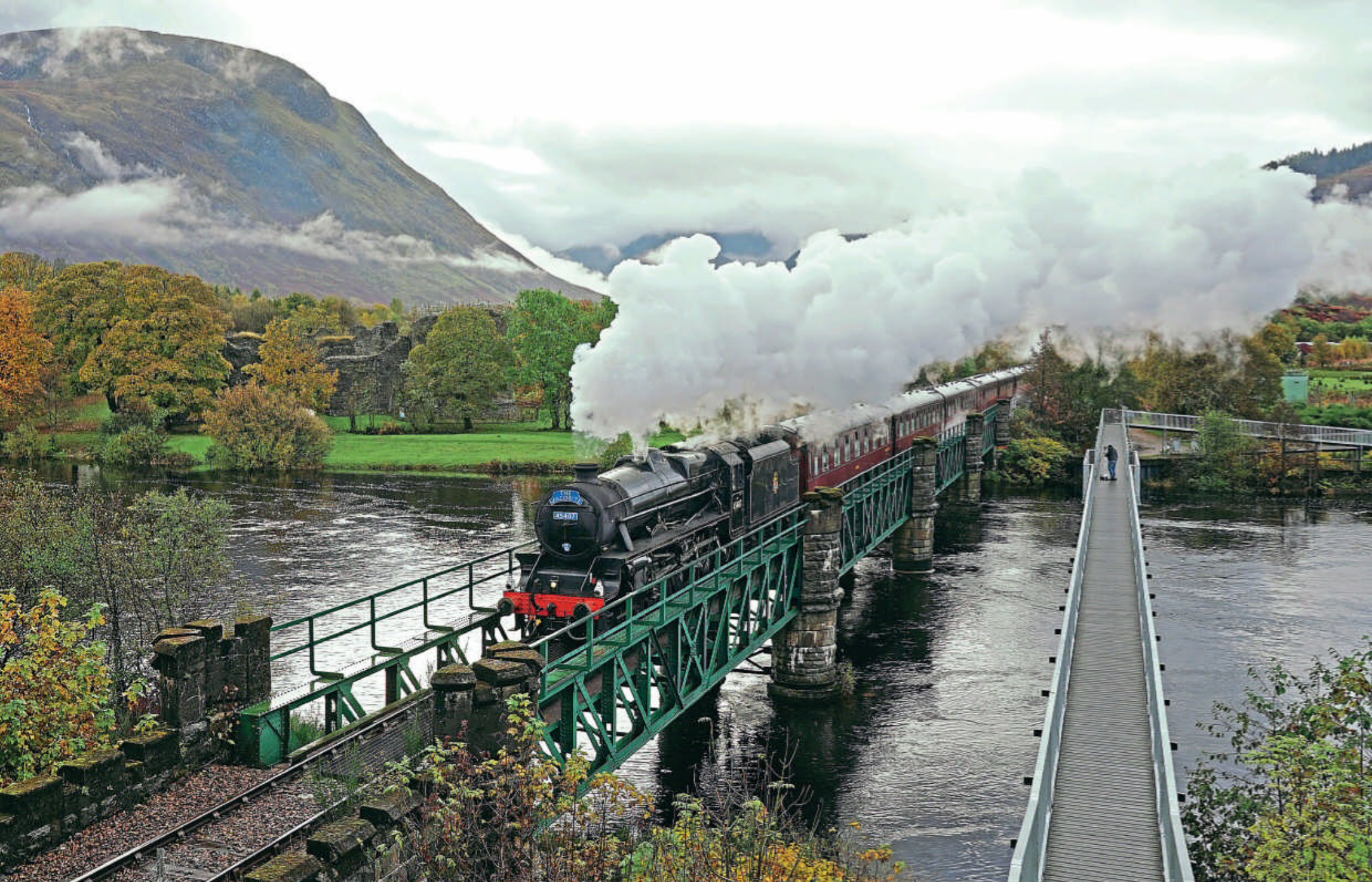
Bookings are now being taken for West Coast Railways' 2021 'Jacobite' season. 'Black Five' No. 45407 The Lancashire Fusilier is seen crossing the River Lochy bridge at Lochside in Fort William on October 21. GAVIN THOMSON
