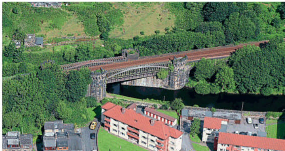
Aerial view of George Stephenson's Gauxholme viaduct. NETWORK RAIL
