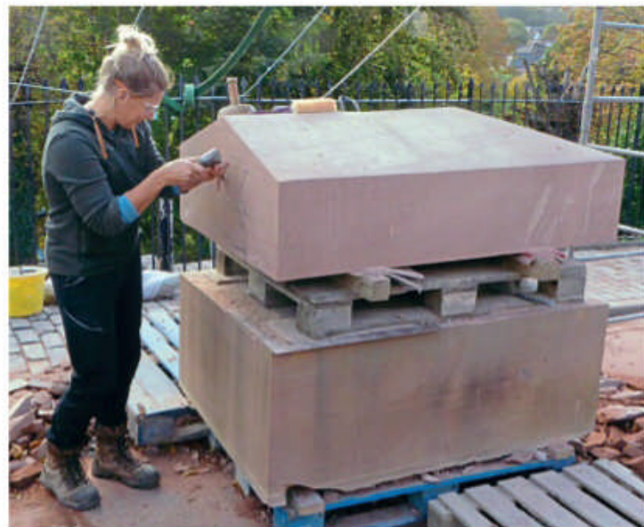
Above: Made from sandstone recovered from the Liverpool & Manchester Railway, one of the new capping stones is manoeuvred into place. SVR
