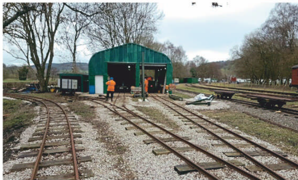
The Ashover Light Railway Society's 'Tribute Line' at Peak Rail's Rowsley South station taking shape. ALRS
