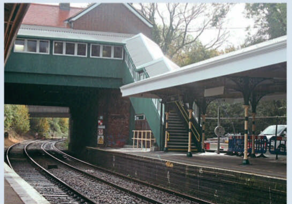
The new footbridge at Eridge station. NETWORK RAIL
