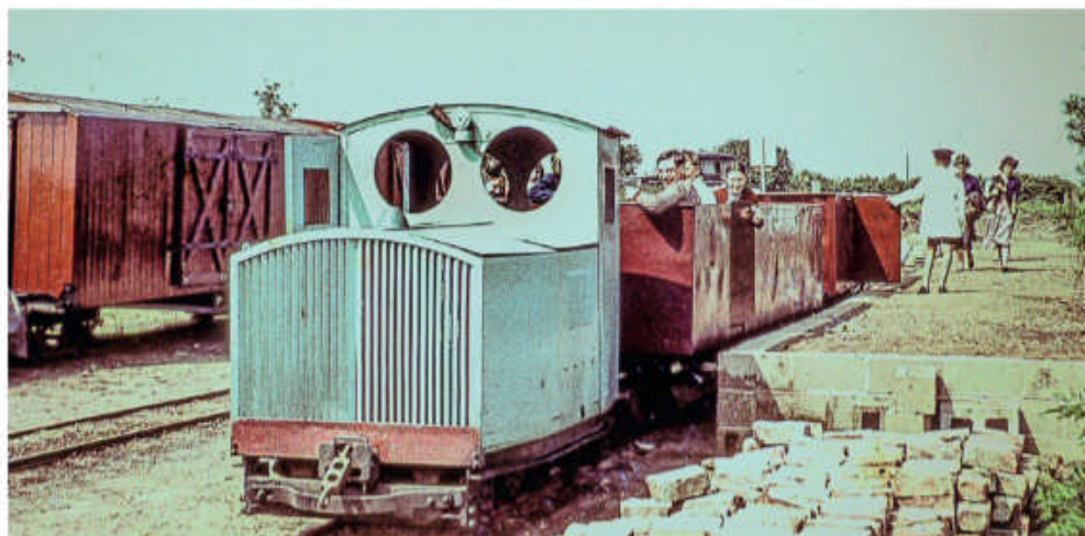
May 22, 1961 the platforms at North Sea Lane and Beach had been completed and an extra carriage had been built. Passengers are loaded into the two carriages at North Sea Lane, prior to setting off for Beach. The guard in short trousers and an oversized white jacket is still a volunteer in 2020. MIKE SWIFT
