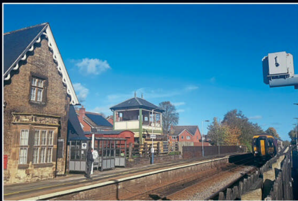
Lowdham station signalbox relocated next to the Grade II listed station building, on the opposite side of the line from its original position. HWA
