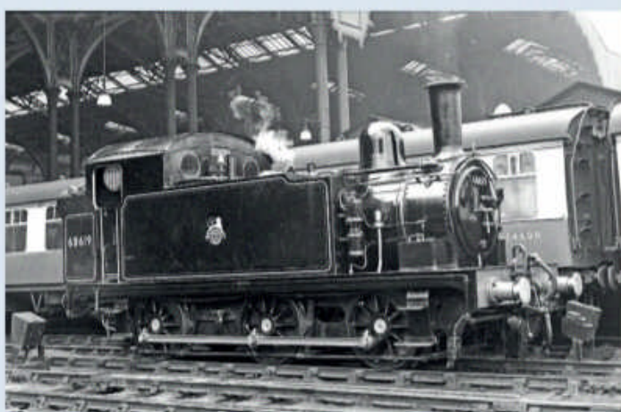
Veteran on parade: Immaculate J69 class No. 68619 on station pilot duty at Liverpool Street on May 11, 1957, when the 0-6-0T was 53 years old. One of the GER veteran's successors in the role, preserved Class 08 D3690/08528, has relocated from the Great Central Railway to the Derwent Valley Light Railway in York to become one of three operational ex-BR diesels on the line. RC RILEY/TRANSPORT TREASURY
