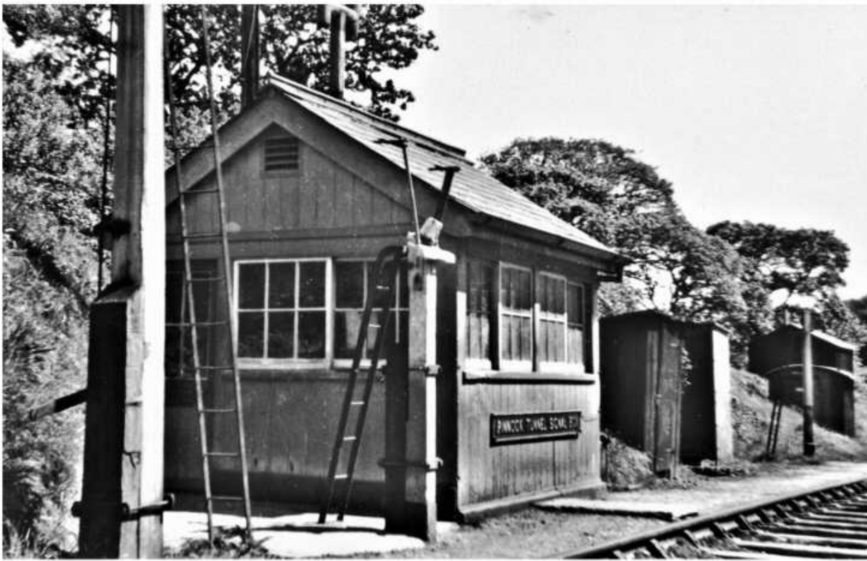
Above: The ground level intermediate signal box at Pinnock was located just on the Fowey side of the tunnel and controlled no pointwork but was an important means of breaking up the section between Fowey and the box at Par Bridge level crossing, particularly when trains got into difficulties on the steep grades. M Dart/J Vaughan Collection
