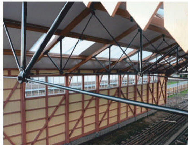
A view of the interior of the Maidenhead canopy relocated at Wallingford. TONY STEAD
