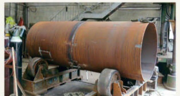
The new boiler barrel for Collett auto tank No. 1420 assembled at Buckfastleigh. SDR
