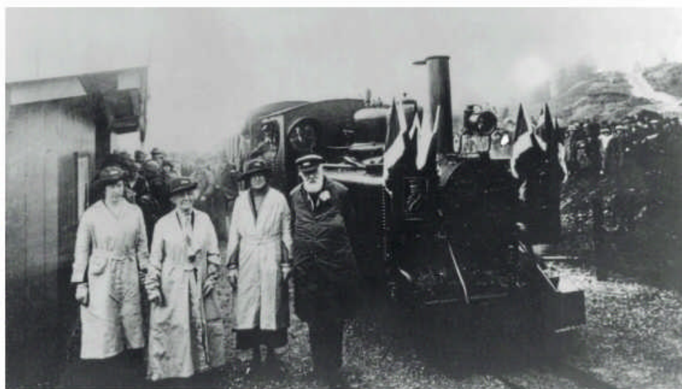
Baldwin 4-6-0T Joan and its train at the Ashover Light Railway's opening ceremony at Ashover Butts station on April 6, 1925. CSRM
