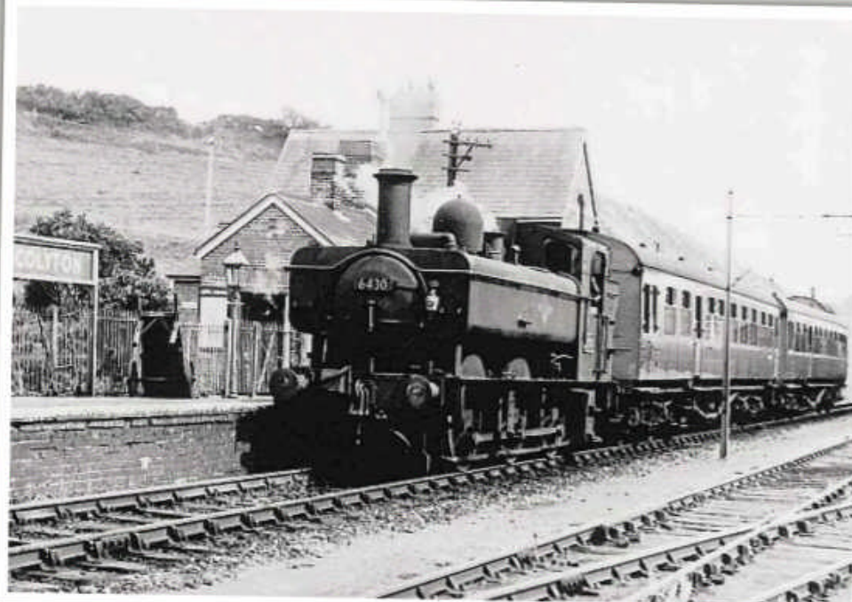
Colyton station with GWR pannier No. 6430 heading a branch train. No. 6430 was shedded at Exmouth Junction and Yeovil in latter BR days, and is now based on the Llangollen Railway. ST
