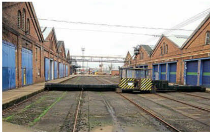
The incident repair and west repair shops at Wolverton Works are now likely to remain. PHIL MARSH
