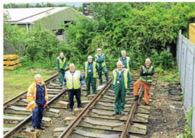
Track panels being laid at CTL Seal to receive the B17 tenders, and for a Clan Project requirement. CHRIS JONES/CLAN PROJECT
