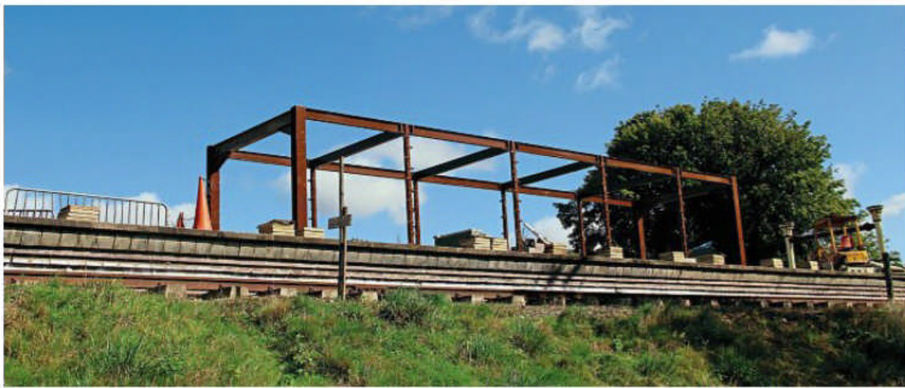
The fabricated steelwork for the on-platform waiting room as erected presents an impressive structure as viewed from the town car park. GEORGE JONES
