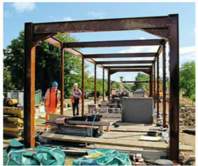
A platform level view of the steelwork structure. GEORGE JONES
