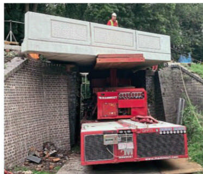
Carefully does it: the new bridge deck lifted on to the abutments using a Mammoet crane on September 10. GCR
