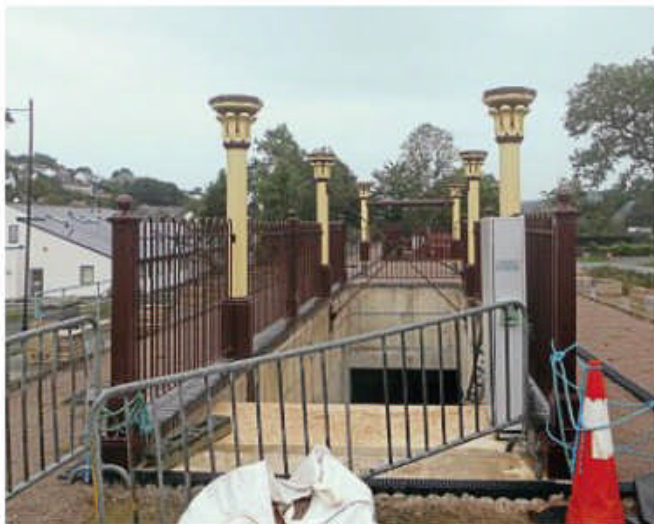
The canopy columns from London's Blackfriars station in position on September 2. ROBIN JONES
