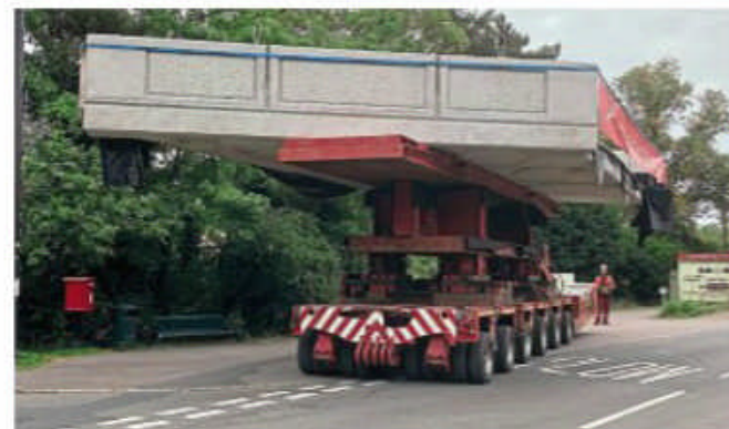
The new deck for Bridge 341 on its way by road from Quorn & Woodhouse station yard. GCR
