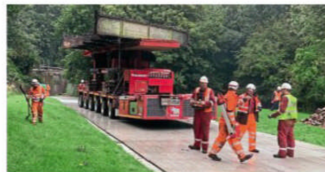
Track mats were laid on the field leading to Bridge 341, to allow the transport carrying the old deck to be brought out on September 2. GCR
