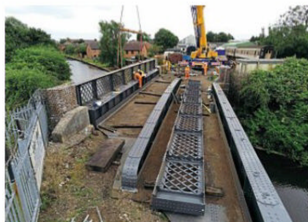
The first of the restored side panels is installed on the bridge. FoGCML
