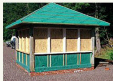
Built off-site as a kit of parts during lockdown, the panels of Invergarry station's replica signal cabin are taking shape. INVERGARRY & FORT AUGUSTUS RAILWAY MUSEUM
