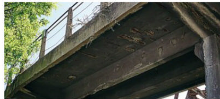
Above: The underside of a section of viaduct awaiting repair with exposed steel reinforcing bars evident. SKLR
