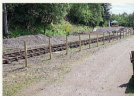
The new fence is seen along the running line at Invergarry, which was erected during lockdown. INVERGARRY & FORT AUGUSTUS RAILWAY MUSEUM
