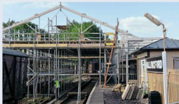
The Maidenhead station canopy being re-erected at Wallingford. DR TONY STEAD
