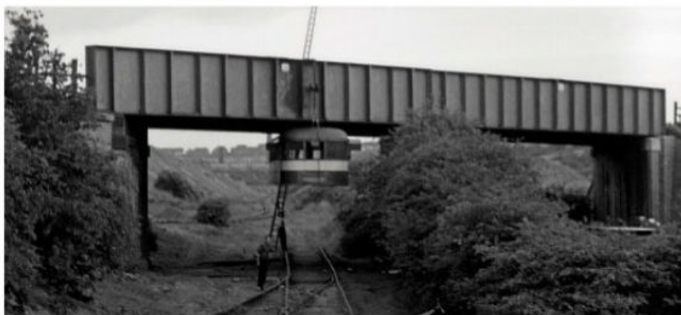
Above: Was this the most unusual way of delivering and reassembling a carriage in history? The top deck of Swansea & Mumbles car No. 2 is craned from the railway overbridge on June 18, 1960, awaiting lowering onto its lower deck and bogies. KEITH TERRY/NATIONAL TRAMWAY MUSEUM, CRICH
