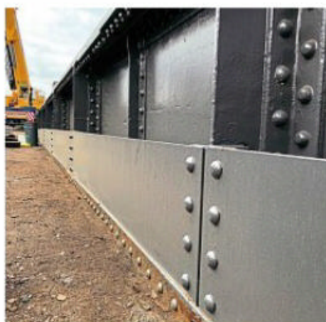
Right: Loughborough's Grand Union Canal bridge side panels being replaced on July 3. The GCR's locomotive sheds can just be seen behind the crane. FoGCML
