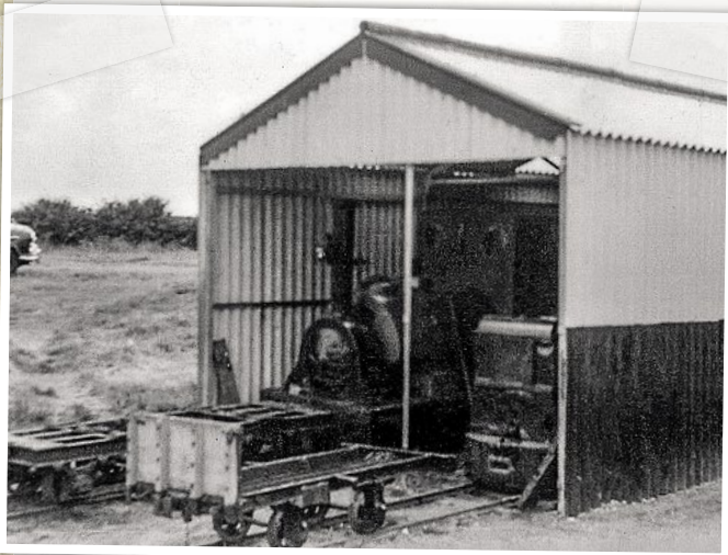
Above: In 1961 the LCLR bought two locomotives from Rugby Portland Cement's works at Southam in Warwickshire: Peckett 0-6-0ST Jurassic No. 1008 of 1903 – the star attraction of today's Skegness LCLR – and Lincoln-built Ruston Hornsby three-cylinder 3hp diesel No. 168437. The diesel proved near-impossible to start and was too slow for passenger services, so it was broken up in 1968. CW UNDERHILL/CCLR/LCLR
