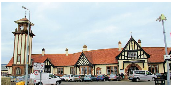
Wemyss Bay station with its clock tower. The flat windows can be seen above the ground floor. HUGH DOUGHERTY
