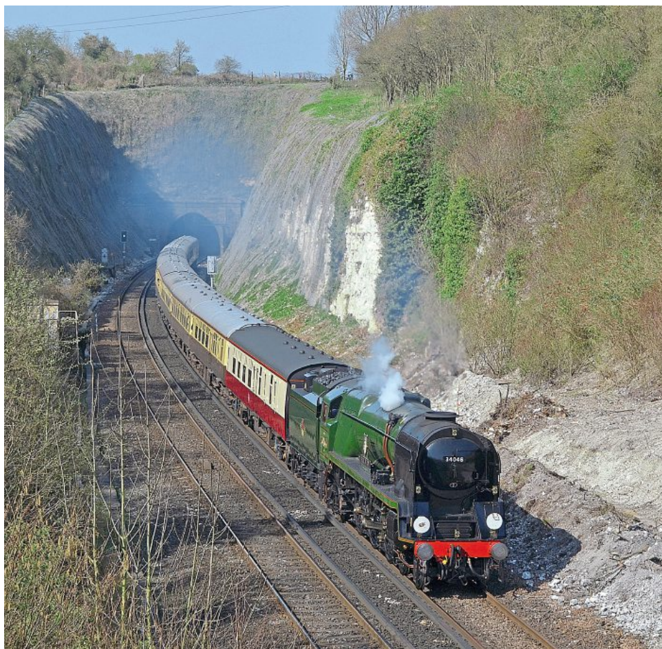
On March 27, 2014, Bulleid West Country light Pacific No. 34046 Braunton has just exited Chelsfield Tunnel and is approaching Knockholt with a 7.04am Solihull-Canterbury West excursion. Newly-completed remedial work on the chalk walls of the cutting shows that land slippage here remains a concern a century after Nesbit's time. DAVID STAINES
