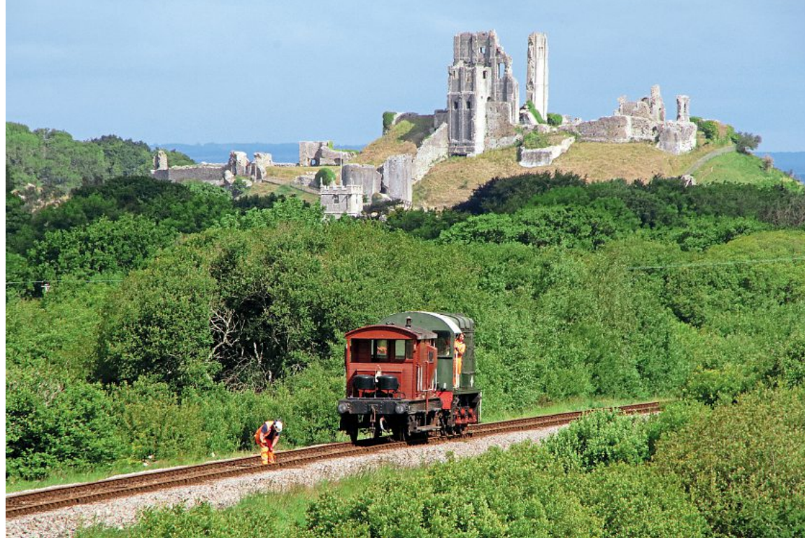
South of Corfe Castle – and with the historic ruins of the medieval castle dominating – the Swanage Railway's permanent way manager Barry Light checks and tightens fishplate bolts during a regular inspection of the heritage line's track on June 5. Hauling the short works train is D3591 – one of the line's two Class 08 shunters – which was built at Crewe in 1958 and a Purbeck resident since 1986. ANDREW PM WRIGHT
