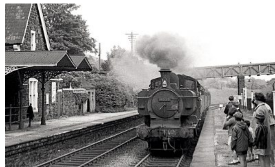
The last eastbound passenger train from Pontypool to Neath enters Pontypool (Clarence Street) on December 30, 1964, again hauled by No. 4639. RH MARROWS
