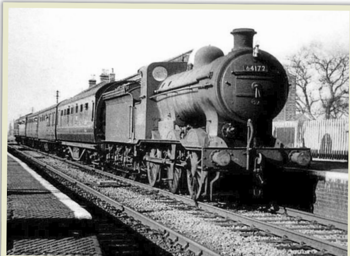
GNR Ivatt 521 class (LNER J6) 0-6-0 No. 64172 is seen heading east through Twenty in the 1950s. Built at Doncaster in 1911, No. 64172 was withdrawn from Boston in March 1960 and scrapped the same month. All of the class had been withdrawn by 1962. HERITAGESOUTHOLLAND.CO.UK
