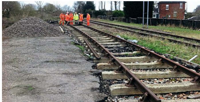
The siding being laid by the Bramley Line Heritage Railway Trust at Waldersea depot, where it hopes to create a visitor centre. BLHRT
