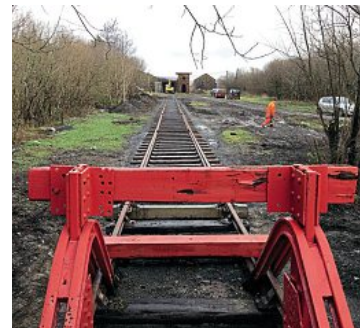
Broad gauge track laid on the original formation. JIM DEEGAN
