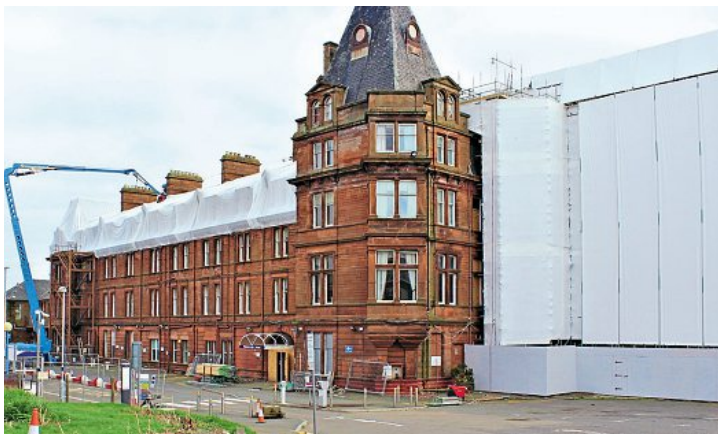
Scaffolded and shrouded, Ayr Station Hotel awaits its fate. HUGH DOUGHERTY
