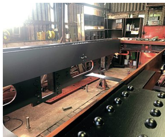
Work has continued on No. 5551's tender frames in South Devon. LEAKY FINDERS/THE LMS-PATRIOT PROJECT
