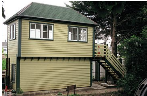
Left: The new Nene Junction signalbox, which is now ready to welcome visitors to Railworld from July 4. This is the rear of the structure looking towards the main lines. BRIAN PEARCE
