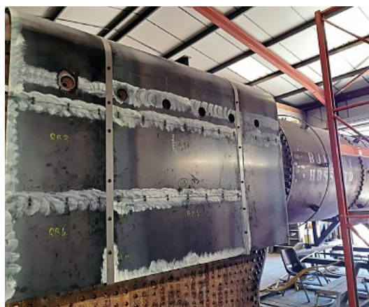
Good progress is being made on fitting cladding to No. 5551's boiler. HBSS/ THE LMS-PATRIOT PROJECT
