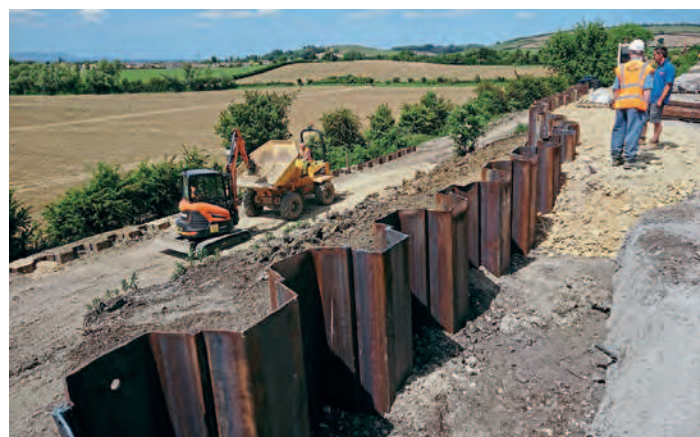
Contractors finishing the repairs to the landslip south of Gotherington station in late May. JONATHAN TAYLOR/G/WRW
