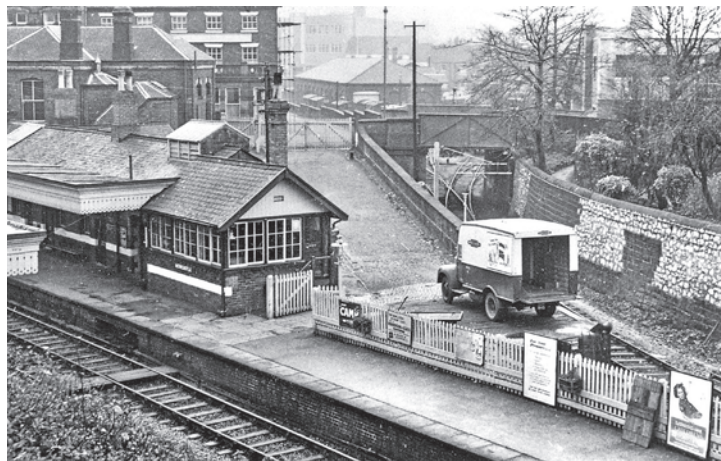
Sign of the times: A British Railways' truck waits in the yard of Newcastle-under-Lyme station in May 1964, two months after it closed. The line on the right led down to the goods yard. Ten totem signs from the Staffordshire station sold for a total of two guineas (£2.10) in a railwayana auction in Stoke-on-Trent on June 6, 1964. BRAMPTON MUSEUM, NEWCASTLE-UNDER-LYME
