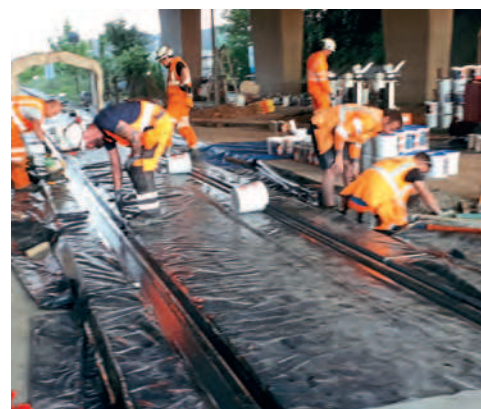
The installation of the new Yaxham Road crossing underway. MNR
