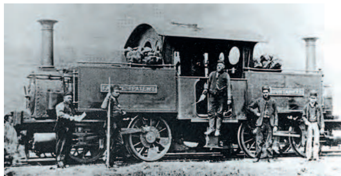
Above: Double Fairlie Mountaineer of 1869 at Burry Port in the 1890s. The Burry Port & Gwendraeth Valley Railway was the only standard gauge line in the UK to regularly use double Fairlies. GRS
