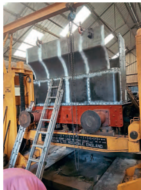
Latest progress being made on the bunker of Didcot flagship No. 1466. WESTERN STEAM ENGINEERING
