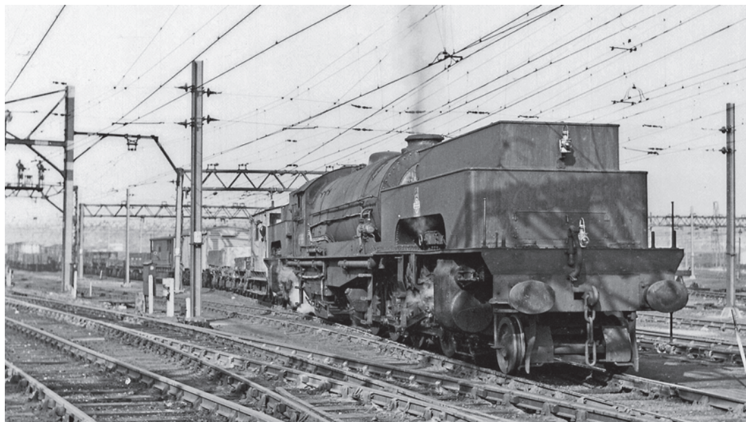
Unique LNER U1 class 2-8-0+0-8-2 No. 69999 heads a freight train out of Dewsnap Sidings near Guide Bridge on the electrified Manchester to Sheffield route on October 11, 1953. The Beyer-Garratt was photographed by Brian Green during his time based in the area. BKB GREEN
