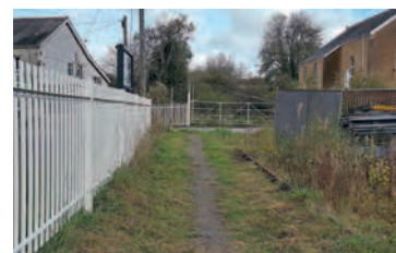
The refurbished level crossing gates and new station fencing at Pontyates. GRS
