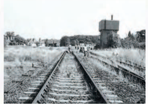
Clearing weeds from the track in 1959. BLUEBELL RAILWAY ARCHIVE
