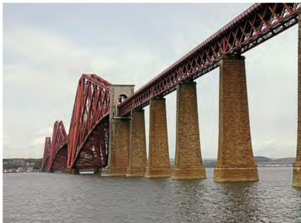
Looking along to the south cantilever which will be topped by the viewing platform. It will be accessed by a walkway and stairs. HUGH DOUGHERTY
