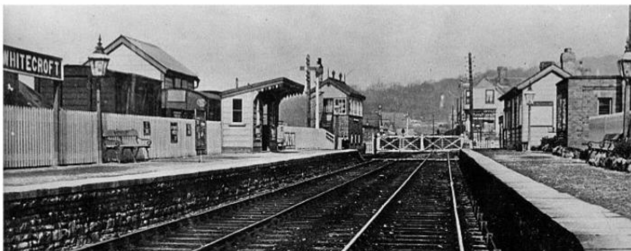
Whitecroft station in its heyday, complete with a passing loop that is set to be restored.
