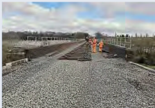
Track being re-laid on Falling Sands viaduct a mile west of Kidderminster on March 21. BRENT CLEETON/SVR
