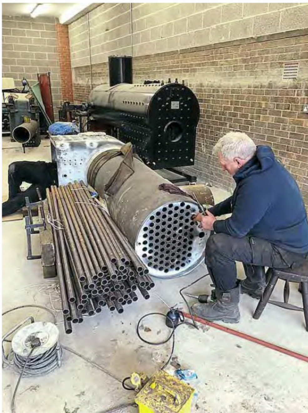
Tubes being fitted in the replica of 1863-built Mountaineer's boiler. NBRES
