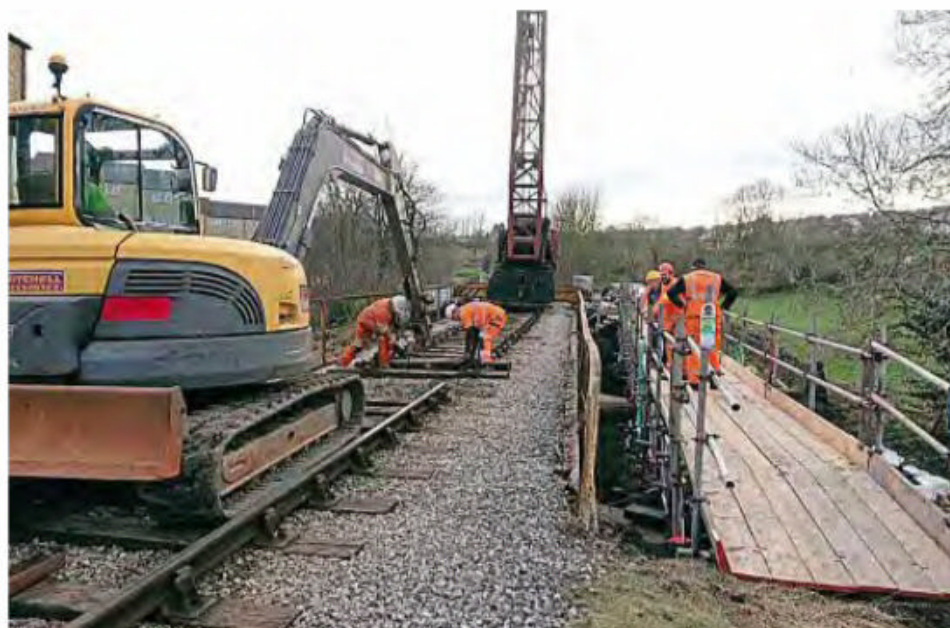
Above: Track being lifted at the start of the bridge replacement operation. KWVR
