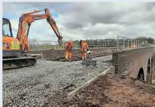
Track being re-laid on Falling Sands viaduct a mile west of Kidderminster on March 21. BRENT CLEETON/SVR
