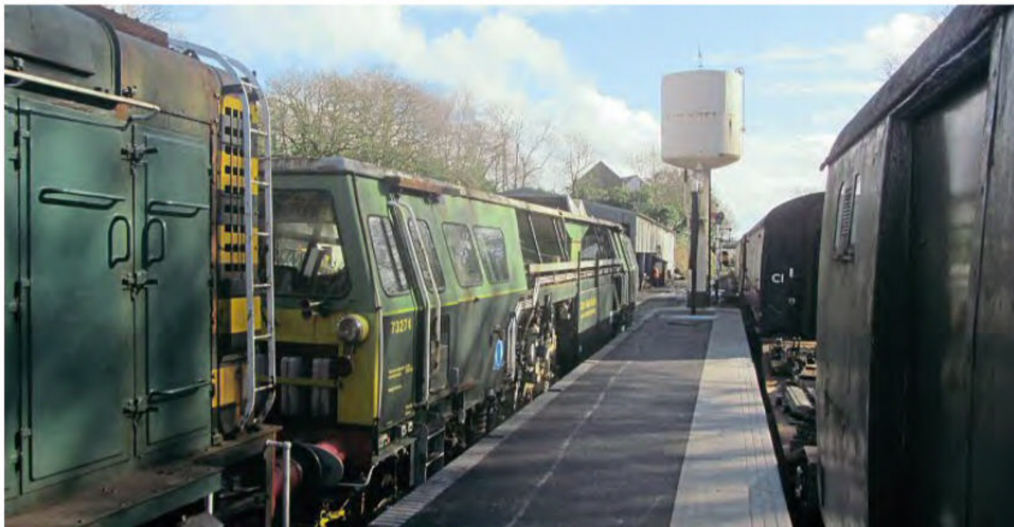
March 11 sees platform 2 almost complete, and awaiting a fence on the left-hand edge. Tarmac has just been laid. In the shed road stands the South Devon Railway's tamper, and in the platform itself the permanent way train. JIMMY JAMES
