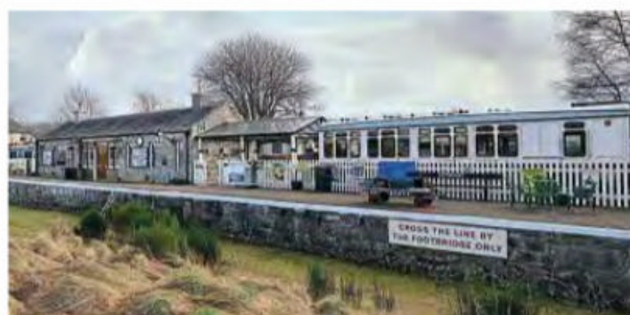
The platform view shows how well the restoration of Cromdale station has been carried out. GALBRAITH
