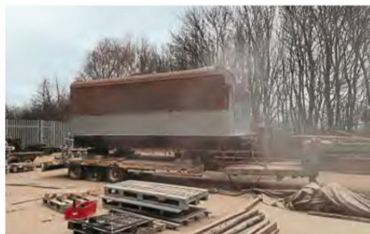
The P2 tender tank being gritblasted at MIS North East at Peterlee on March. MIS was North View Engineering Solutions' subcontractor for this task.
