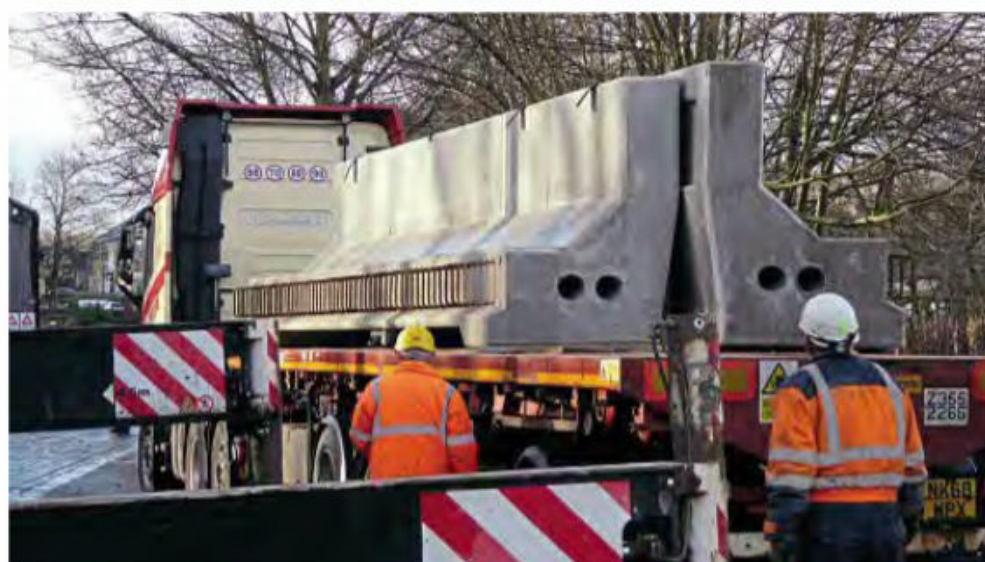
Above: The new beams for Bridge 11 moved into place. KWVR
