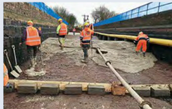
Concrete pumping and placement underway earlier. NICK YARWOOD/SVR
