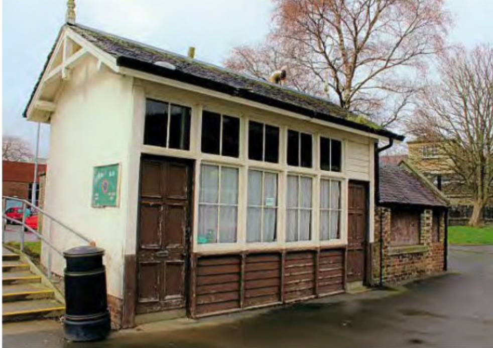
The weighbridge hut which will house the railway museum. HUGH DOUGHERTY
