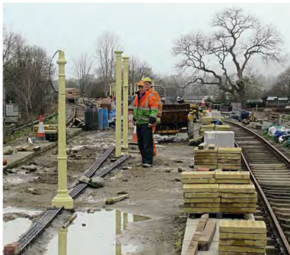
The platform with lamp posts and columns for the Corwen board in situ and drainage channels as laid out with tactile pavers stacked for fitting. GEORGE JONES
