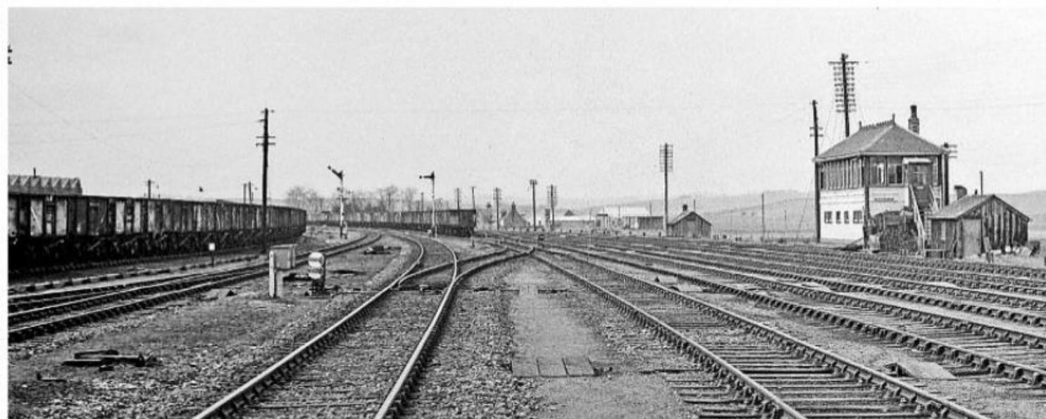
Hopes for survival: A panoramic view at Inverurie station in 1970 with the signalbox on the right, while on the far left the roof of the former Great North of Scotland Railway works that had closed the year before is just visible. The signalbox itself closed last year and could be saved from demolition if current talks between Network Rail and a rail heritage group are successful. TRANSPORT TREASURY/NORRIS FORREST
