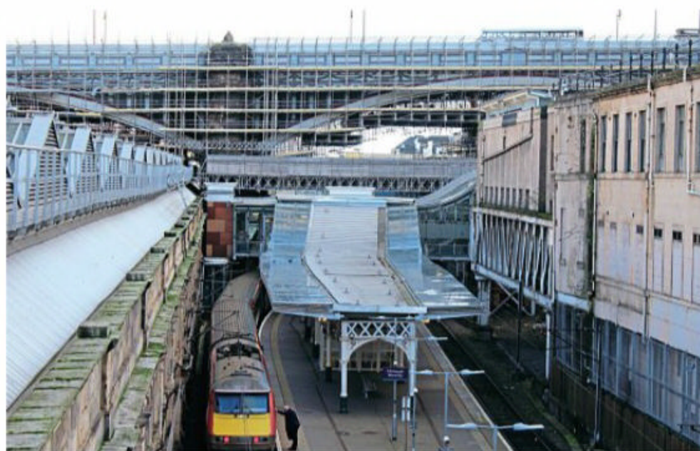
Looking towards scaffolded North Bridge above one of the remaining LNER Class 91-hauled trains in service on January 15. HUGH DOUGHERTY
