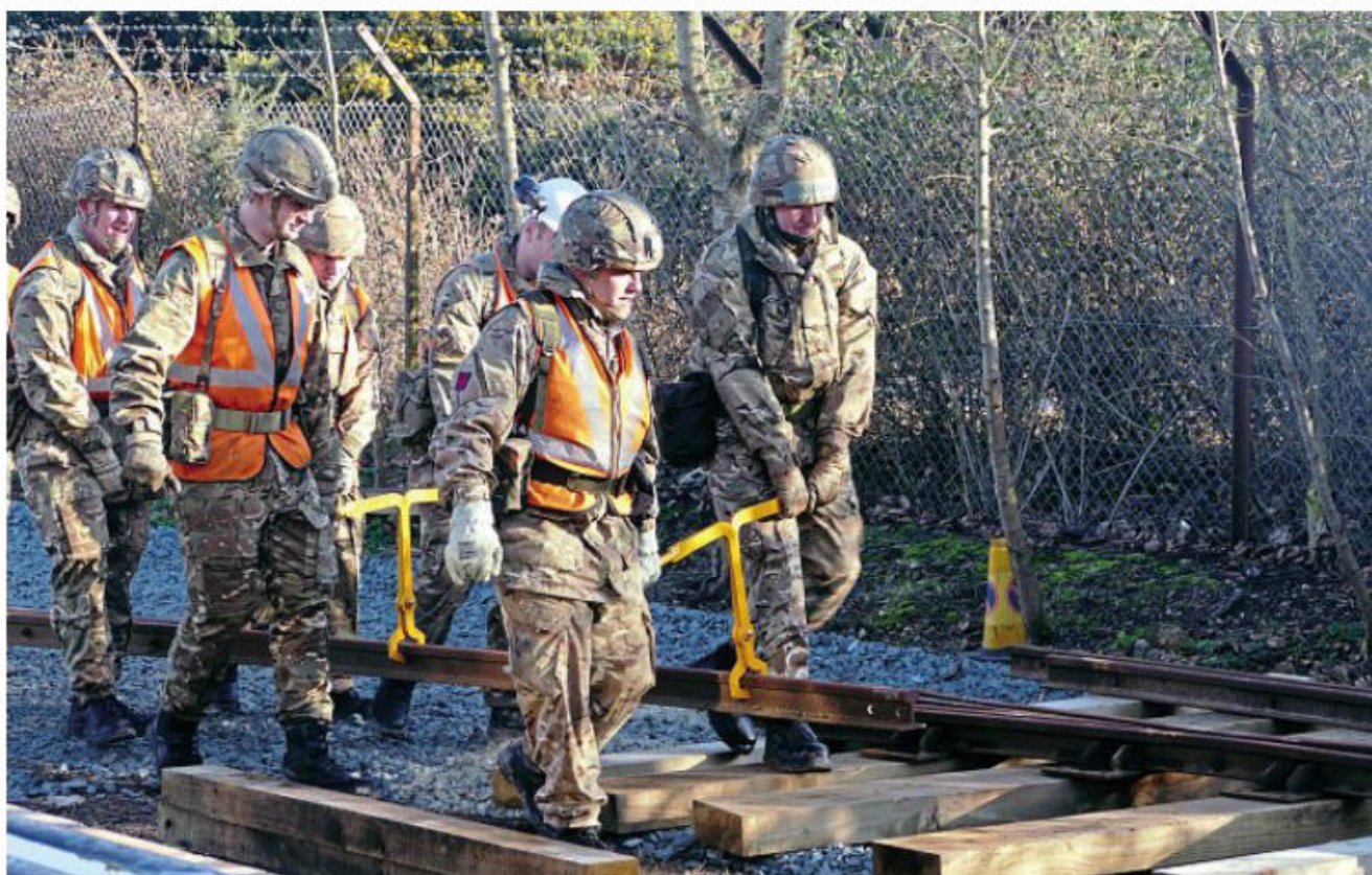
The project received a welcome boost on January 18&19 thanks to the efforts of the 507 Specialist Team Royal Engineers, the army reserve unit that specialises in the repair and construction of railway infrastructure. The 26-strong team descended on the Steamworks site in Blyth Road, Southwold, to lay the first Southwold Railway metals for passenger use in 91 years. SRT
