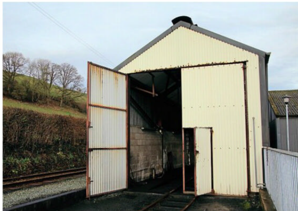
The shed doors – note the pedestrian opening in the right-hand door.
