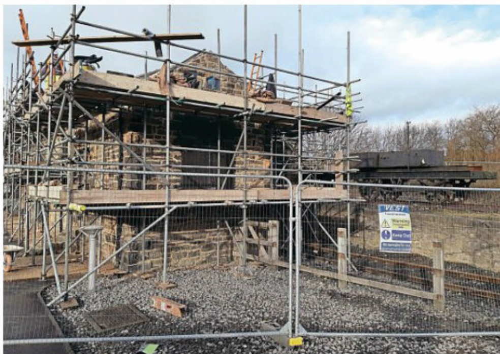
Vital repairs to Grade II listed buildings underway on the Locomotion site at Shildon on January 23. NRM
