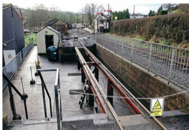
Two pits are located a short distance in front of the shed – one for inspections, the other for ash. The signalbox, workshop and station buildings can be seen in the distance.
