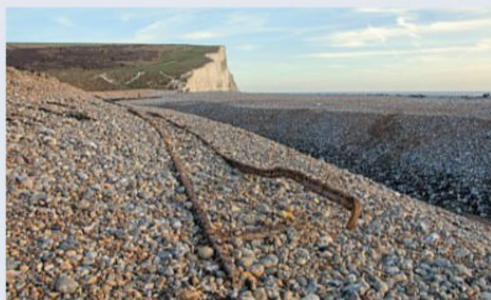
The exposed section of rusting track at Cuckmere Haven, last used 56 years ago, with the Seven Sisters in the distance. ANDREW DIACK
