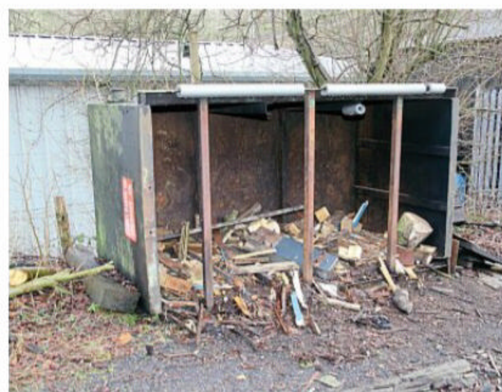
A close-up of the timber store.
