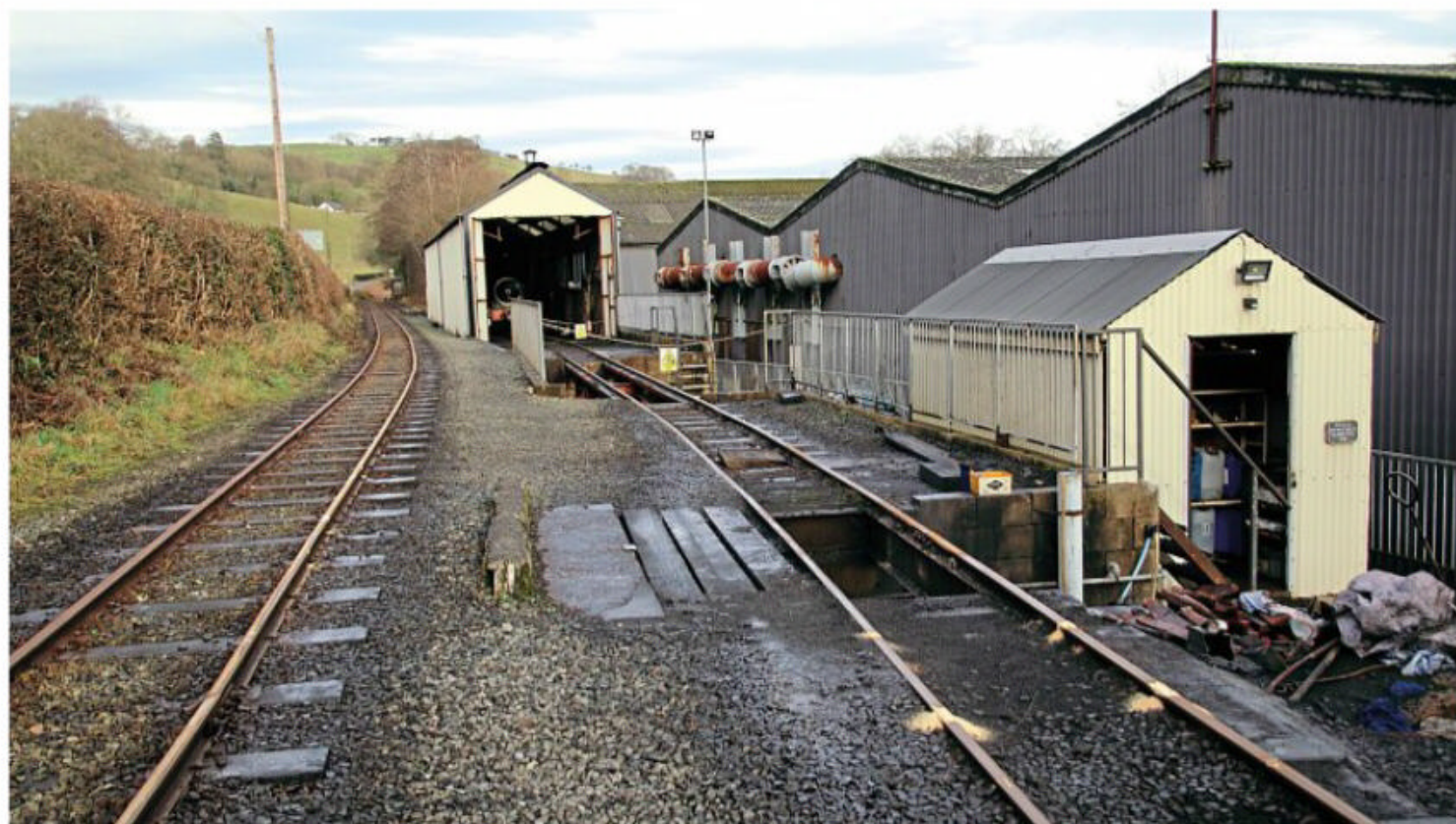
An overview of the shed and pits – the ash pit being in the foreground. The hut on the right serves as a store.
