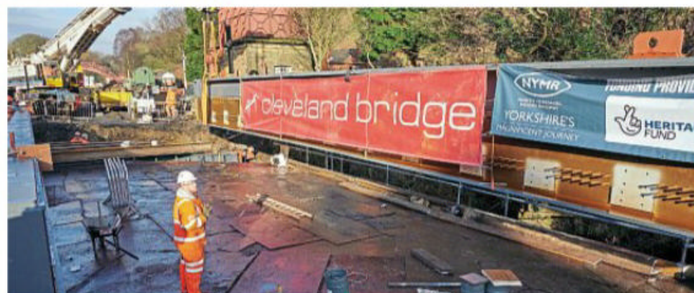
Cleveland Bridge UK engineers are seen undertaking the installation of Bridge 27 on the North Yorkshire Moors Railway.
